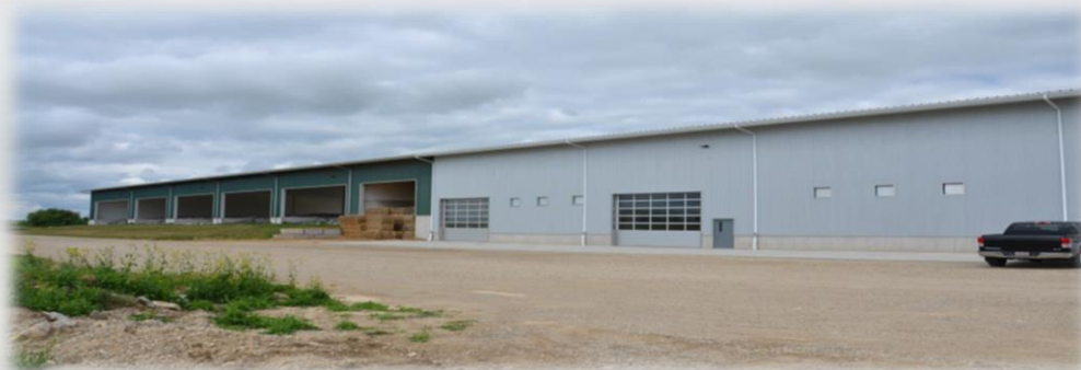
Feed chute delivery exit south side of the Elora Feed Centre.
