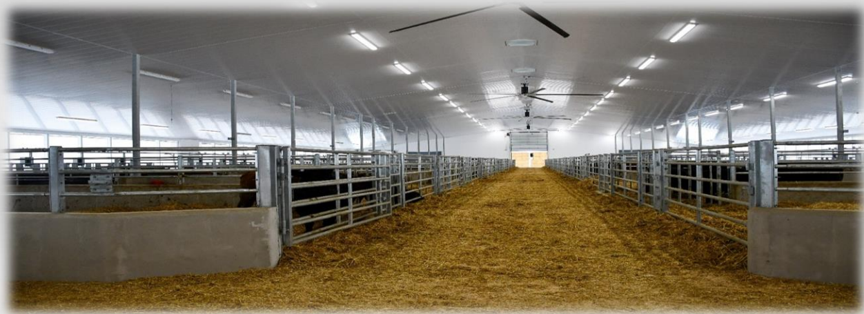
Interior main corridor for new cow/calf barn.
