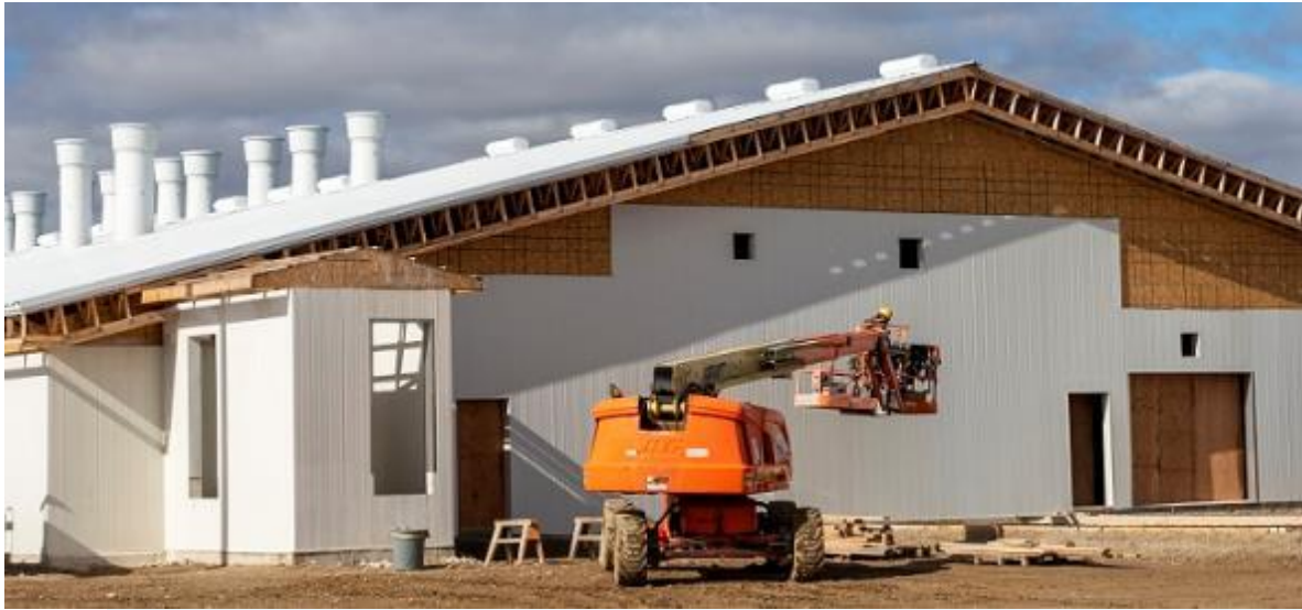
Construction in progress at the Ontario Swine Research Centre in Elora. (Image source: OMAFRA)
