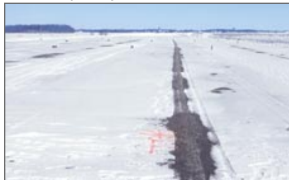
Side-discharge spreader placing salt at centreline
