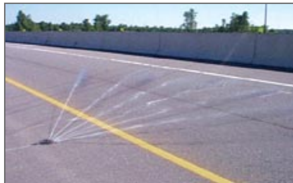
FAST System on Bridge Deck
