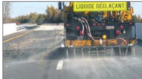
Two-lane Direct Liquid Application by tanker truck
