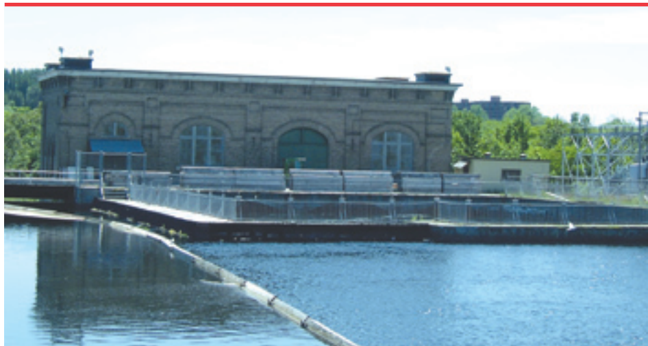
Peterborough Hydro's London Street Generating Station
