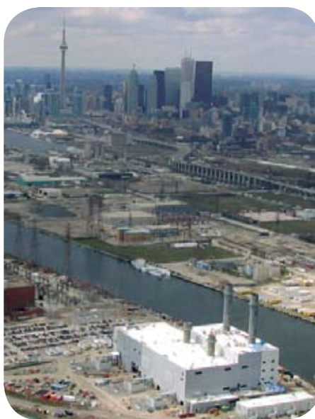
Courtesy Portlands Energy Centre
