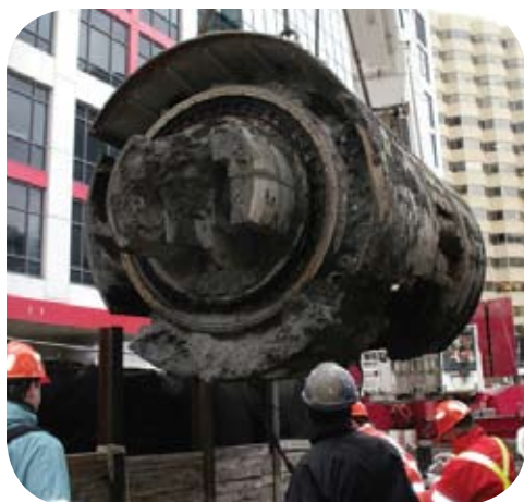
Crews remove the boring machine from its exit point at Hydro One's John Street transformer station.
