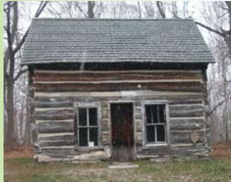
The Foundation is applying to the Ontario Trillium Foundation for the restoration of 3 heritage log cabins at Longwoods. The application is in collaboration with the Upper Thames Military Re-enactment Society. Directors Peter Snow, Anne Smith, and Glenn Stott along with John Lawrence are continuing the research on this project that had been initiated by Sherri Flegel .
