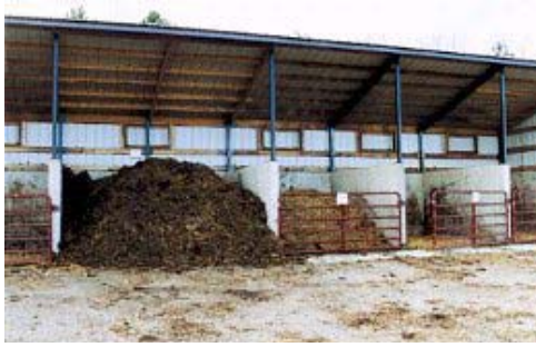
A Bin Composting Unit. (Photo courtesy of Minnesota Department of Agriculture)
