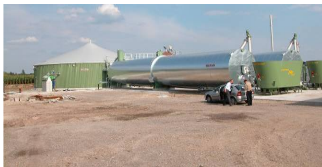
Figure 1. horizontal digester
