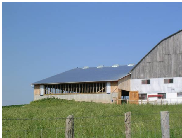
Figure 4: Covered manure storage and livestock yard (separated by concrete walls with swing gates) to eliminate contaminated runoff.*
