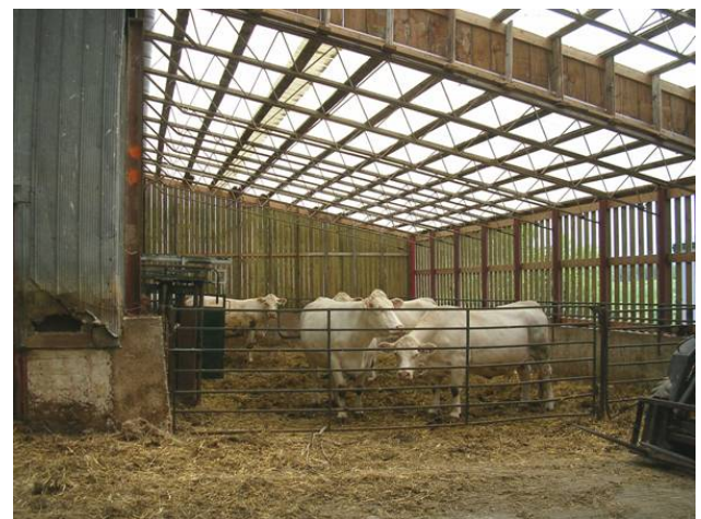
Figure 2: Roofed livestock yard with a poured cement pad and containment walls to eliminate manure runoff and divert precipitation (rain, snow) away from the yard.*
