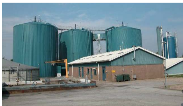
Figure 4: vertical totally mixed digester
