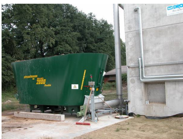
Figure 3: Corn silage being added to a digester
