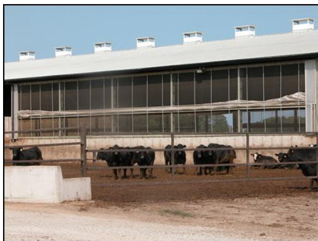
Figure 1. Natural Ventilation Requires Large Wall Openings
