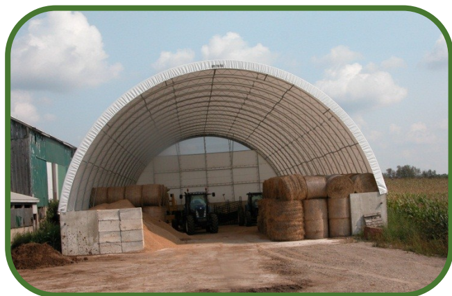
Figure 1. Fabric-covered buildings have multiple uses
