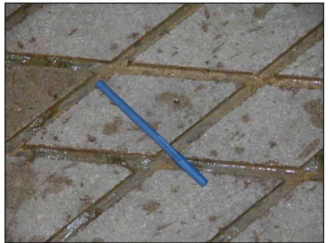
Figure 3. Diamond Grooving for Improving Traction
