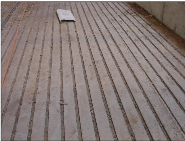
Figure 2. Longitudinal Grooves for Improving Traction
