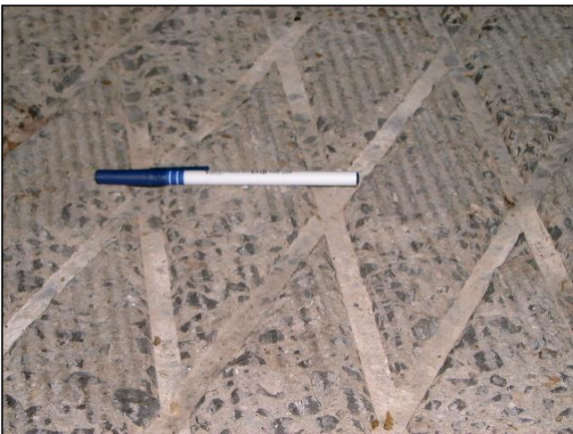
Figure 4. Surface Milling Improves Traction
