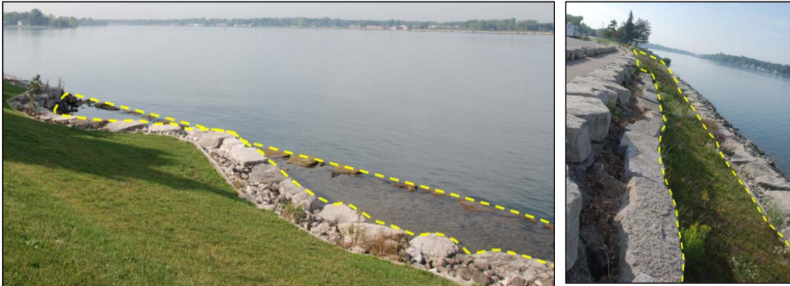
Figure 7.2.1 Guthrie Park Shoreline work. The left image shows an aquatic/wetland habitat pod and the right image a terrestrial habitat pod, outlined in yellow. This project naturalized the shoreline of the shipping channel while maintaining erosion control in the St. Clair River. Similar work will be done at the Courtright shoreline project site.
