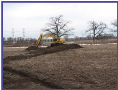
New trail construction at Bowmanville/ Westside Marshes.
