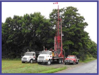
Borehole Drilling Rig.
