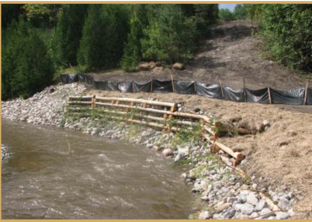
Bioengineering - A live crib wall is used to prevent streambank erosion on a local creek.
