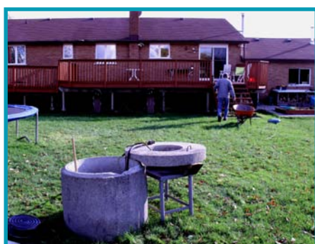
A well prior to receiving an upgrade.
