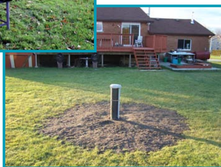
A well after the upgrade.
