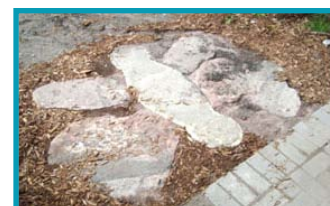
The new butterfly custom stone walkway.
