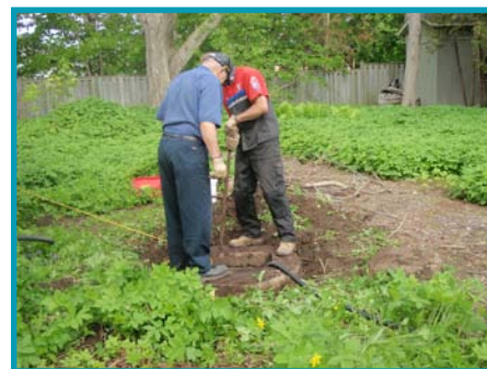
One of the seven inactive wells being decommissioned.
