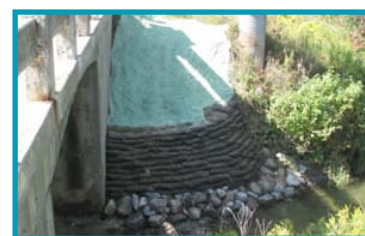
The new Envirolok system installed by CLOCA staff on Taunton Road.
