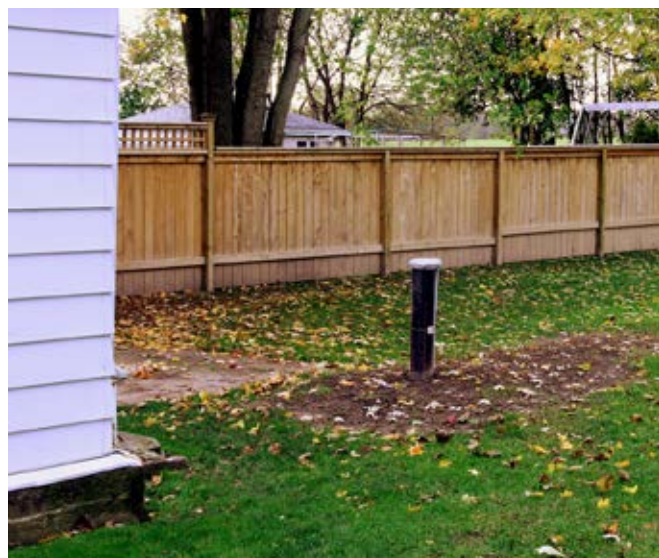
A well after being decommissioned by CLOCA staff.
