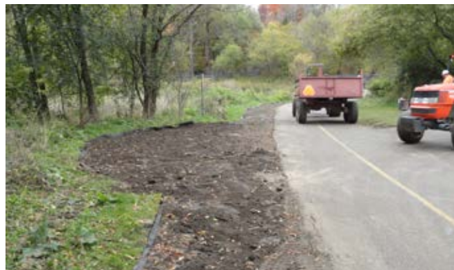
Working along the bike path.
