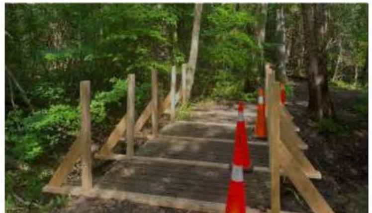
Enniskillen Conservation Area – Under repair
