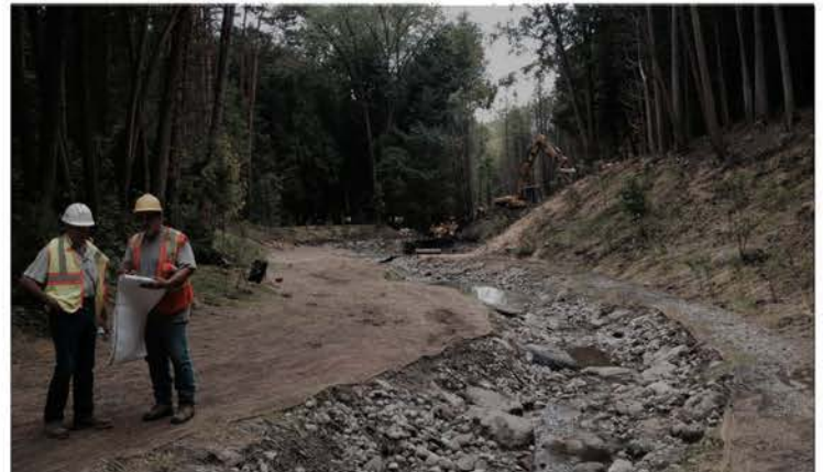
Tributary reinforcement construction
