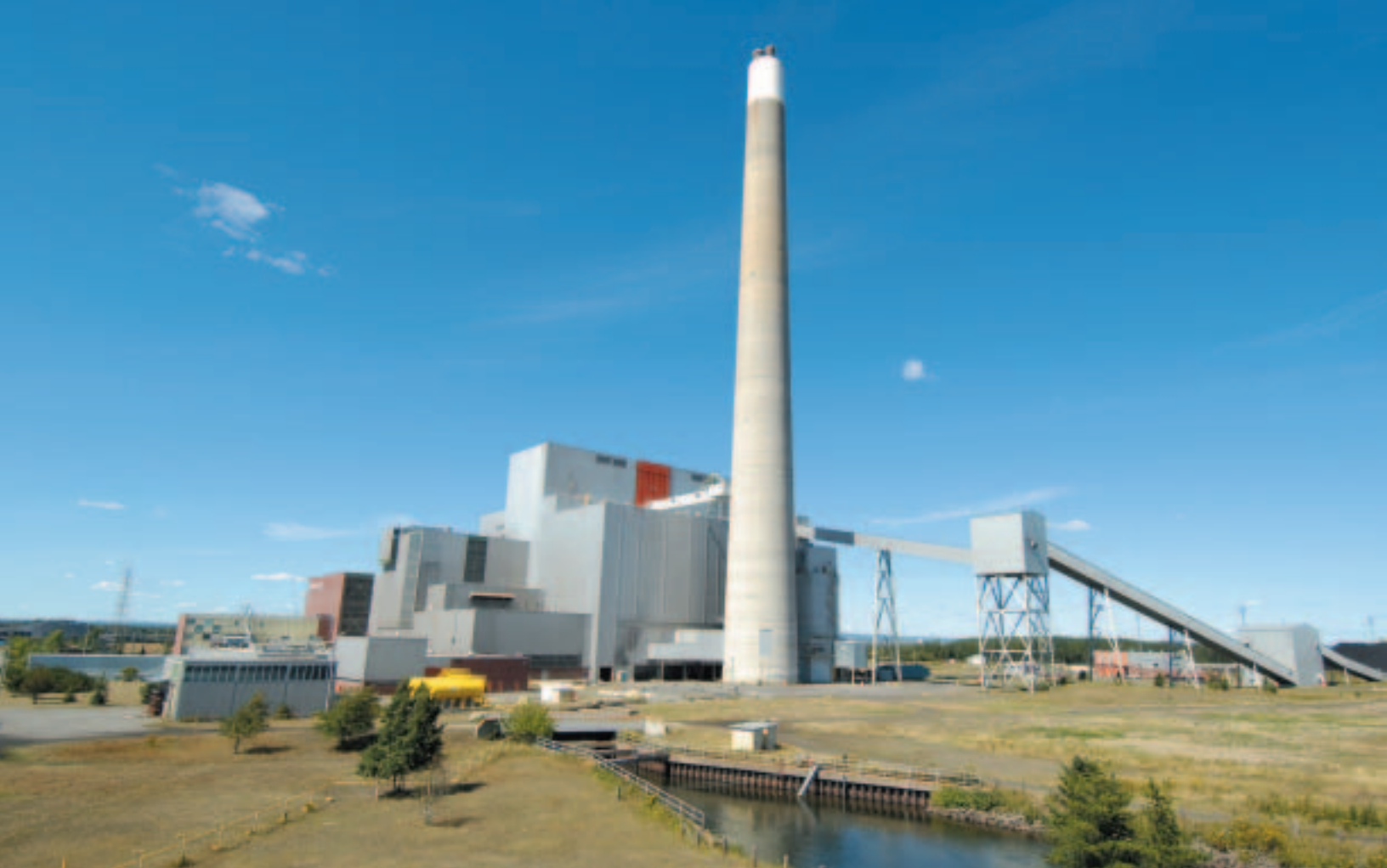
Thunder Bay Generating Station. Photo: Ontario Power Generation
