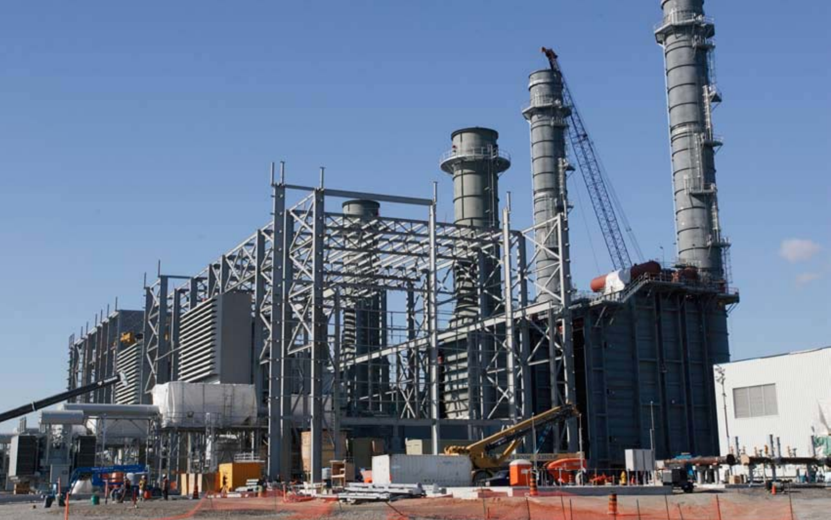
The Portlands Energy Centre in Toronto, currently under construction.
