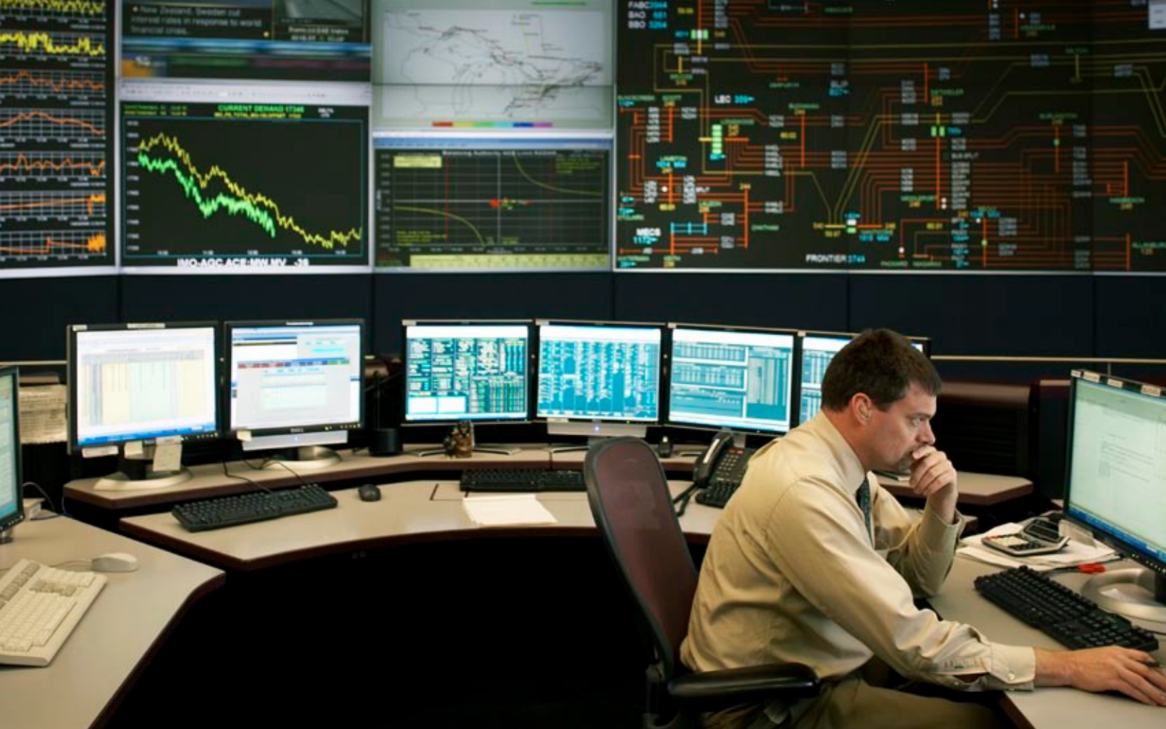
IESO Control Room
