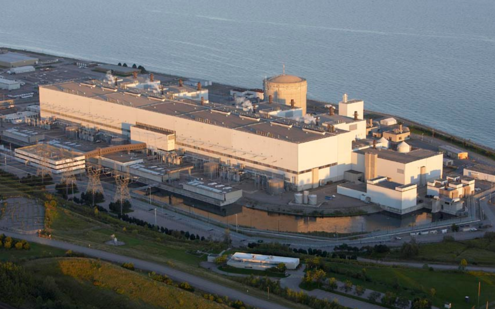
Darlington Generating Station
