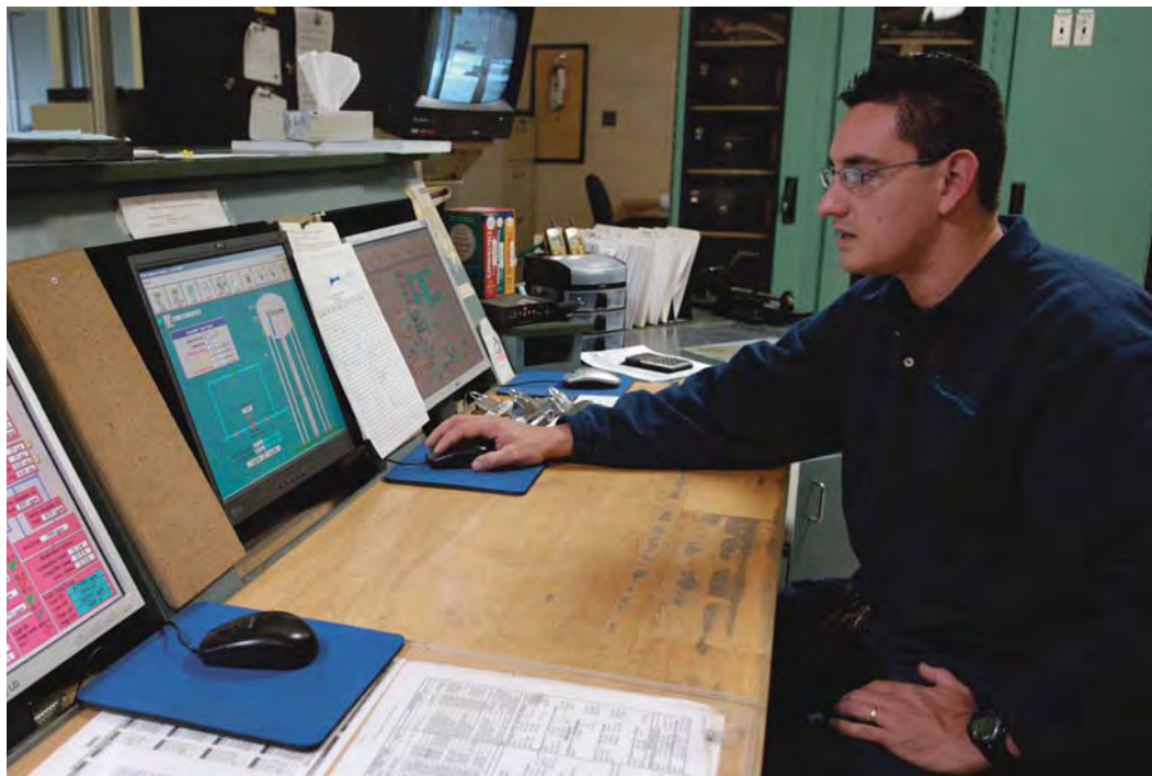
Operator examines the supervisory control data acquisition system (SCADA) screen.
