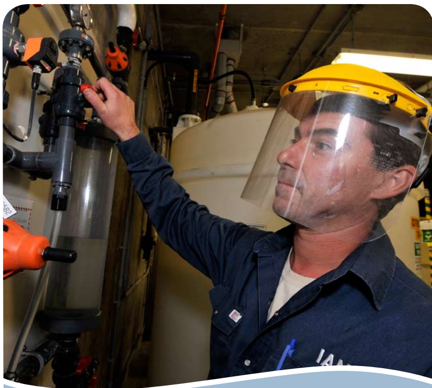
A drinking water plant operator checks equipment.
