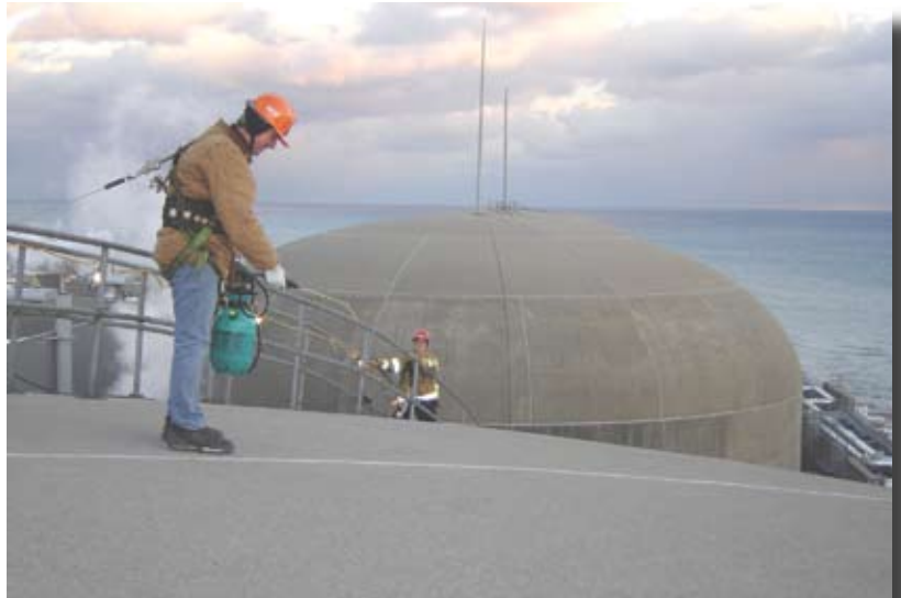
During the recently completed planned maintenance outage for Unit 6, the reactor building was pressurized inside to allow measurement of the integrity of the steel-reinforced concrete building. The employee shown here wearing all appropriate safety equipment, including fall arrest harness, is spraying a specialized solution on the concrete joints looking for leaks. The test results demonstrated the integrity of the building was intact.
