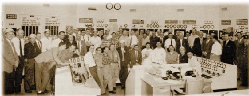
Control room at NPD Generating Station start-up, April 11, 1962
