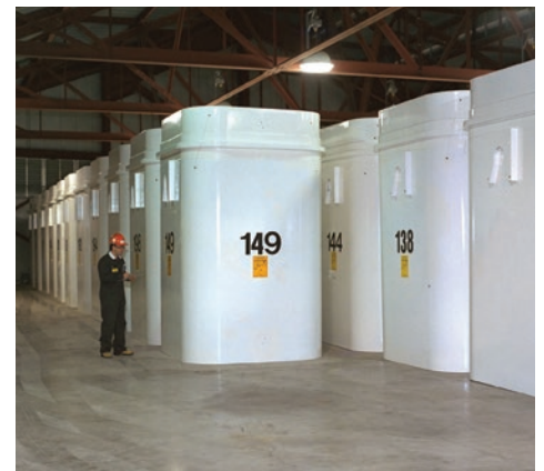
PWMF used nuclear fuel storage canisters
