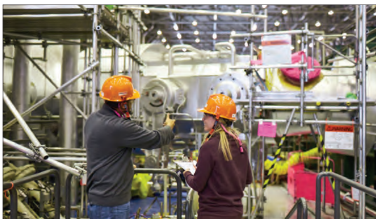
Staff in discussion on the turbine floor of the Darlington Nuclear Generating Station, April 2018.
