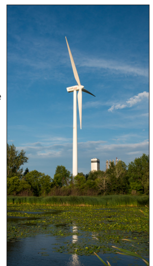
Pickering's Wind Turbine.
