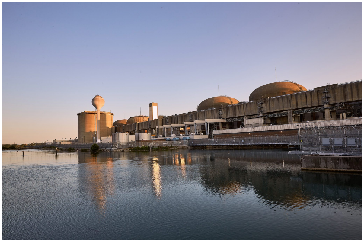
Pickering Nuclear Generating Station
