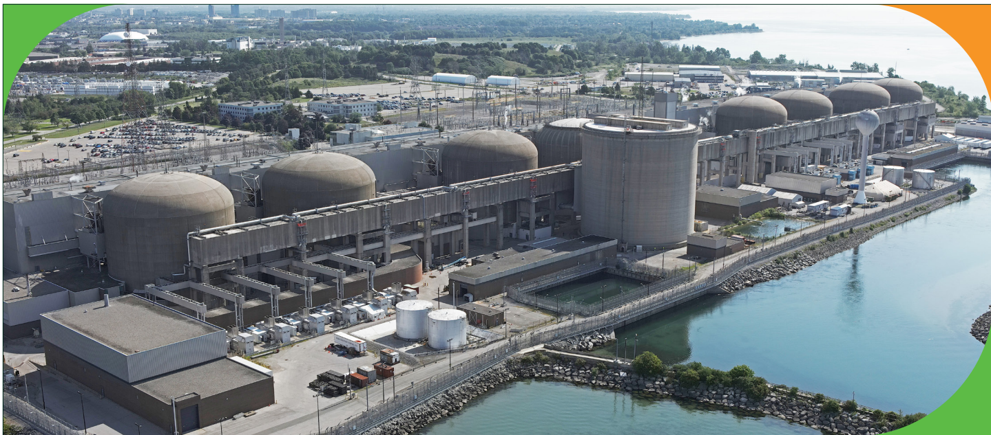
Aerial photo of Pickering Nuclear Generating Station
