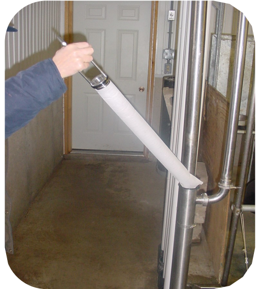
Figure 6: Care should be taken to avoid contamination when installing a new filter.
