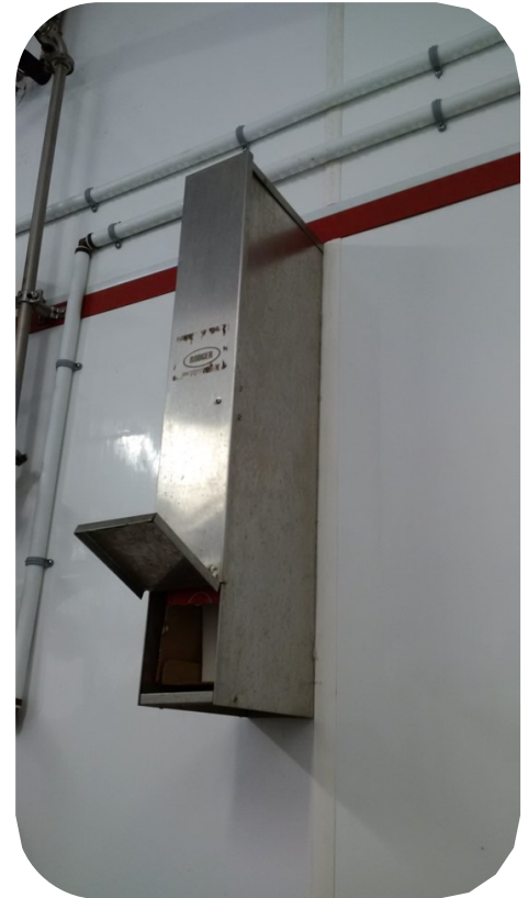
Figure 4: An example of a dust-proof, water-proof filter storage container.
