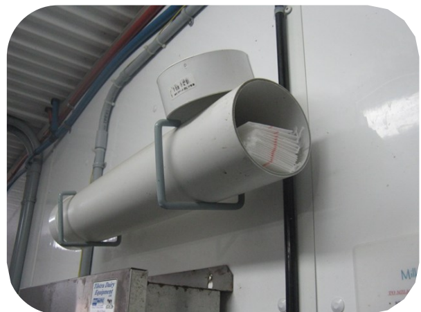
Figure 5: Another example of a dust-proof, water-proof filter storage container.
