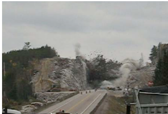
Highway 17 rock removal
