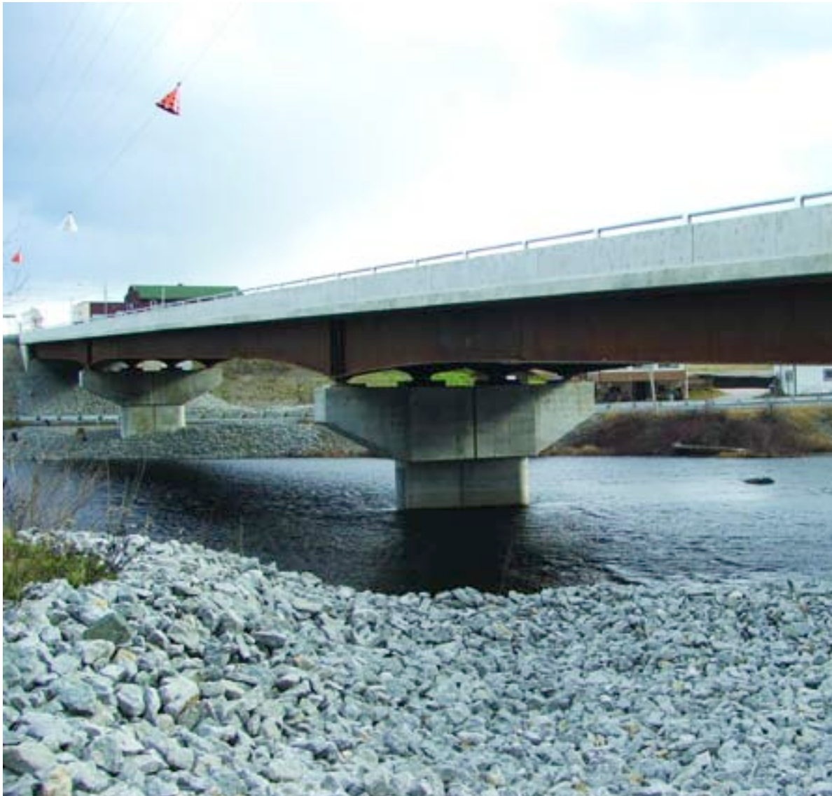
New structure at Matachewan
