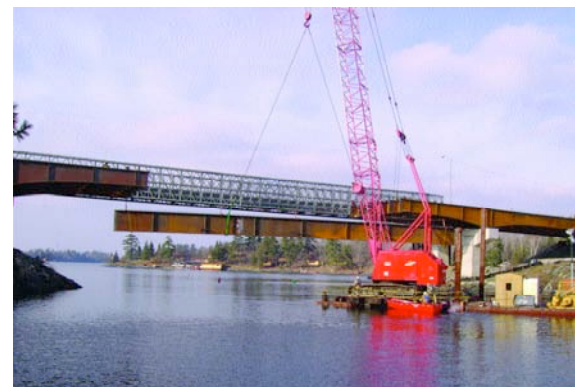
New bridge under construction
