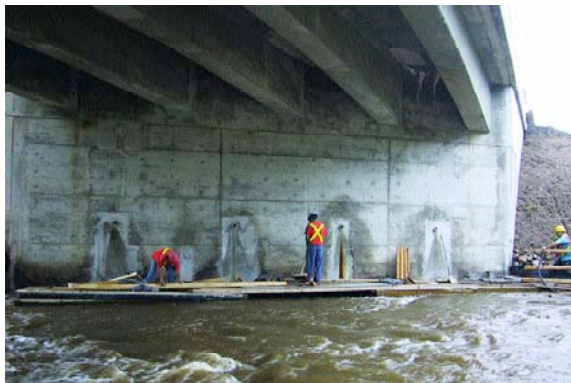
Bridge repairs underway
