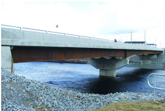
New structure at Matachewan
