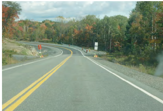
Highway 518 reconstruction complete
