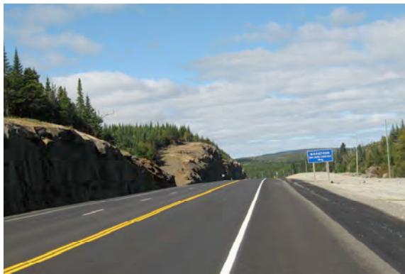
Highway 17 resurfaced with a new passing lane
