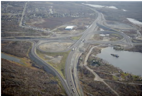
Aerial view of the new interchange on Highway 17
