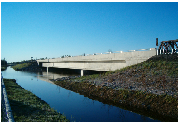
Opasatika River Bridge, Highway 11
