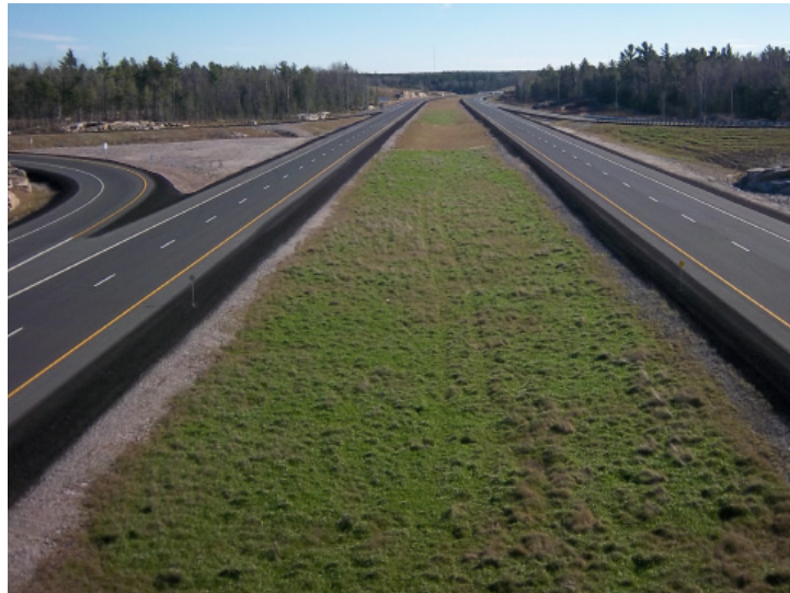
Highway 400/69 after construction
