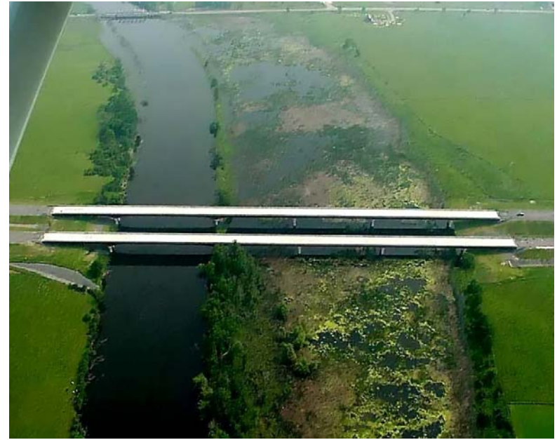
Highway 417 – Mississippi River Bridges, Ottawa
