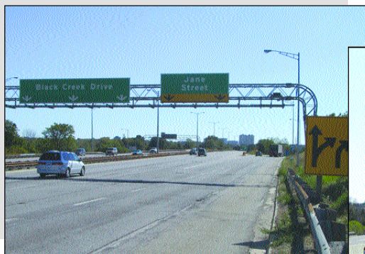
Highway 400 project "before"
