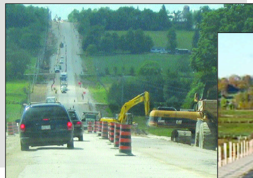
Highway 26 project "during"
