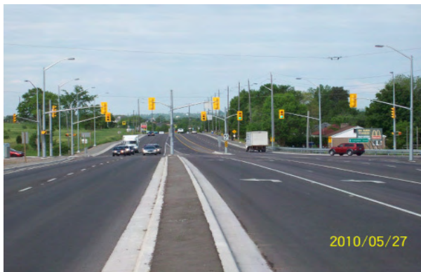
Hwy 7 completed improvements
