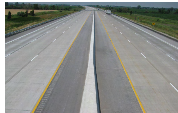
Hwy 401 widening and rehabilitation work completed
