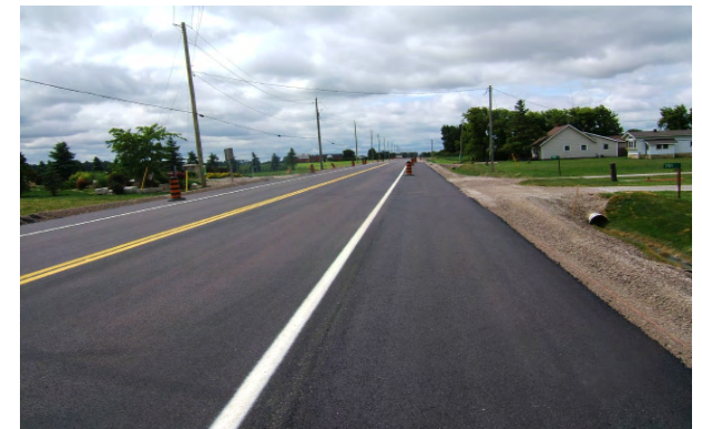
Hwy 77 rehabilitation improvements completed
