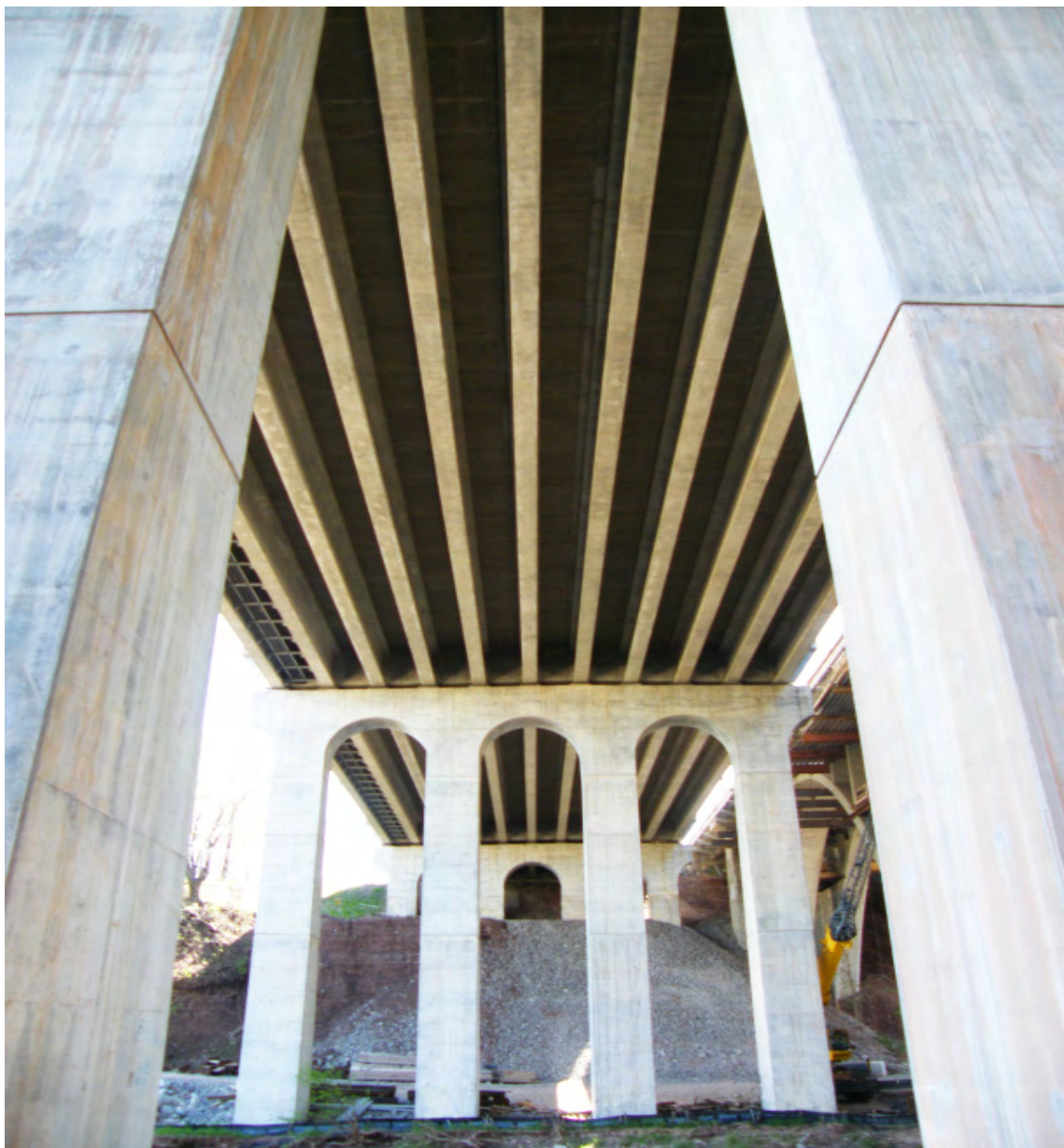
QEW Bridge Rehabilitation
