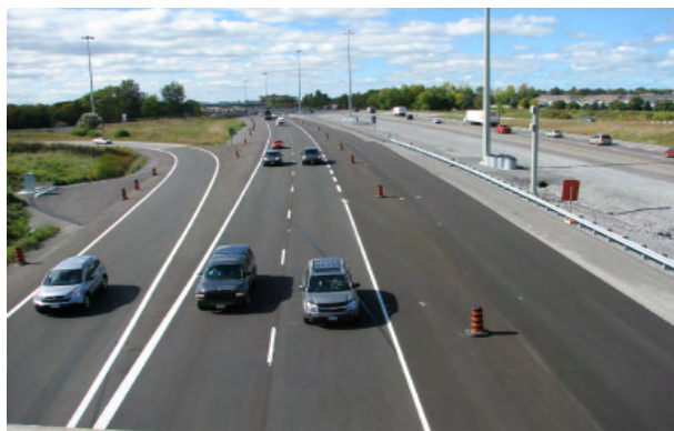
Hwy 417 widening underway
