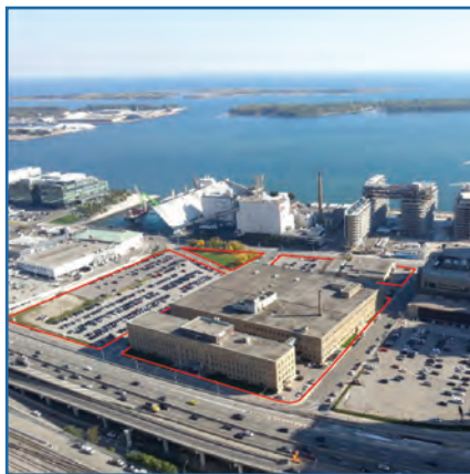
LCBO - Head office Redevelopment
