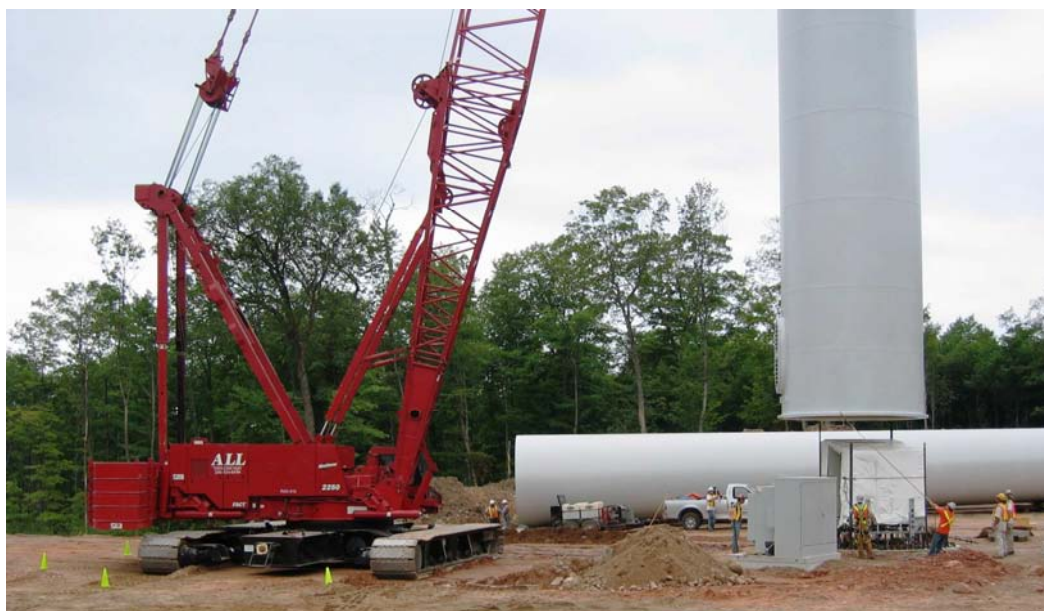
Installing the base section of the tower structure at the Prince Wind Farm. This section weighs 51 tonnes and is required to thread through 200 anchor bolts that have already been cast in the 530-tonne concrete foundation.
