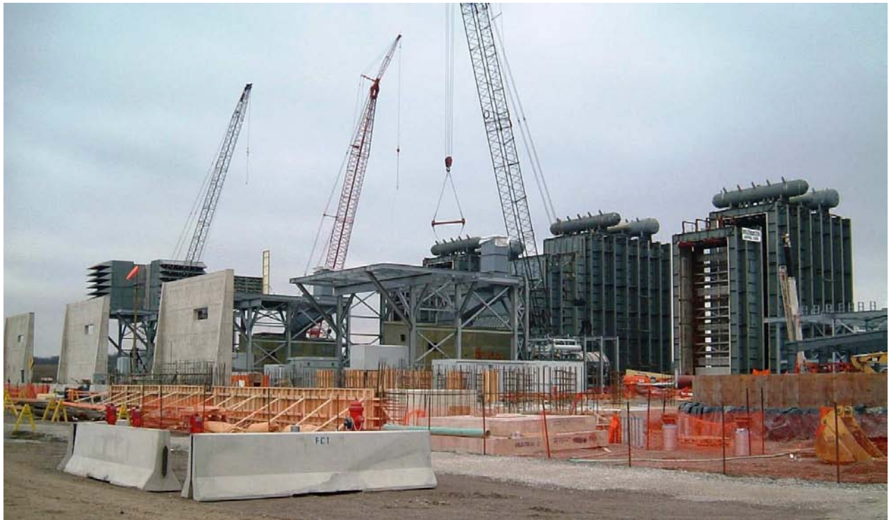
Three heat recovery steam generators are being assembled at GEC.
