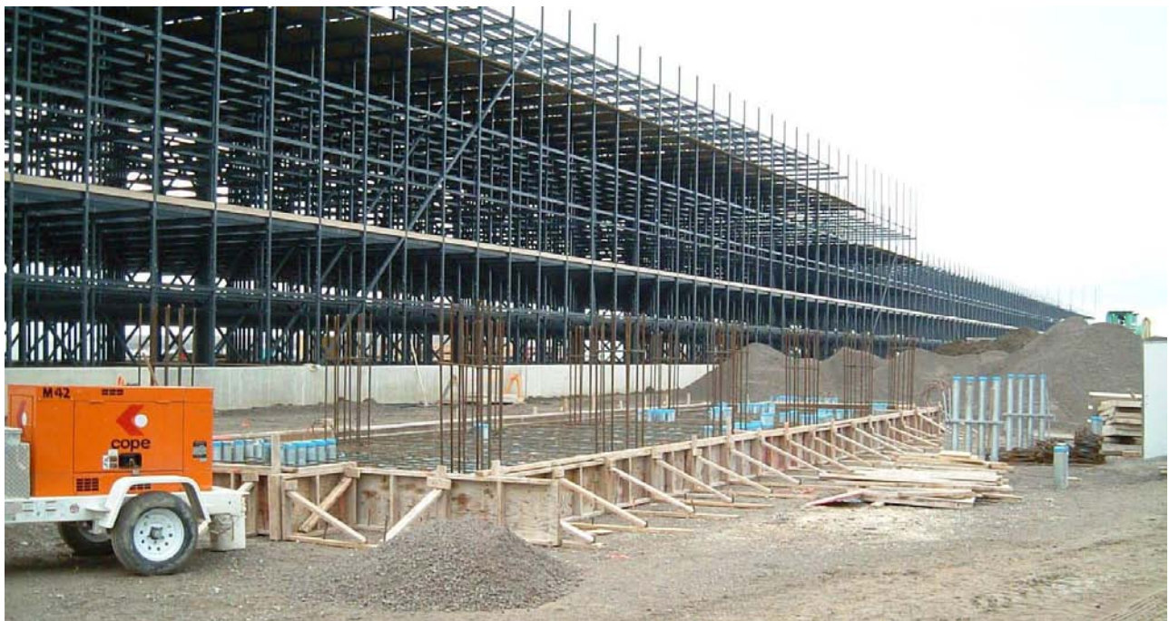
Support for a cooling tower is being assembled at GEC.
