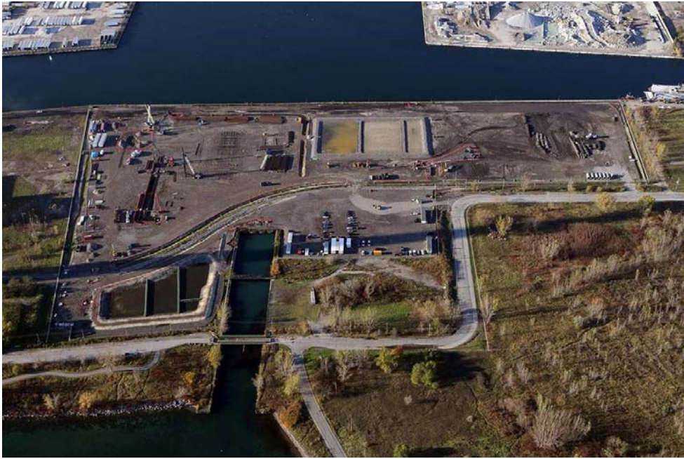
An aerial view of the 538 MW Portlands Energy Centre (PEC), taken in October 2006. This will provide 250 MW of simple cycle operation from this two-on-one natural gas-fired facility by summer 2008, and commercial operation in combined cycle operation is scheduled for summer 2009.
