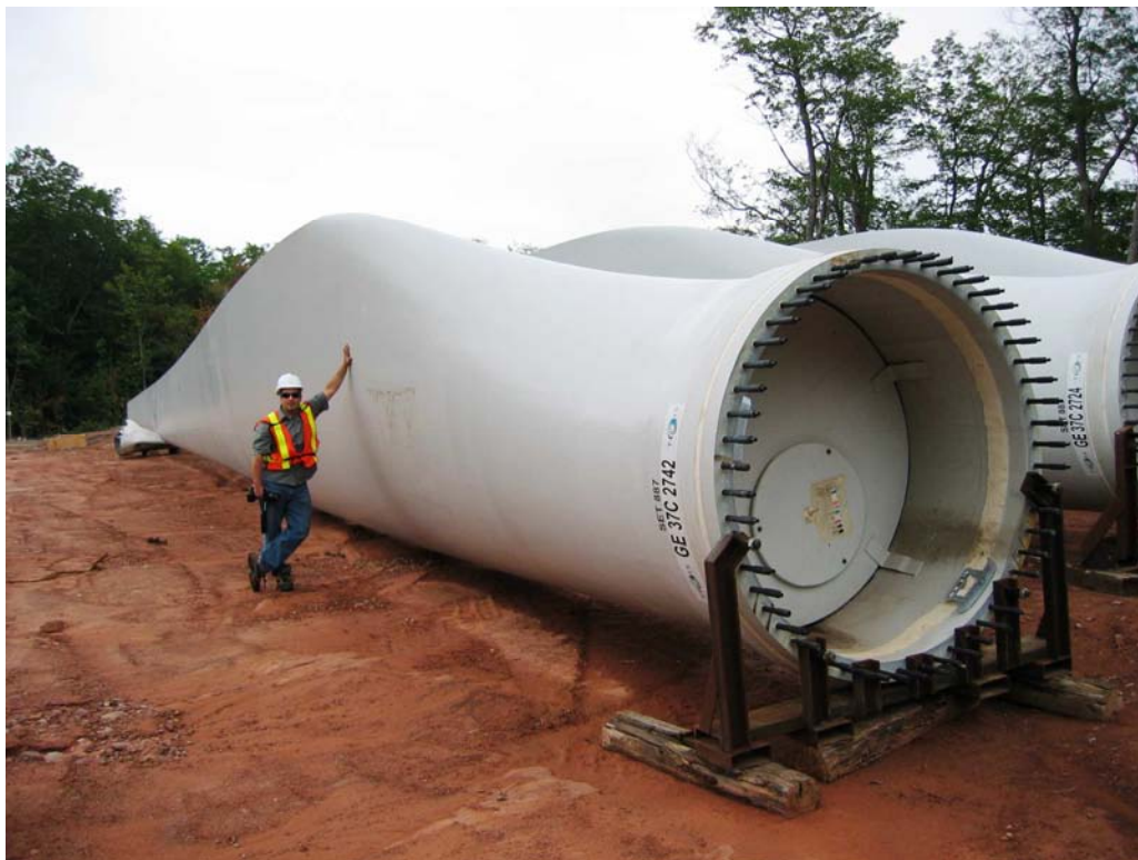
One of the many blades ready for installation at the Prince Wind Farm. Each blade weighs seven tonnes.
