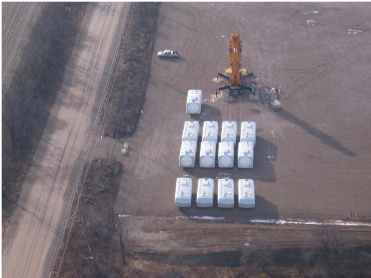
The Melancthon II GE 1.5 model SLE turbine nacelles are being delivered to storage. Each nacelle weighs 56 tonnes.
