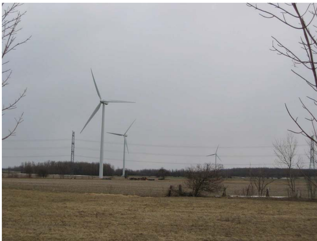
The 40 MW Kingsbridge I Wind Farm developed by EPCOR in Goderich. The project utilized 22 Vestas V80 wind turbines and was placed in commercial operation in March 2006. EPCOR has recently issued a news release notifying its stakeholders that they are re-examining the 160 MW Phase II because of permitting delays.
