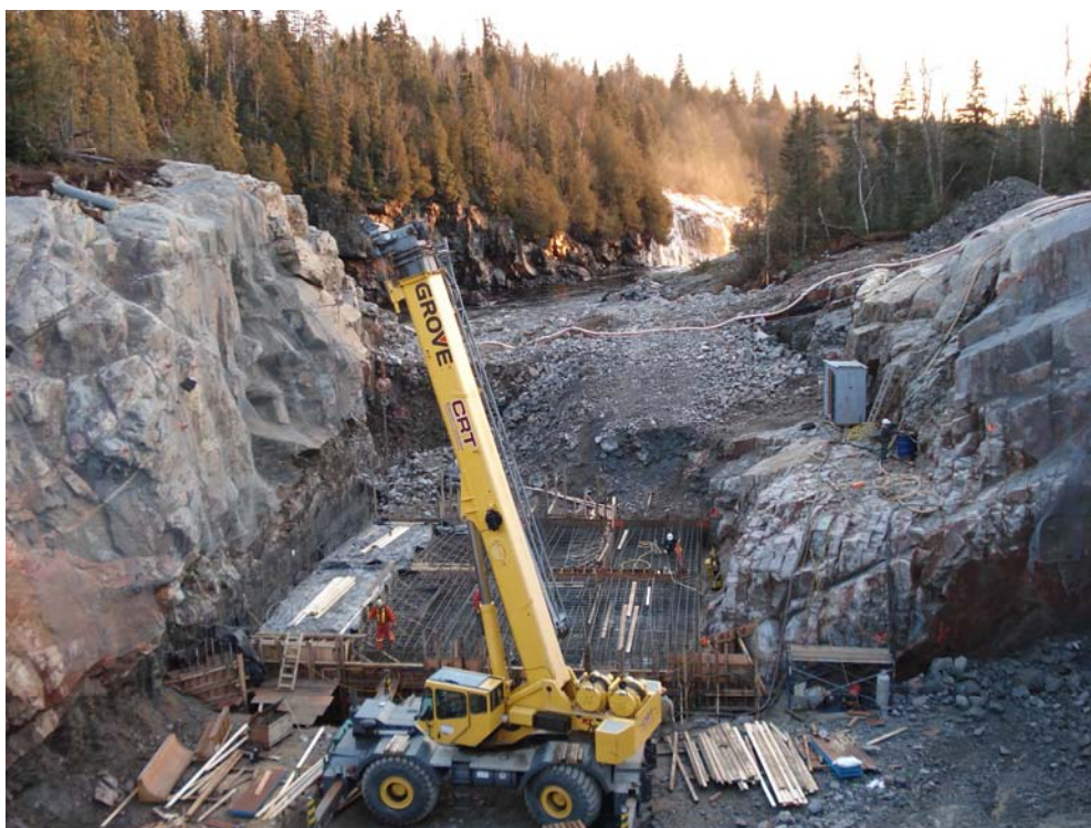
Concreting the base slab of sluice structure at Umbata Falls. The project is scheduled for commercial operation by summer 2008.
