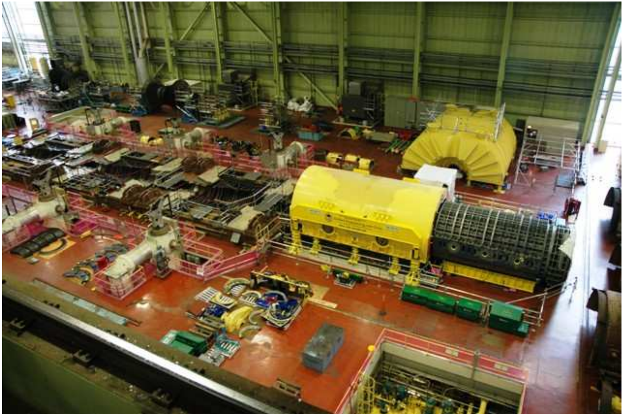
Work in progress on turbine generators at Units 1 and 2
