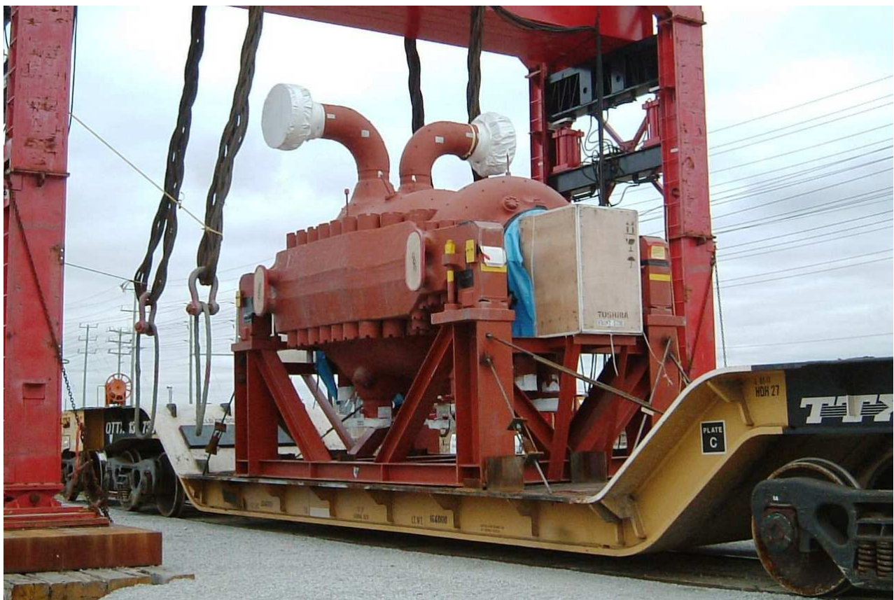
Steam turbine components are delivered to the GEC site.
