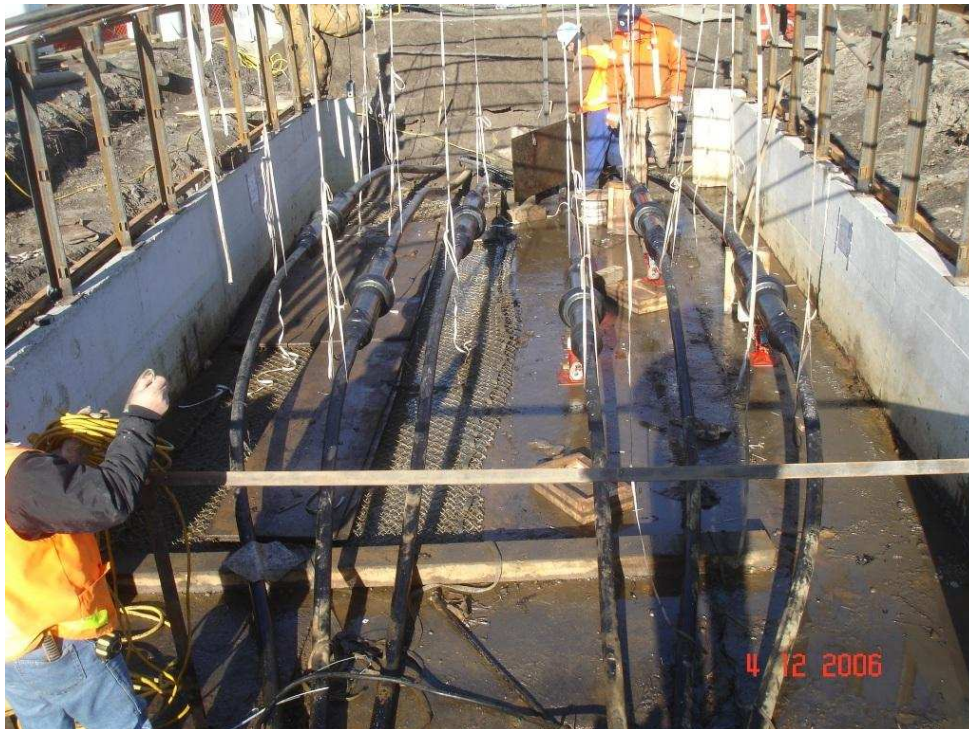
Prior to building PEC, two circuits of existing 115kV underground cables need to be diverted under a tight 43-day outage schedule. In December 2006, joints for the diversion were successfully completed.
