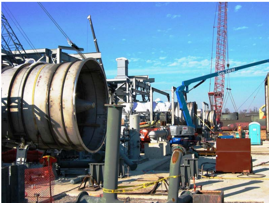
All of the three combustion turbines have already set at GEC
