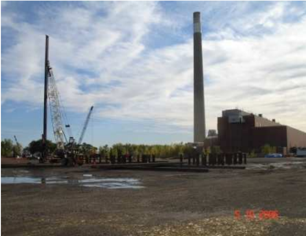
Piling for combustion turbine generators at PEC adjacent to the decommissioned R.L. Hearn G.S.
