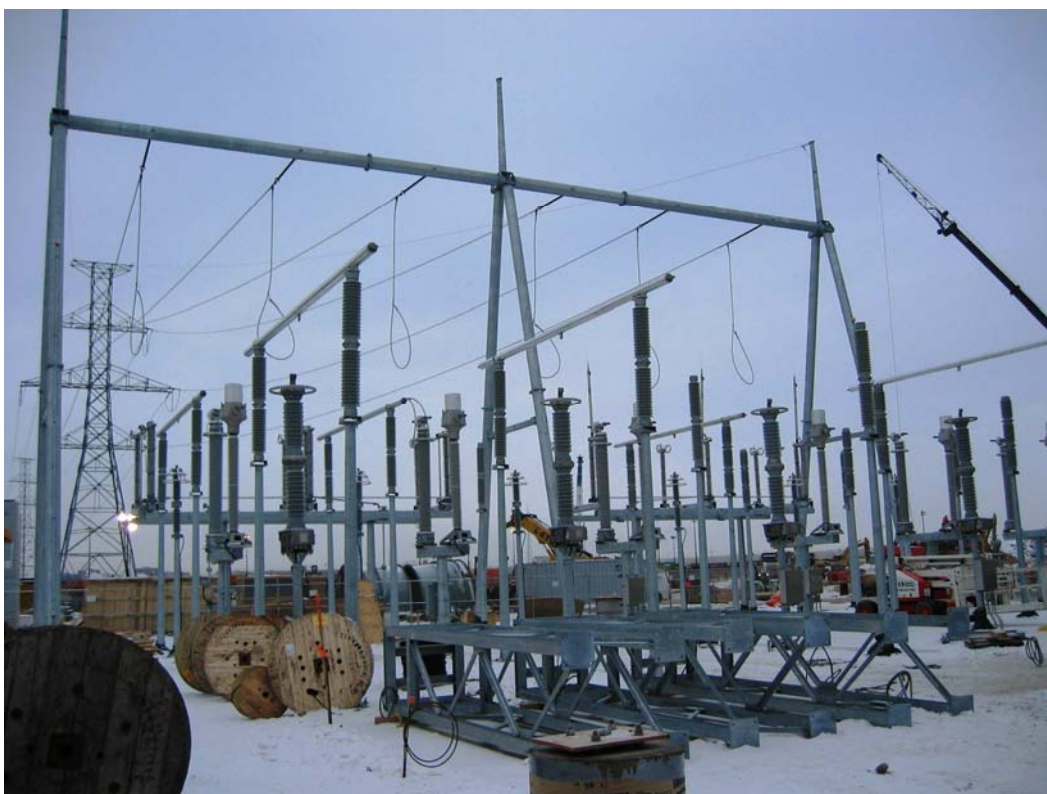
The Goreway switchyard installation in progress
