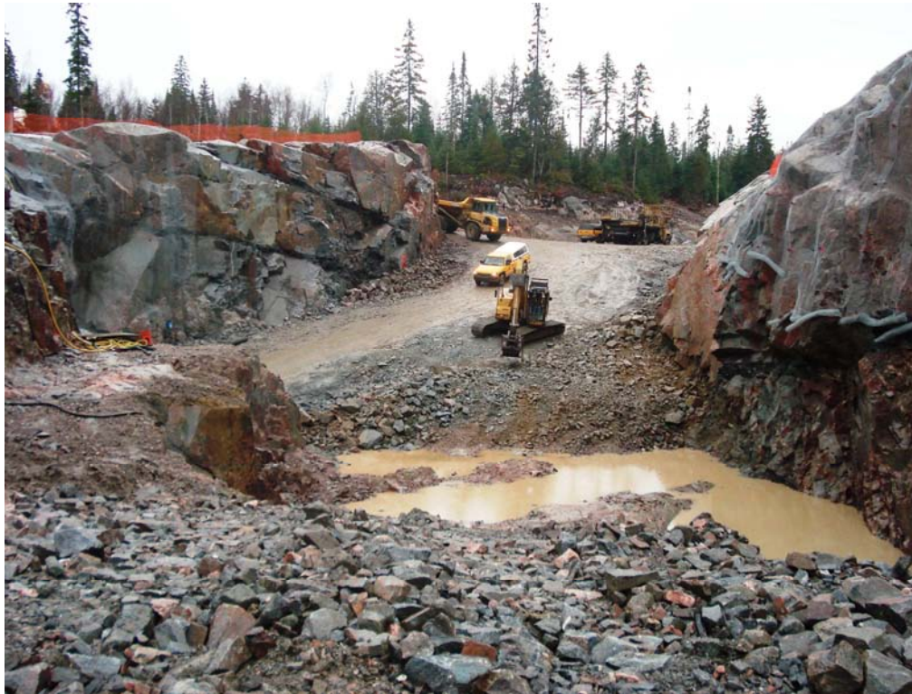
Sluice and division channel for Umbata Falls generating station being excavated
