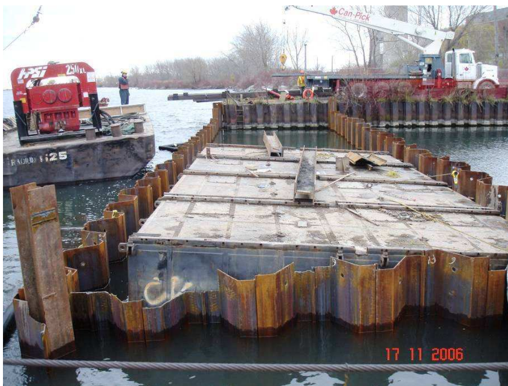
A sheet pile cofferdam at the south end of the discharge channel
