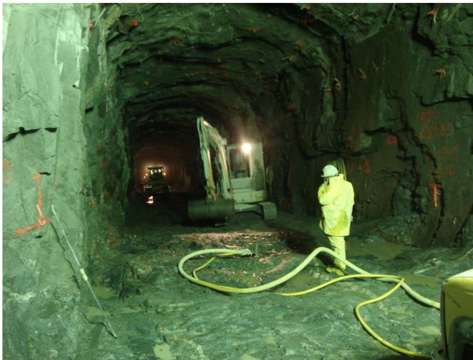
Power tunnel for the Umbata Falls hydroelectric station under construction. The station consists of two Kaplan units with a combined rated flow of 80 cubic metres per second and a net head of 32.8 metres.
