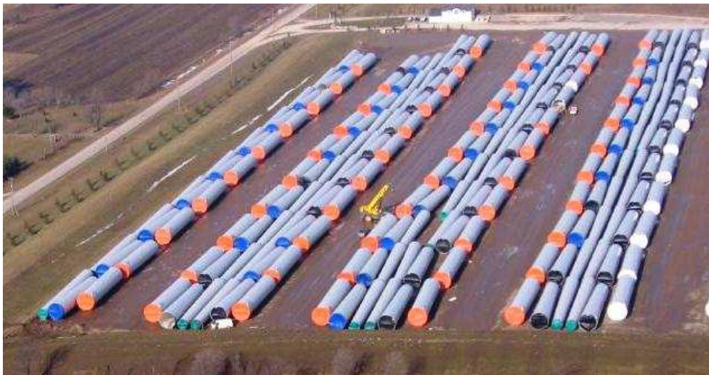
Photos of turbine tower sections for Melancthon II. Phase II consists of 88 towers and each tower consists of three sections. The total weight of the three sections combined is 110 tonnes.
