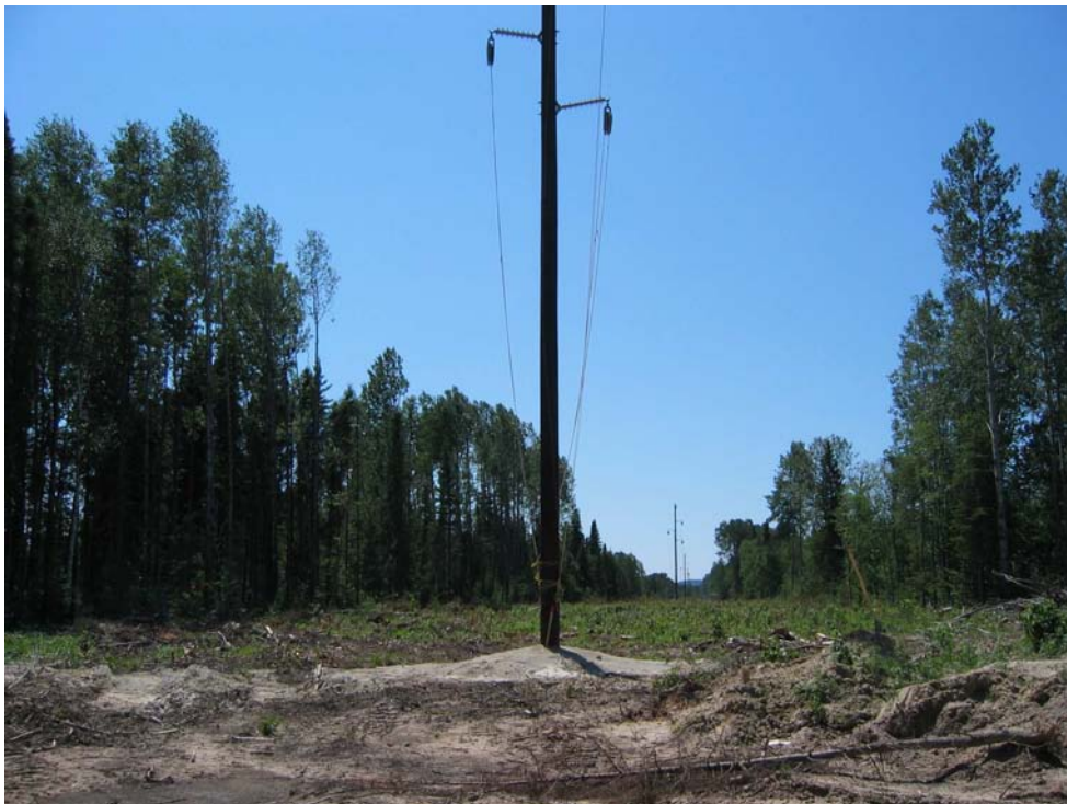
Wood pole structures for 23 km of 115 kV transmission line connecting to the Hydro One system were installed in the summer of 2006.
