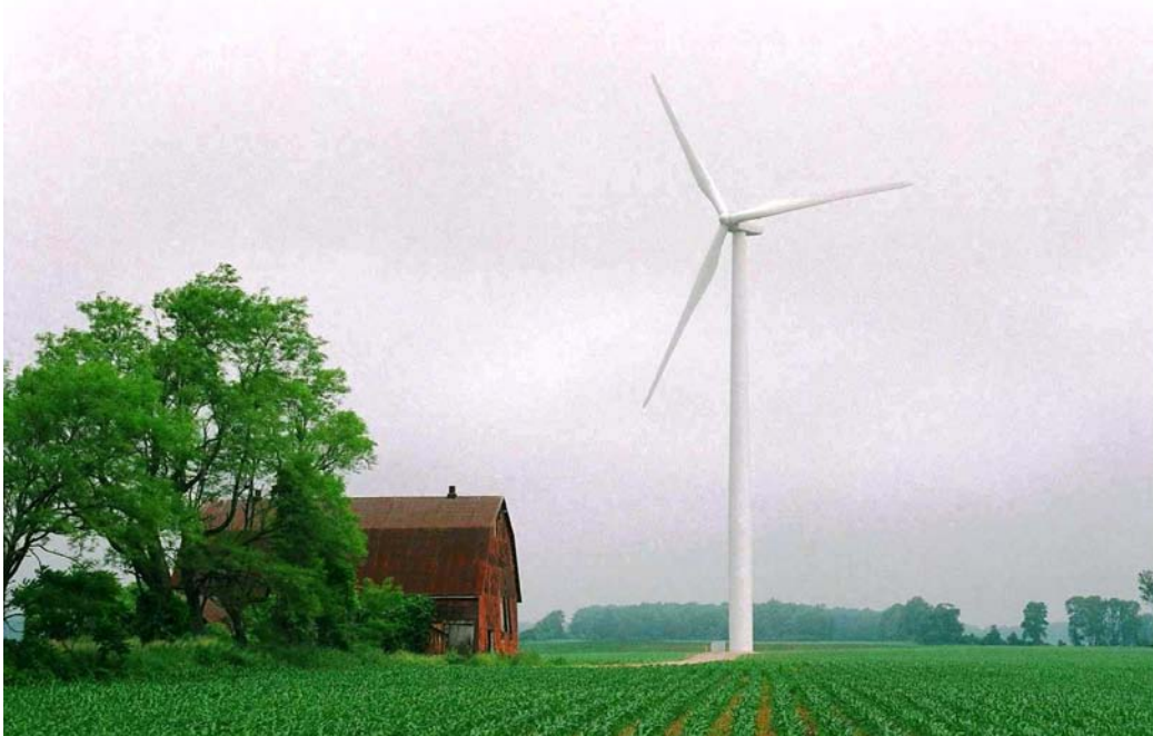
One of the 66 GE 1.5 model SLE wind turbines at the Erie Shores Wind Farm.
