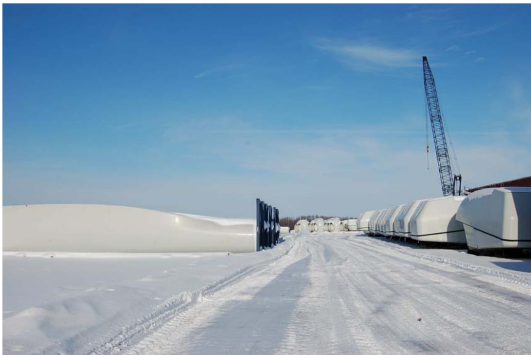
Vestas V82 wind turbine blades, nacelles and hubs for the Enbridge project. This project will install 121 turbines.
