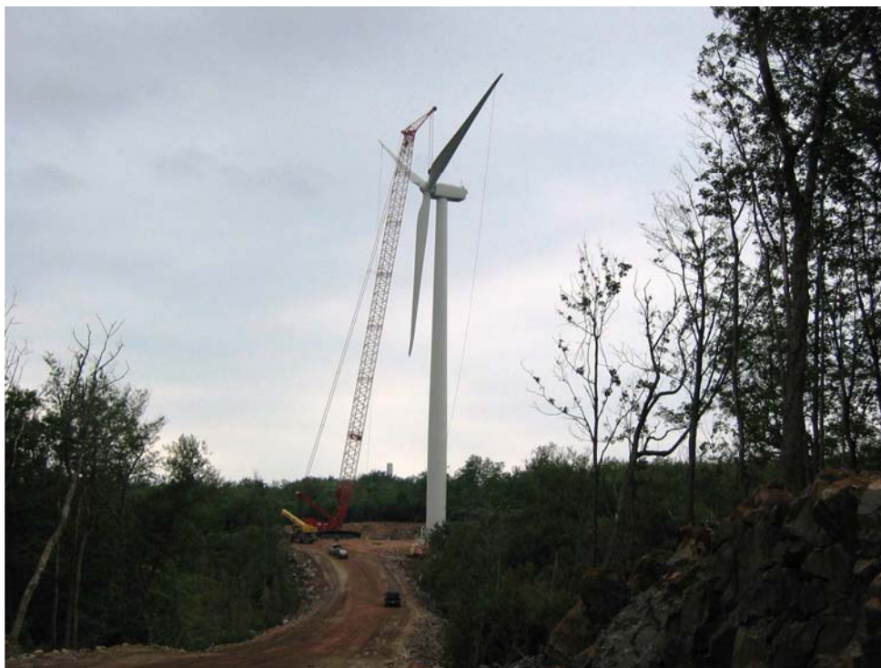
Installing one of the 126 GE 1.5 model SLE wind turbines' rotors at the Prince Wind Farm
