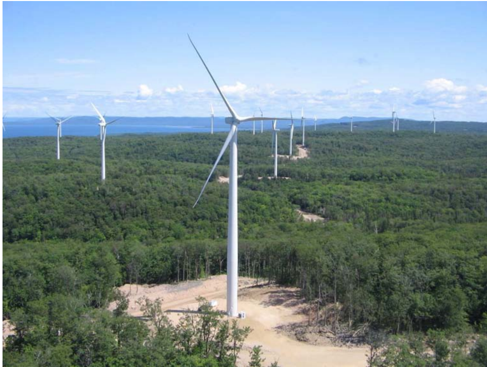
This 189 MW Prince Wind Farm in Sault Ste Marie was placed in commercial operation in the fall of 2006. The project was developed by Brookfield Power.
