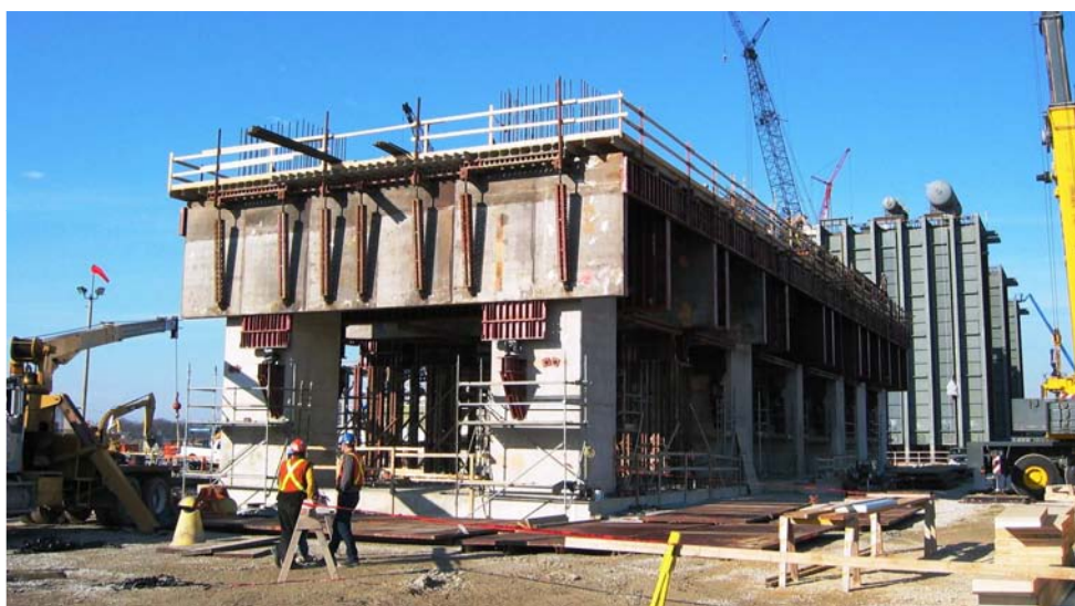
Concrete supporting structure for the 500 MW steam turbine generator at GEC under construction
