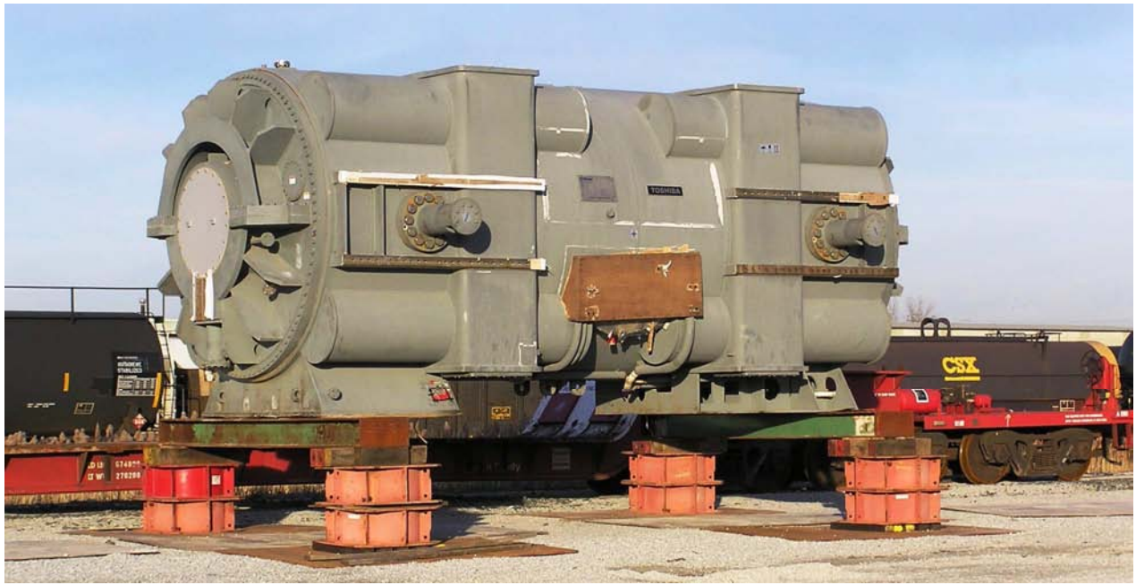
A steam generator delivered to the GEC site
