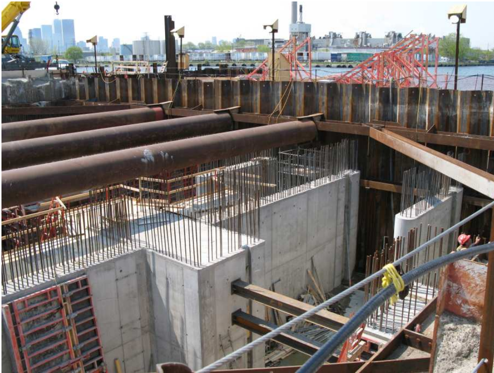
Construction of cooling water intake and pump house at Portlands Energy Centre in progress
