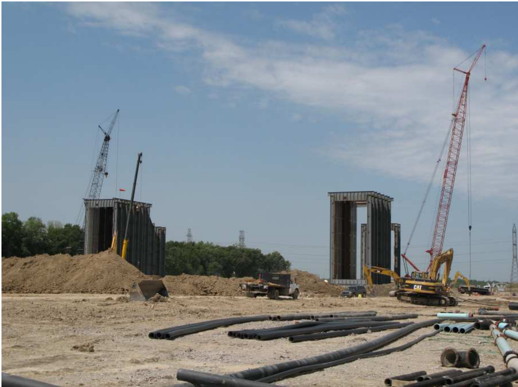
Erection of two heat recovery steam generators has begun at the St Clair Energy Centre
