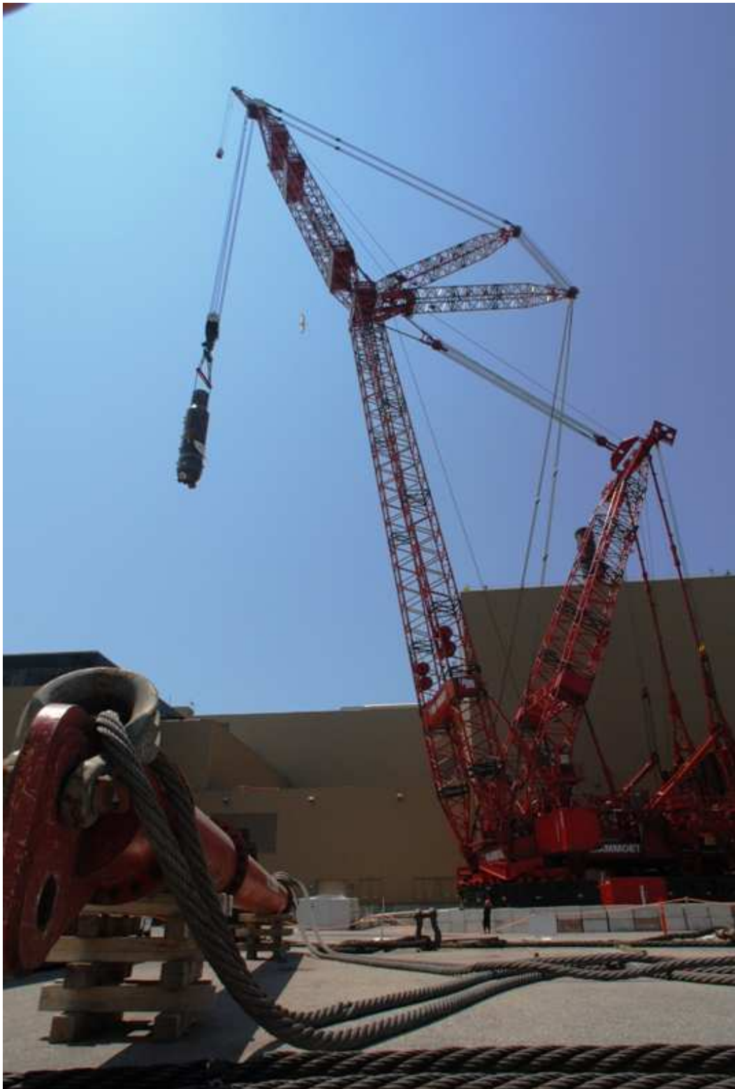
The first new steam generator being installed with the assistance of a 1,600-tonne crane
