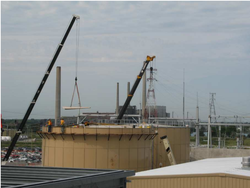
The water storage tank at Greenfield Energy Centre is close to completion
