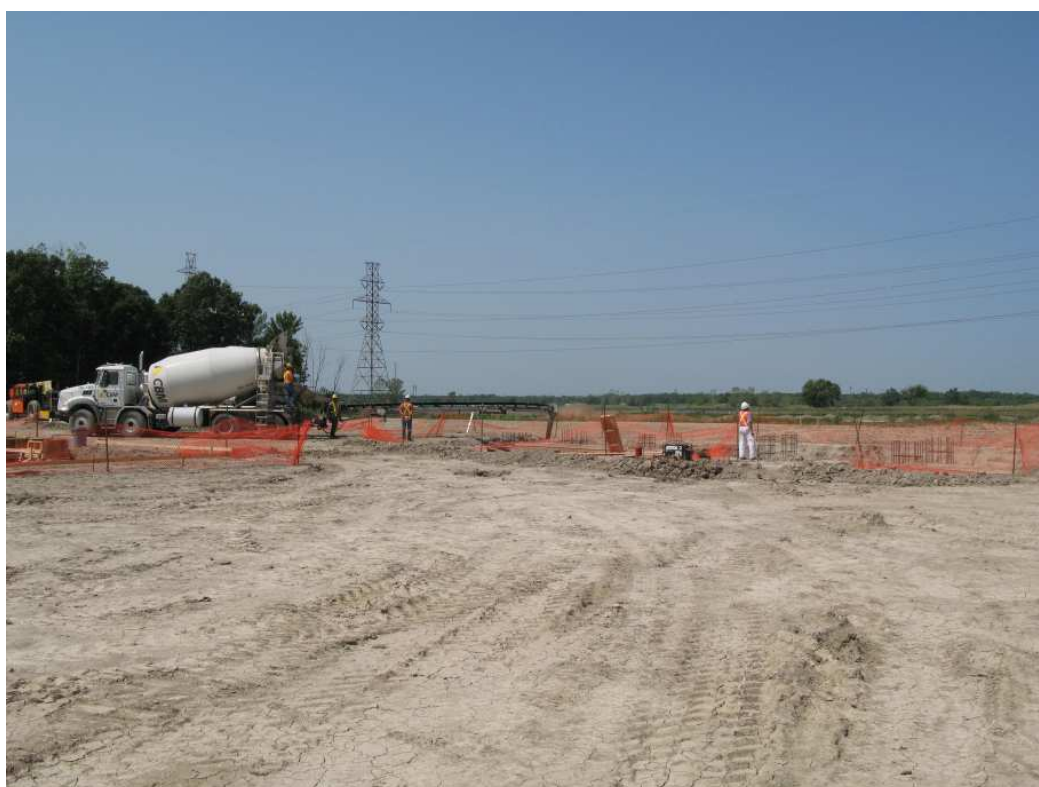
Concreting foundation for the St Clair Energy Centre substation, which is located at the back of the site and adjacent to the Hydro One transmission line
