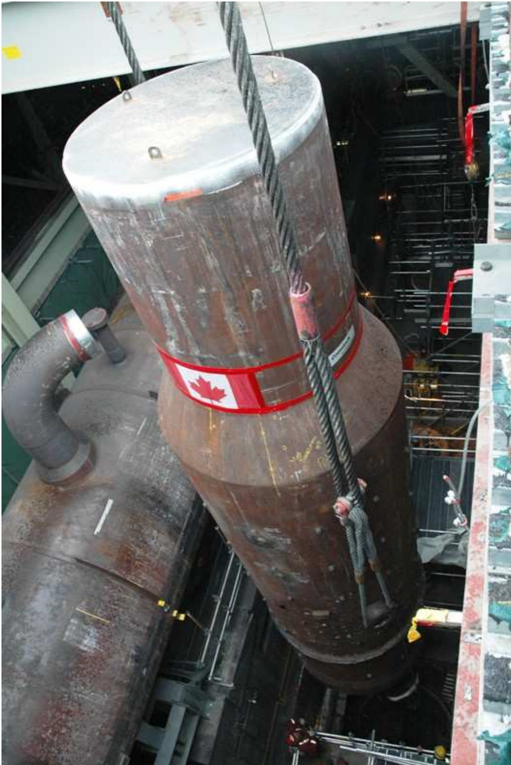
One of the eight 100-tonne steam generators at Unit 2 being removed through an opening cut in the roof of the Bruce A powerhouse
