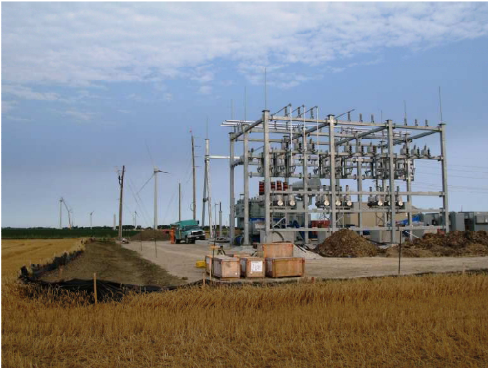
Construction of the "south" substation of the Ripley project is in progress; the "south" substation will step up the energy to 69 kiloVolts (kV) for transmission to the "north" substation for injection into the Ontario power grid
