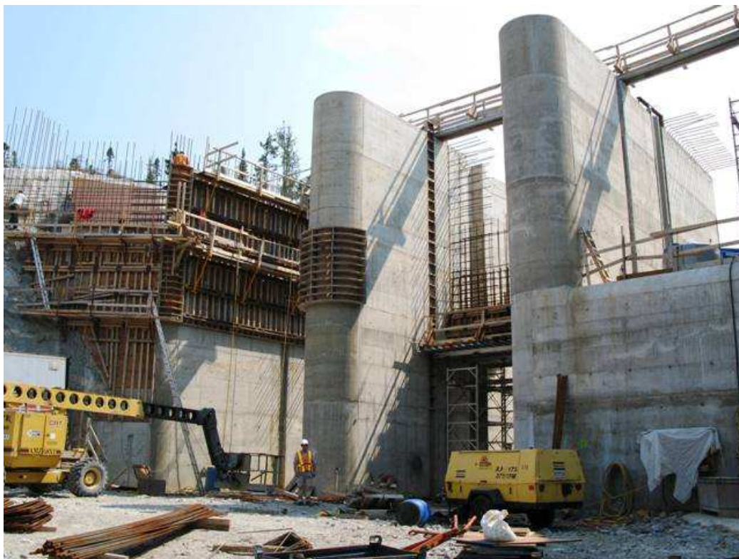
A view of the Umbata Falls sluice structure
