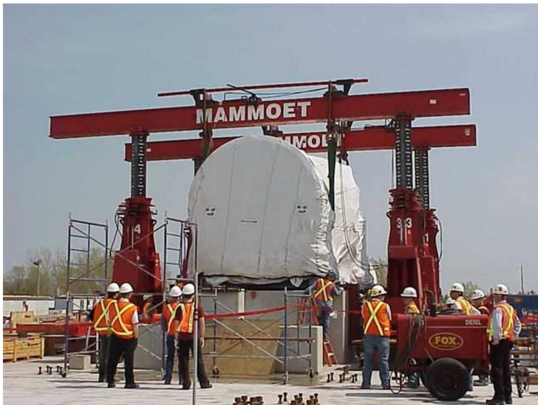
Setting of combustion turbine generator at Portlands Energy Centre
