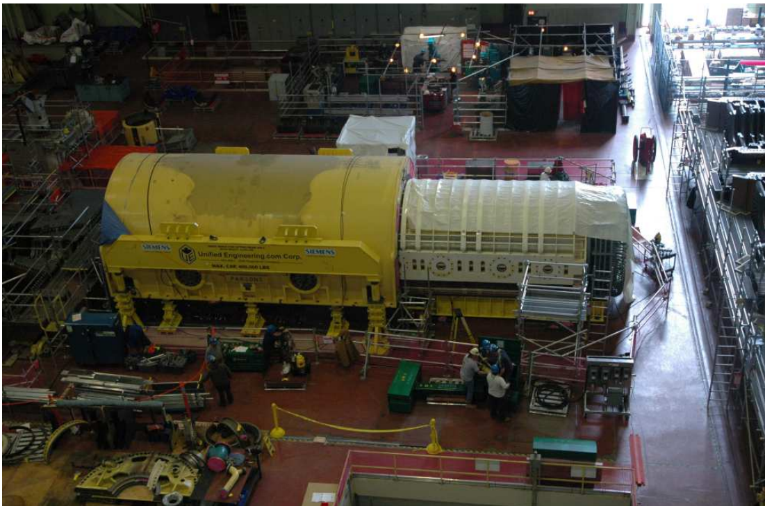
Work crews recently inserted a replacement rotor into the Unit 2 generator and are busy restoring turbine spindles; Siemens is overhauling the turbine generators in both Units 1 and 2 for return to service
