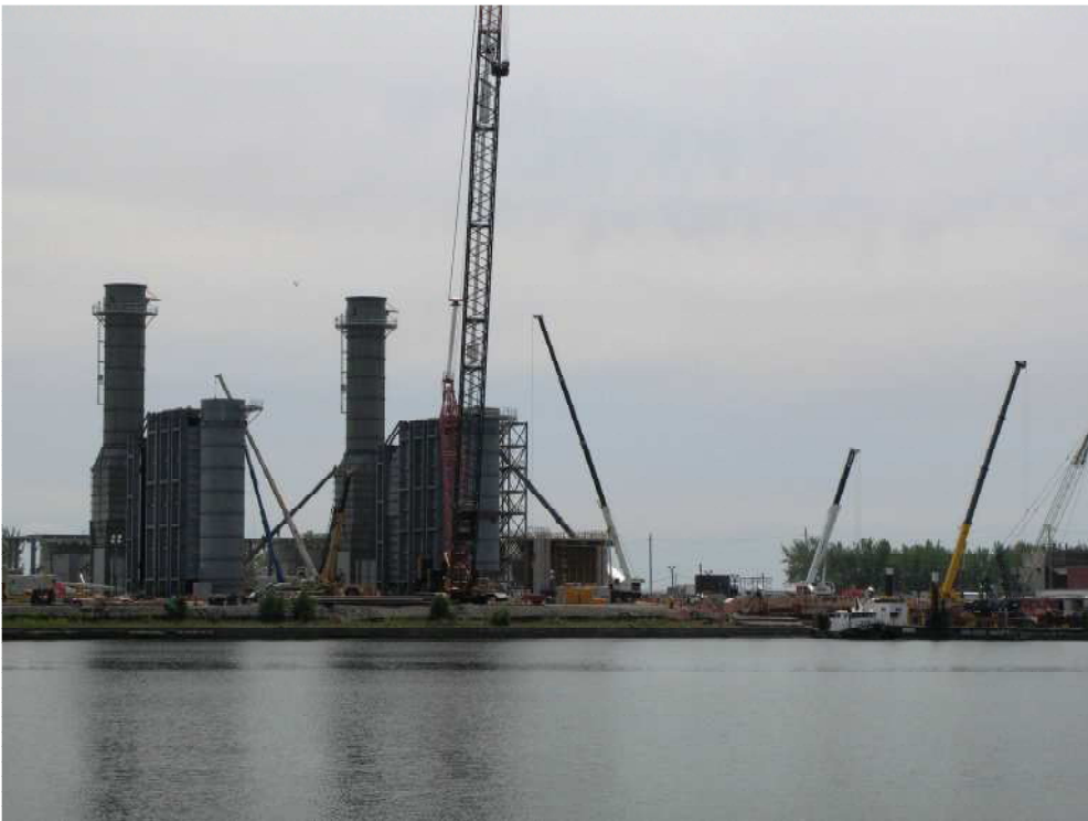
By-pass stacks for simple-cycle operation have been installed and installation of stacks for combined cycle operation is in progress
