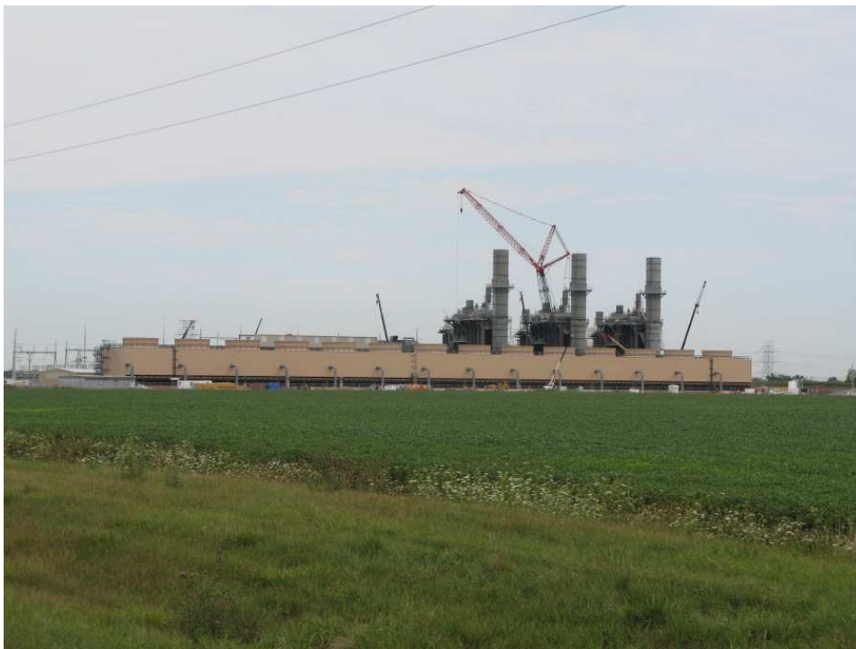
A view of the Greenfield Energy Centre at ground level
