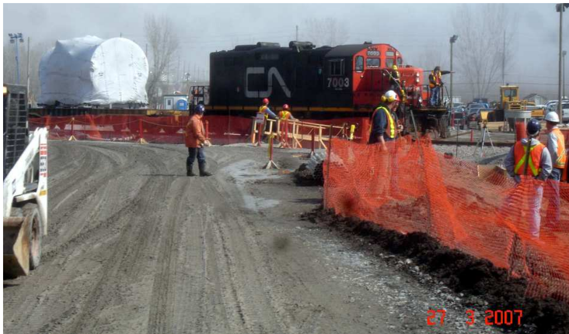
One of the two GE 7FA combustion turbine generators being delivered to the Portlands site via the track that cuts through the site
