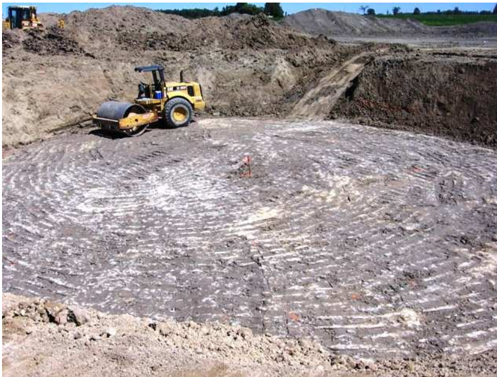
Foundation work in progress for the first wind turbine tower at the Enbridge Ontario Wind Farm
