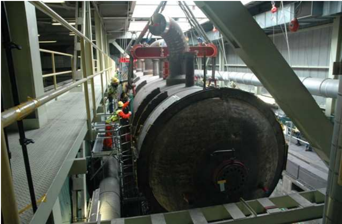
The east steam drum in Unit 2 was lifted aside on April 2, 2007; the vessel, which measures 29.3 metres long by 2.88 metres in diameter, weighs more than 250 tonnes
