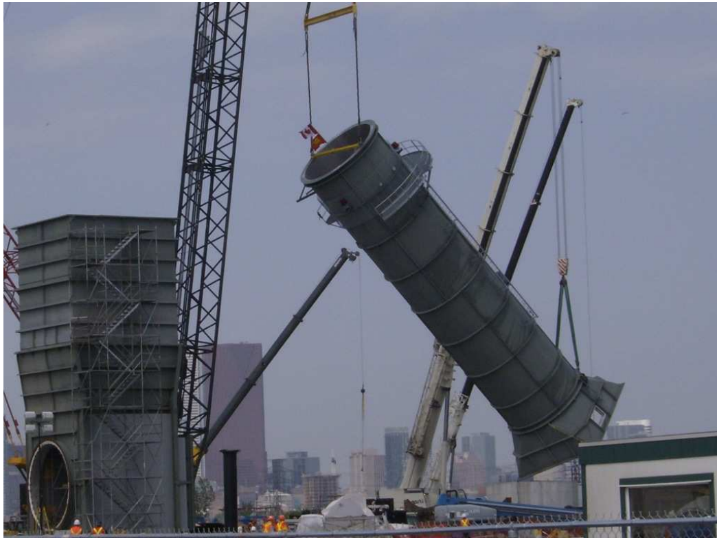
Top section of by-pass stack being installed at Portlands
