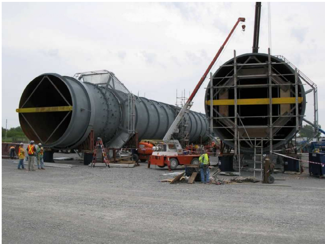
Preparing stack sections for installation at Portlands
