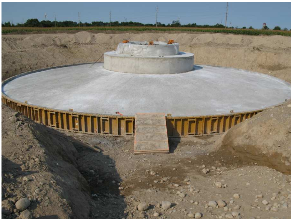
Foundations for ENERCON wind turbines are always circular. As claimed by ENERCON, round foundation has proven to reduce the amount of reinforcement, concrete and formwork
