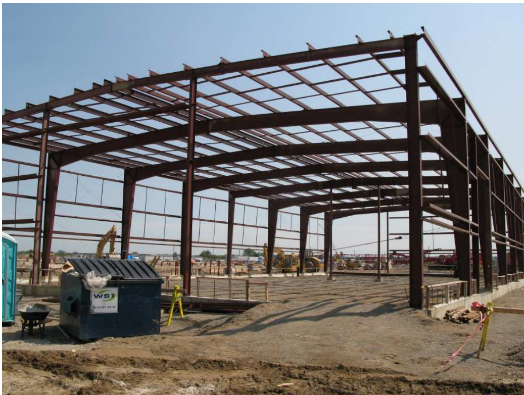
Warehouse at St Clair Energy Centre under construction
