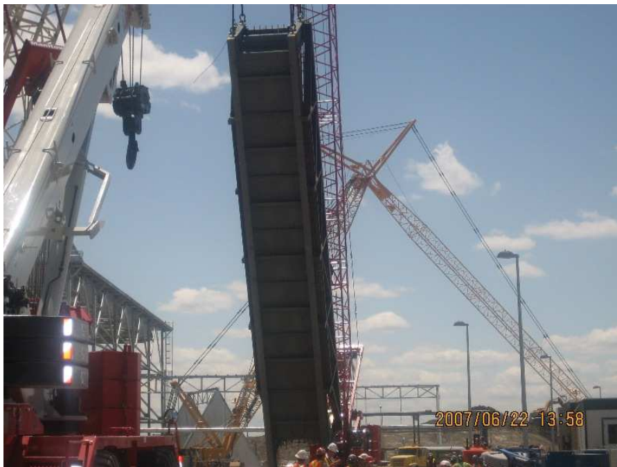
Installation of Heat Recovery Steam Generator module at Goreway Station
