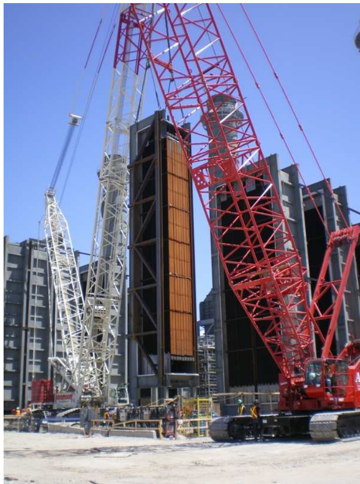
Another view of Heat Recovery Steam Generator module installation
