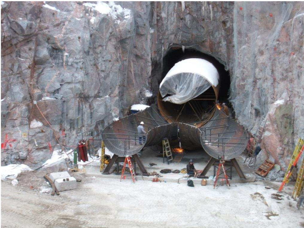
Fabrication of the "Y" bifurcation and welding of steel penstock in progress
