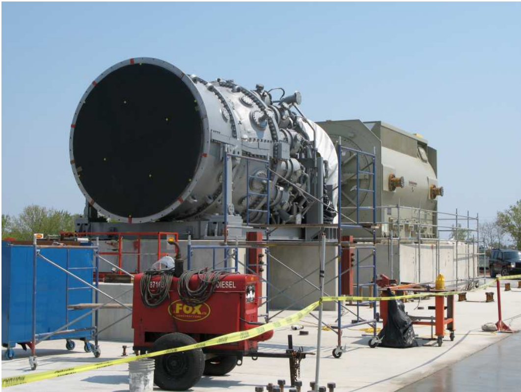
One of the two Portlands combustion turbine generators set on foundations.
