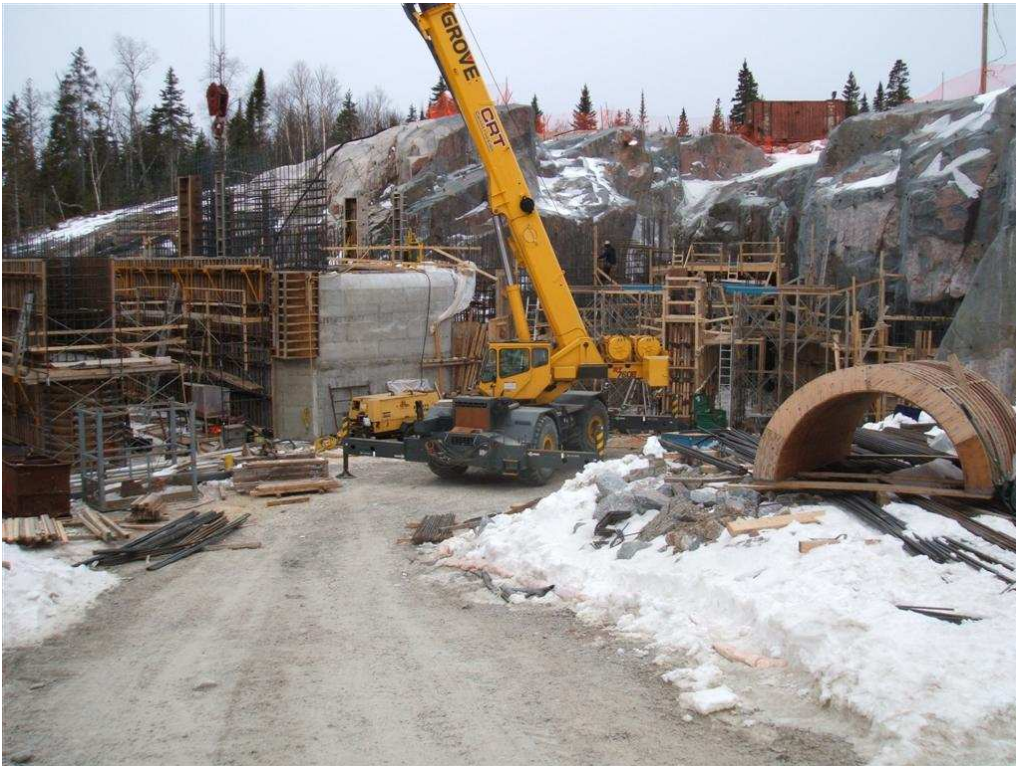
Intake and sluice structure under construction
