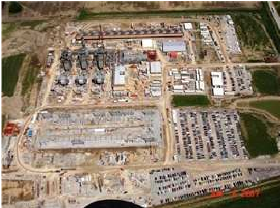
Bird's-eye view of the 1,005 MW Greenfield Energy Centre at Sarnia; the project adopted a "3-on-1" configuration with three Siemens Westinghouse 501FD2 combustion turbine generators, three heat recovery steam generators and one 500 MW Toshiba steam turbine generator; construction started in November 2005 and is targeted to be in service in the fall of 2008
