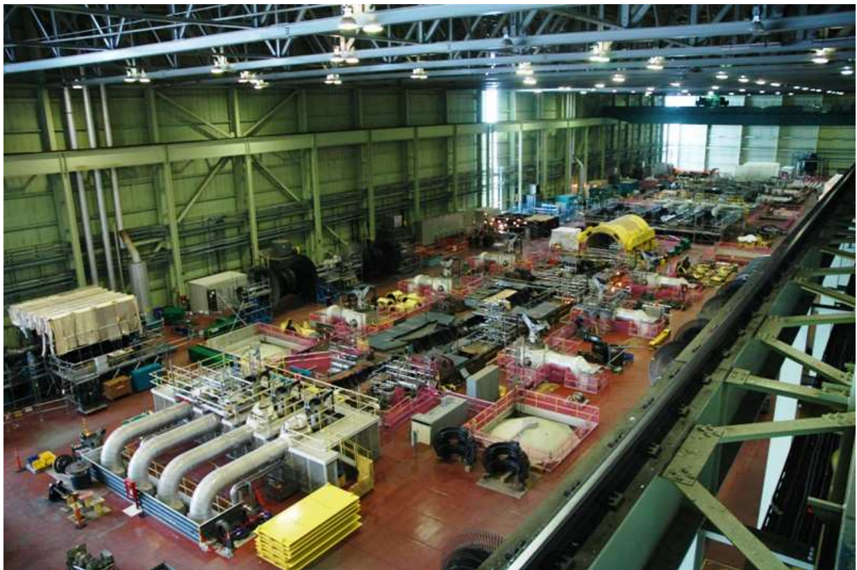
Work in progress on overhauling turbine generators in Units 1 and 2 at Bruce A
