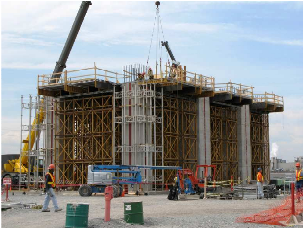
Supporting structure for steam turbine generator in progress
