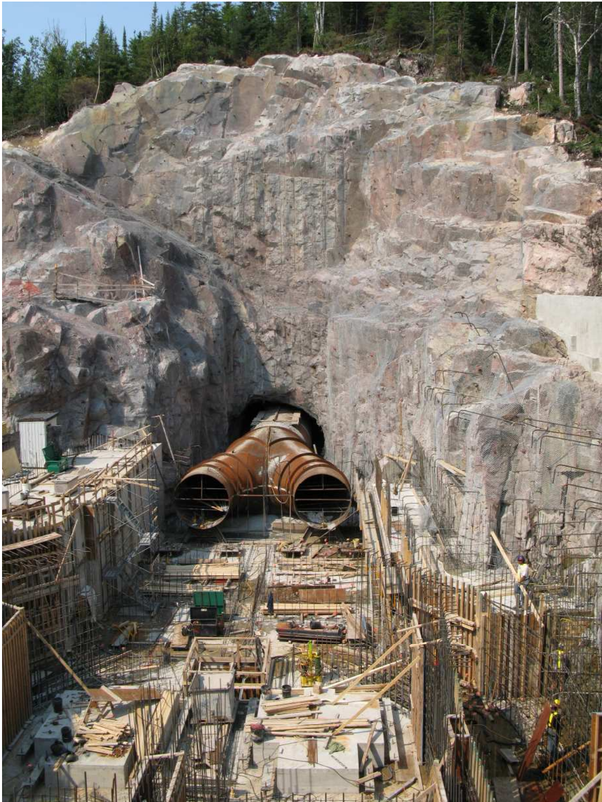
“Y” bifurcation and the Umbata Falls powerhouse under construction
