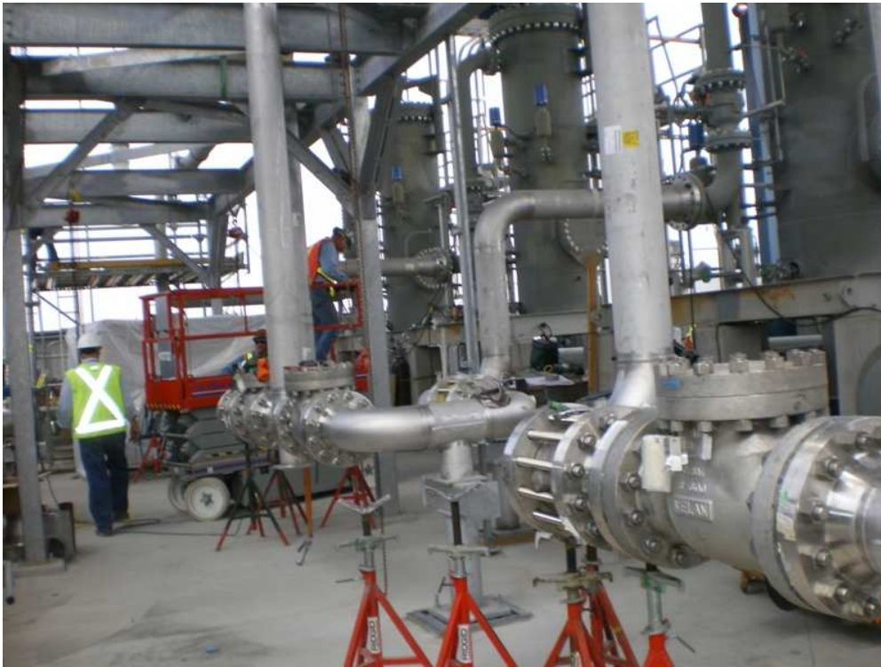
Fuel gas filter building at Goreway Station
