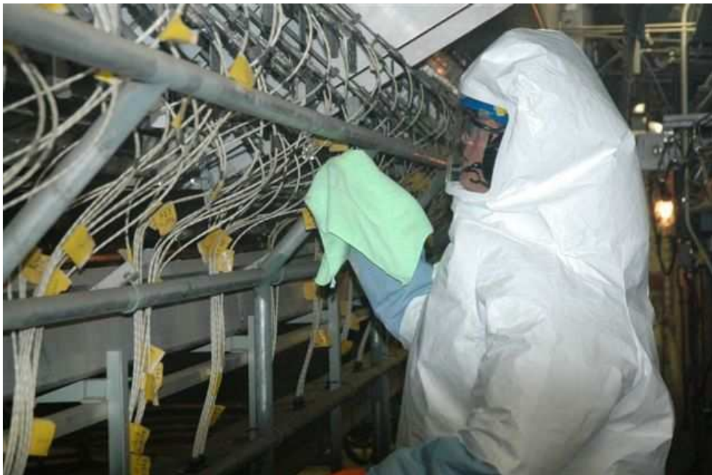
A member of the Radiation Protection team works to decontaminate the inside the Unit 1 reactor vault; it has to be cleaned up enough to allow work to proceed without the need for air-supplied plastic suits
