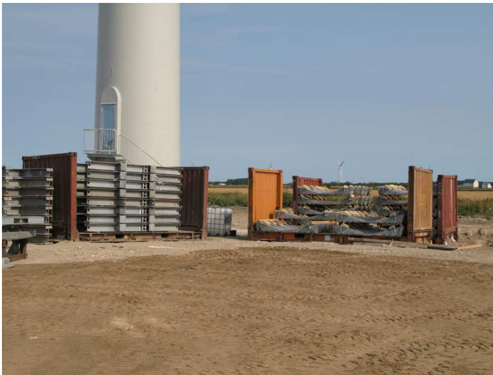
Packing materials for the delivery of wind turbines will be re-packed and returned to ENERCON in Germany for future shipments to another project site
