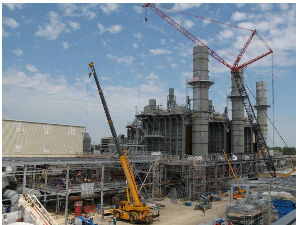
Approximately 90 percent of mechanical installation at Greenfield Energy Centre completed; scheduled commercial operation is the fall of 2008
