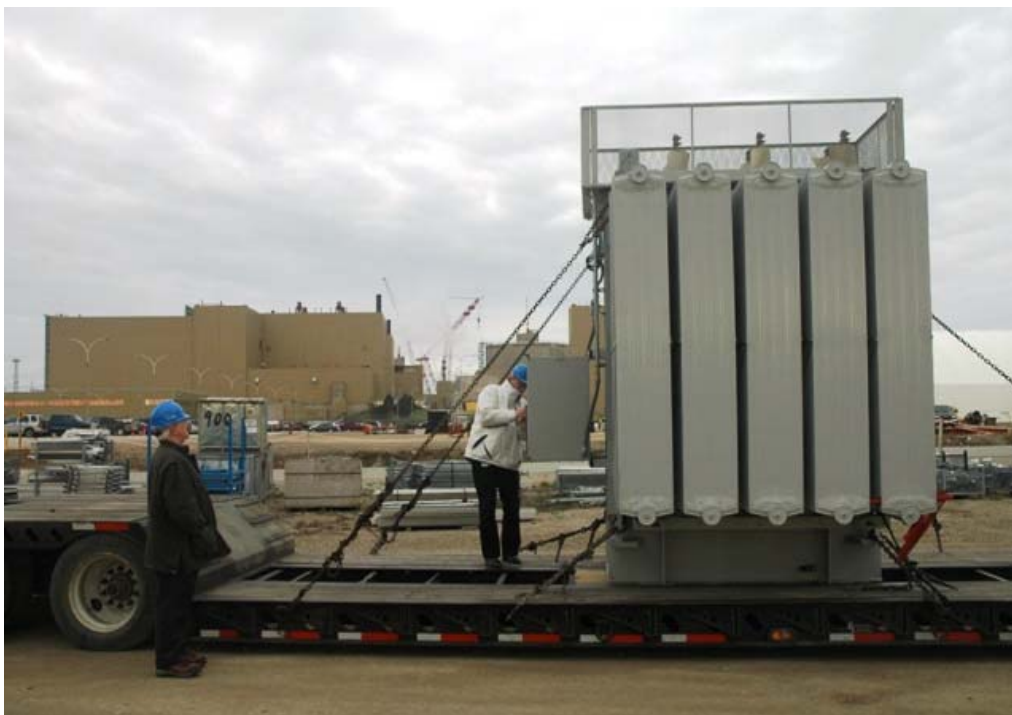
The first of 36 new transformers arrived at Bruce A. Transformers in Units 1 and 2 are being replaced during the Restart Project with new air-cooled units that do not use polychlorinated biphenyls (PCBs).
