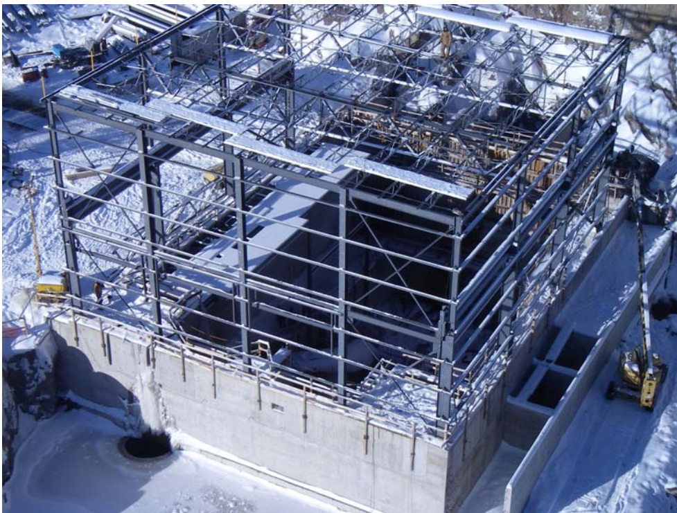
Erection of the structural steel frame for the powerhouse superstructure is in progress.
