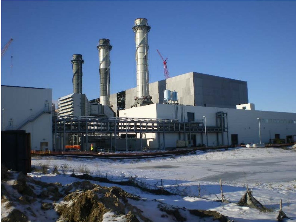
Northwest view of the Goreway Station .
