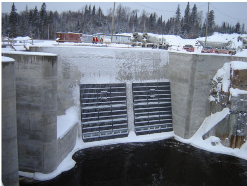
Intake structure is complete with trash racks covering the power tunnel entrance.
