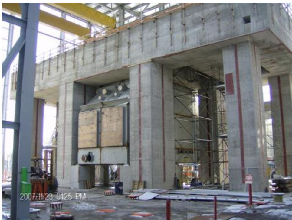
Below the table top, a surface steam condenser has been placed in its final position.
