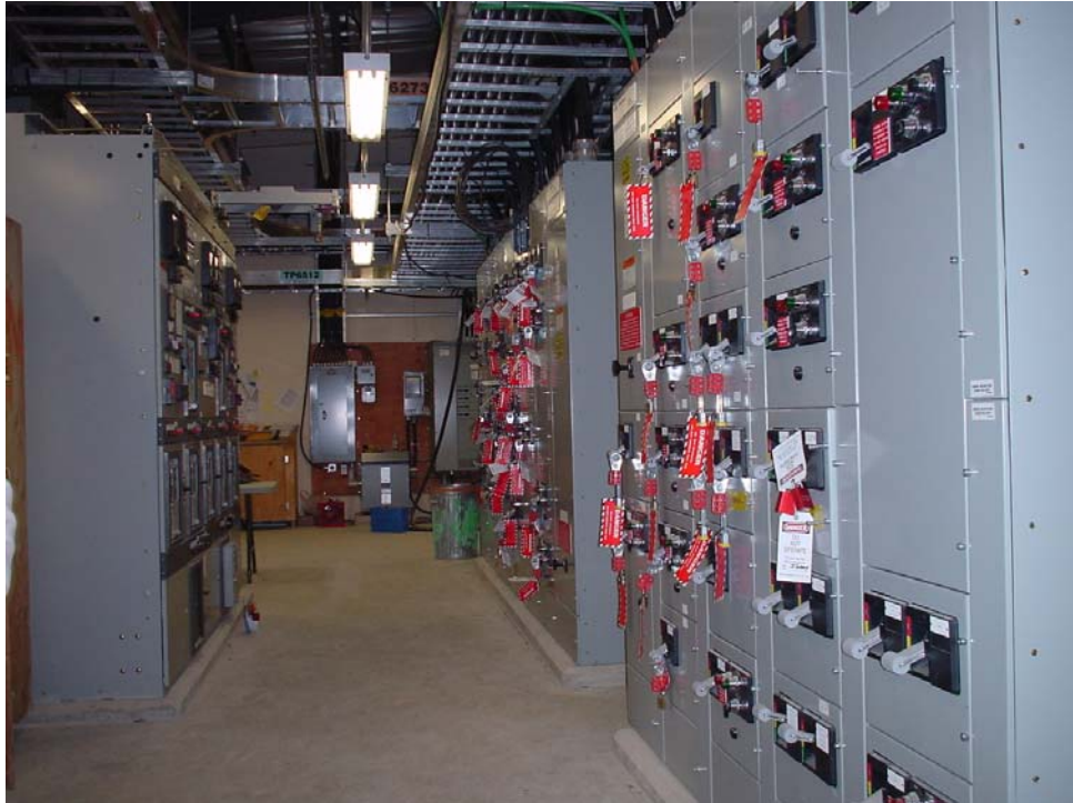
Installation of electrical equipment is complete. Testing and commissioning is in progress.
