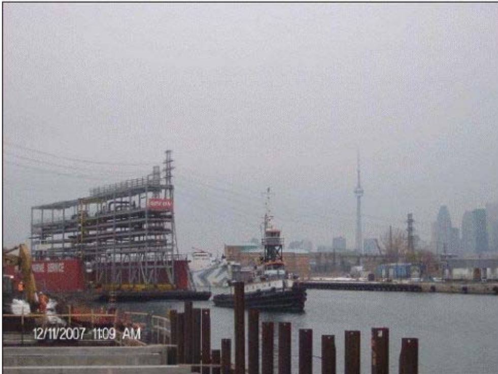
Two utility rack modules are shown arriving from Halifax. The modules were off-loaded directly onto the project site from the shipping channel.
