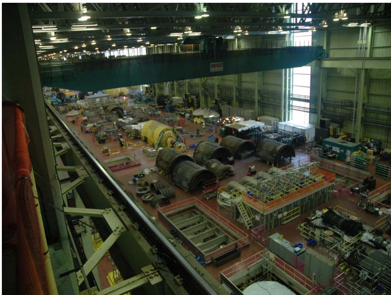
The entire generator floor inside the Bruce A powerhouse is used for the Units 1 and 2 Restart Project.
