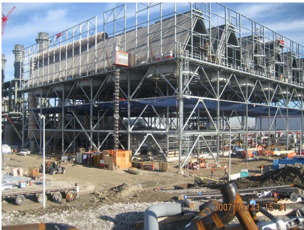
Assembly of the air cool condenser is in progress.
