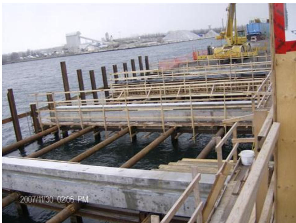
Construction of the intake channel structure at the north side of the pump house is in progress. Precast concrete slabs will be placed on these supports to form part of the 15-metre wide promenade on the north side of the facility site.
