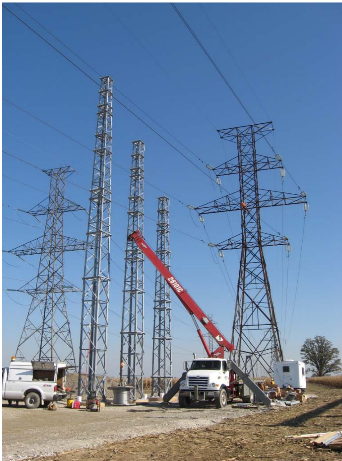
Installation of lattice steel structures for interconnection to the Hydro One 230kV transmission system is in progress.
