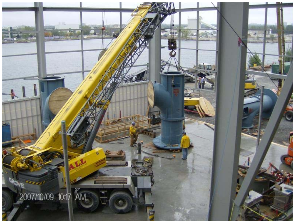
Installation of the main circulating water pump inside the pump house is in progress.
