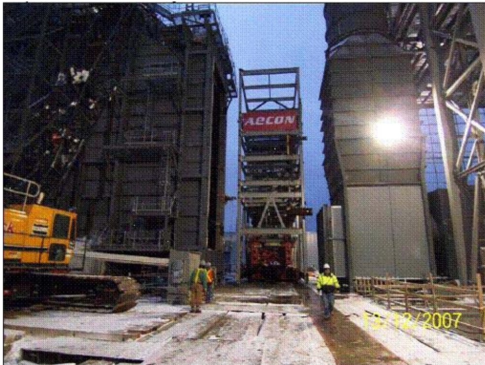
One of the utility rack modules is being moved into position.
