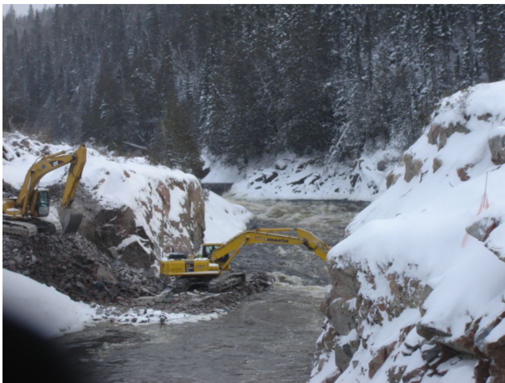
Final excavation of the diversion channel is in progress.
