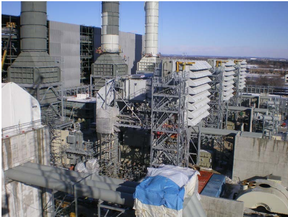
Filter houses of the combustion turbine generators.
