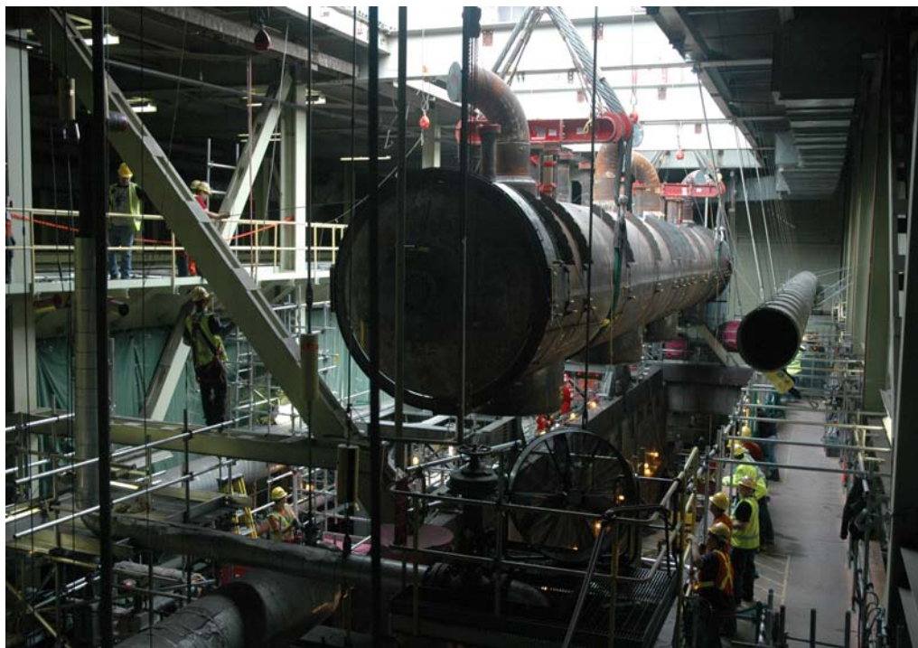
One of the two steam drums of Unit 1 is being lifted back into position after the new steam generators were installed.
