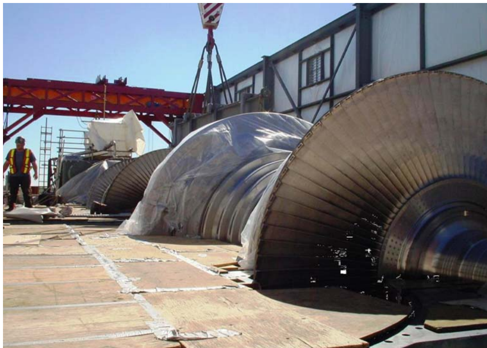
Installation of the 500 MW Toshiba steam turbine.
