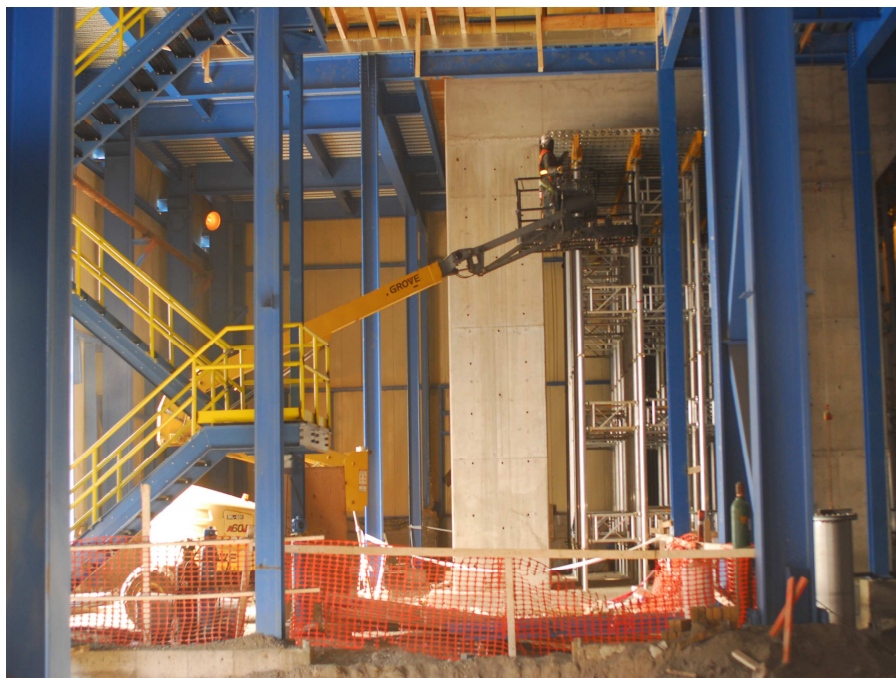
Work on structural steel frame being done inside the CHP building at the Algoma Energy Cogeneration Facility .
