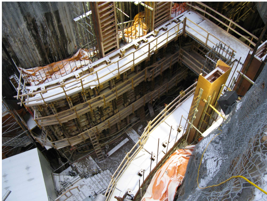
Progress at the Lac Seul GS intake as of the end of 2007
