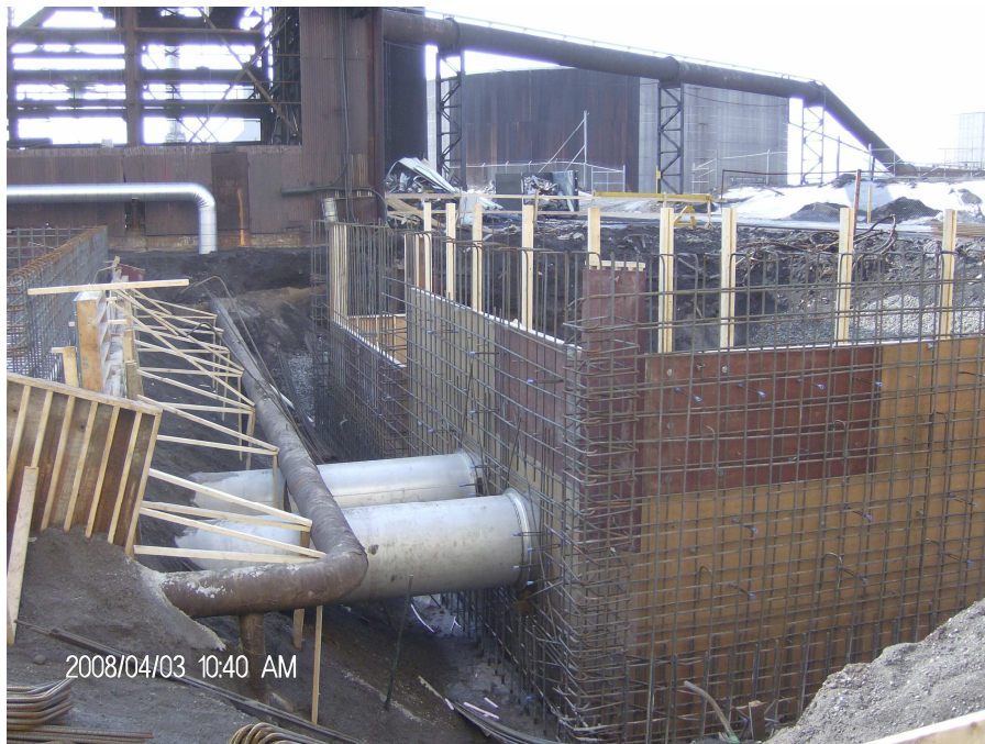
Work on the cooling tower foundation of the 63 MW Algoma Energy Cogeneration Facility in Sault Ste. Marie is underway. COD is expected in the summer of 2009.
