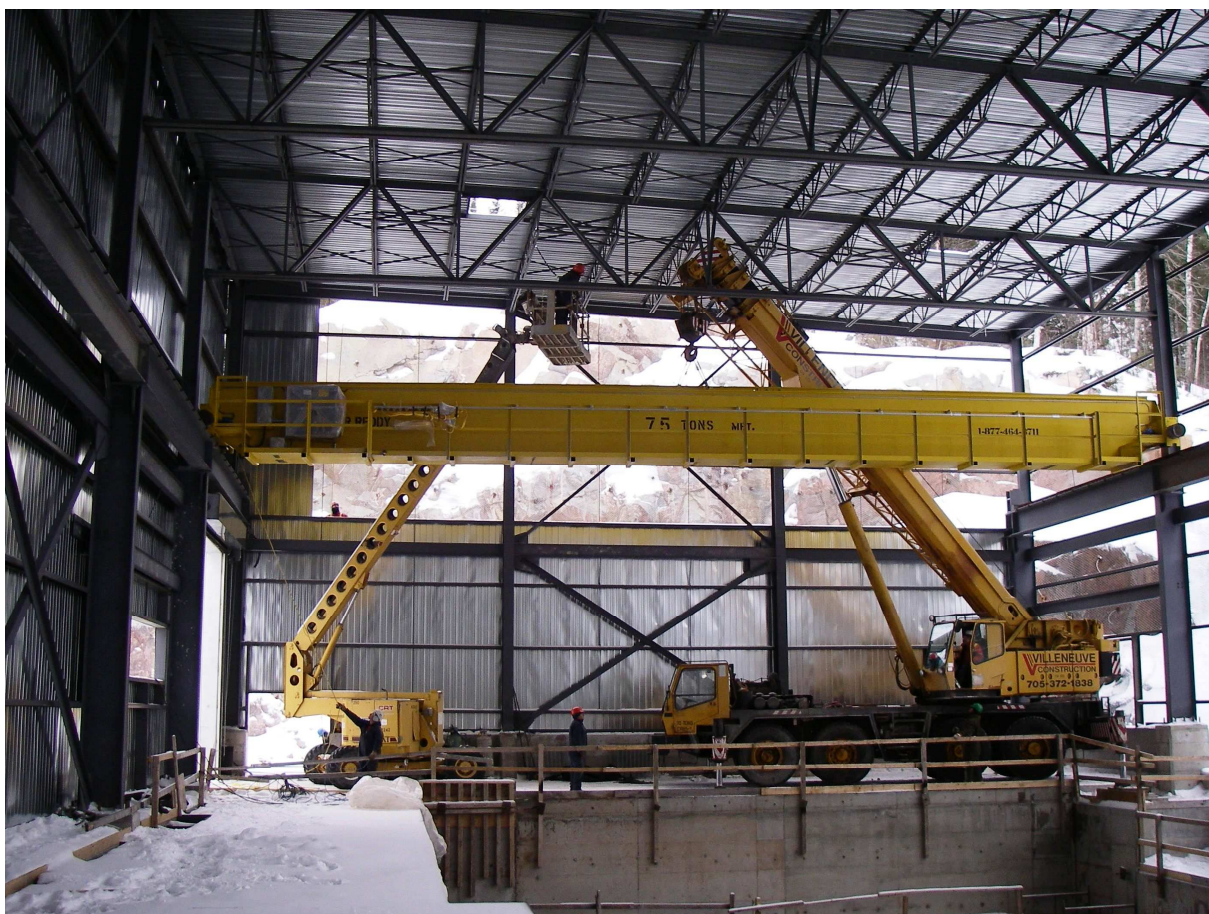
A 75-ton bridge crane is being installed inside the powerhouse at the 23 MW Umbata Falls Hydroelectric Project near Marathon; the project is targeted to achieved COD in the fall of 2008.
