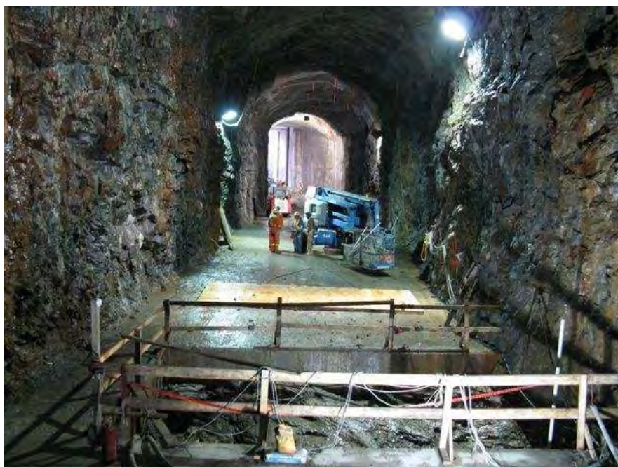
General cleaning of the power tunnel at the Lac Seul Generating Station
