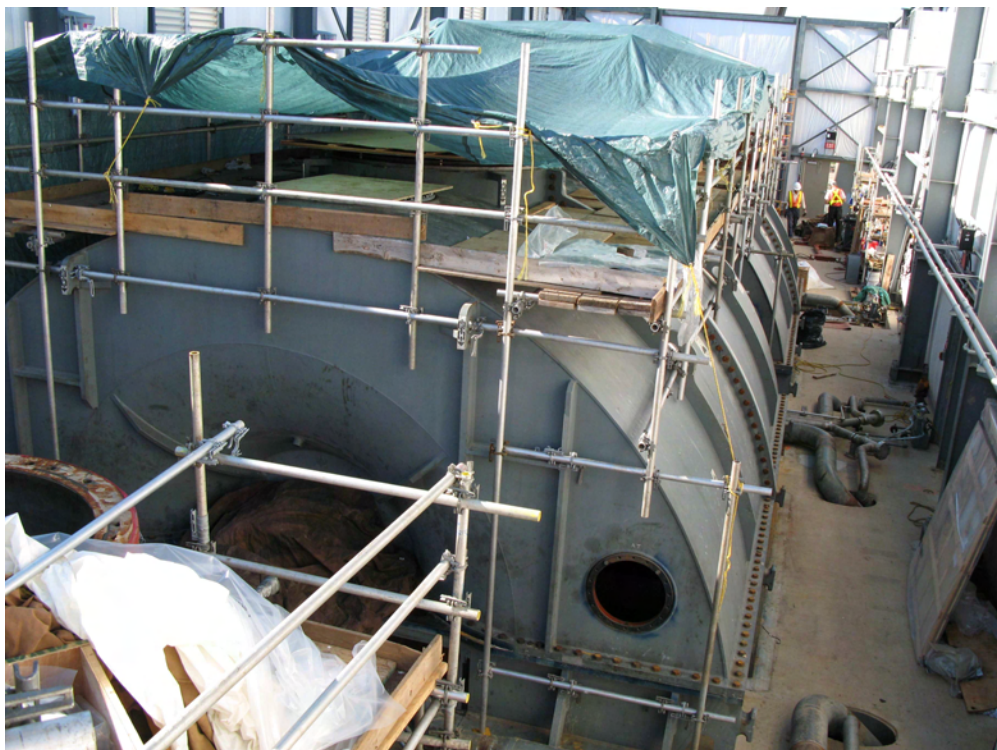
Assembly work continues at the 500 MW Toshiba steam turbine at the Greenfield Energy Centre
