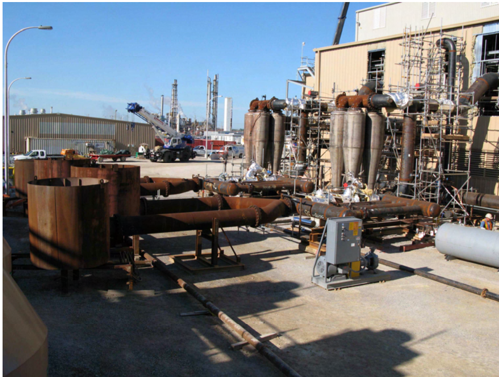
Temporary setup for cleaning steam circuits at the Greenfield Energy Centre
