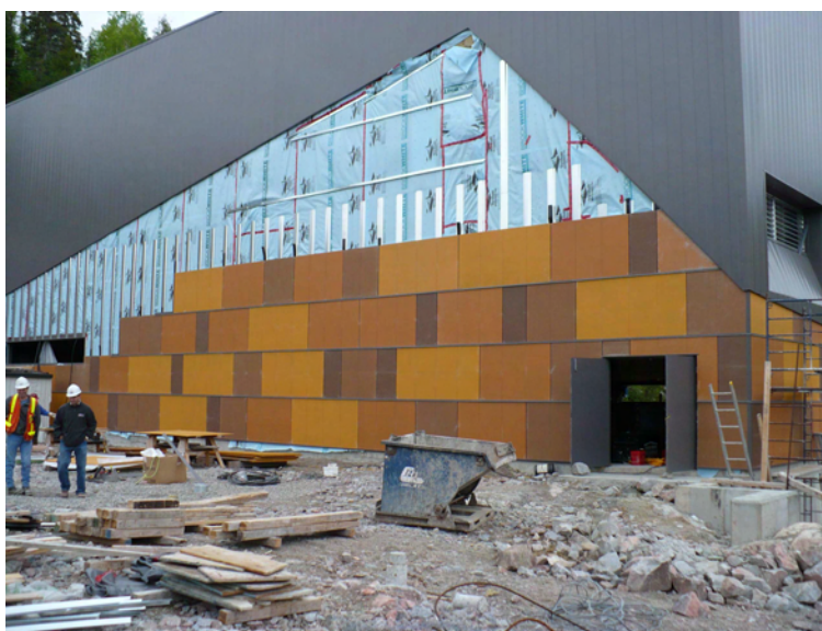
Powerhouse construction for the Umbata Falls hydroelectric generating station is in progress
