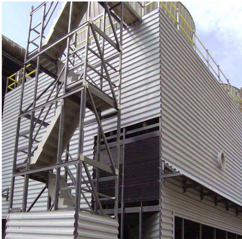
Algoma Energy Cogeneration cooling tower construction nearing completion
