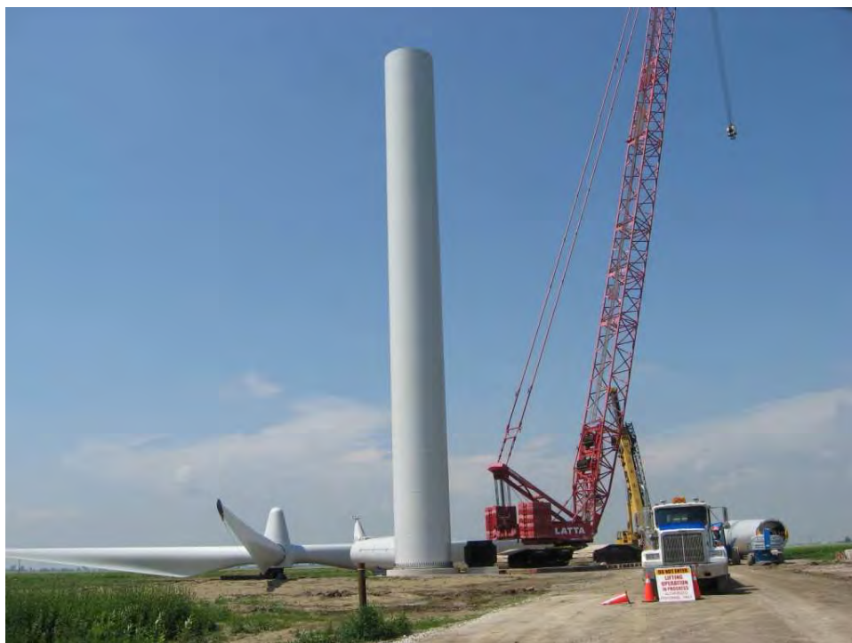
One of the 44 wind towers at the Kruger Energy Port Alma Wind Farm is in the final stage of preparation for installation of the remaining sections of the tower, nacelle and rotor
