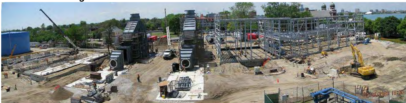
West view of the East Windsor construction site
