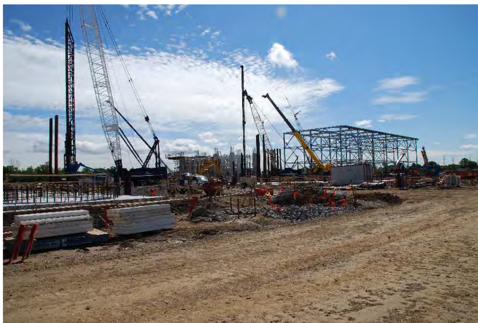
Piling and concrete foundation work continues
