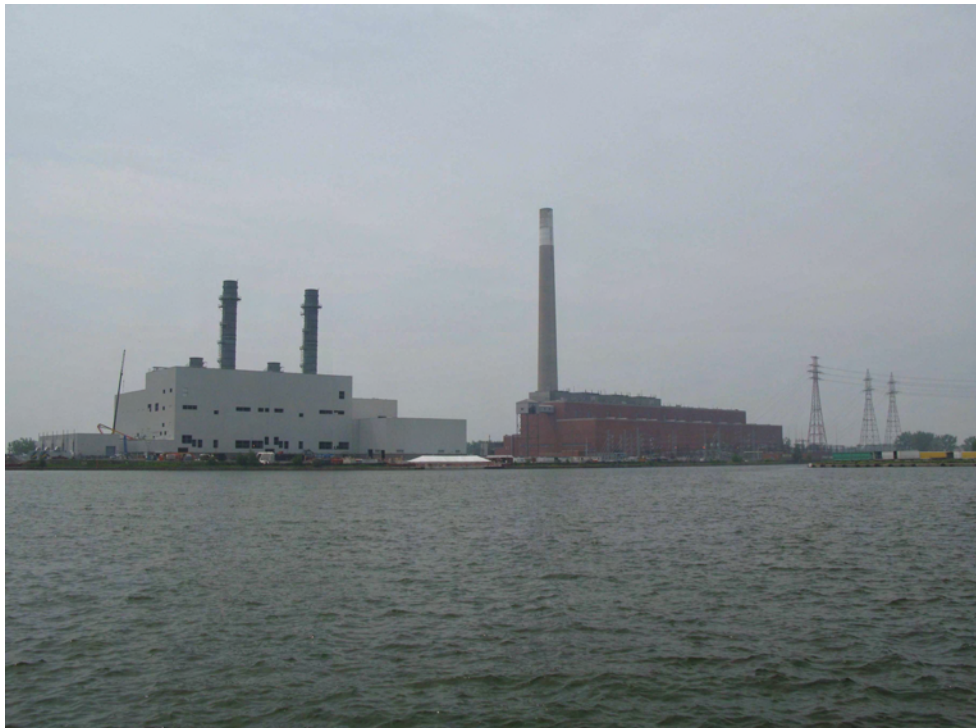
The new 550 MW natural gas-fired Portlands Energy Centre (left) next to the decommissioned 1,200 MW R.L. Hearn coal-fired generating station
