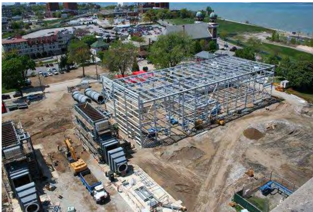
Balance of plant building nearing completion of structural steel installations
