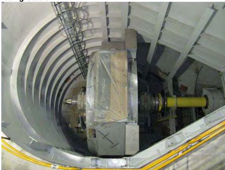
Generator reassembly after machining at the Lac Seul Generating Station
