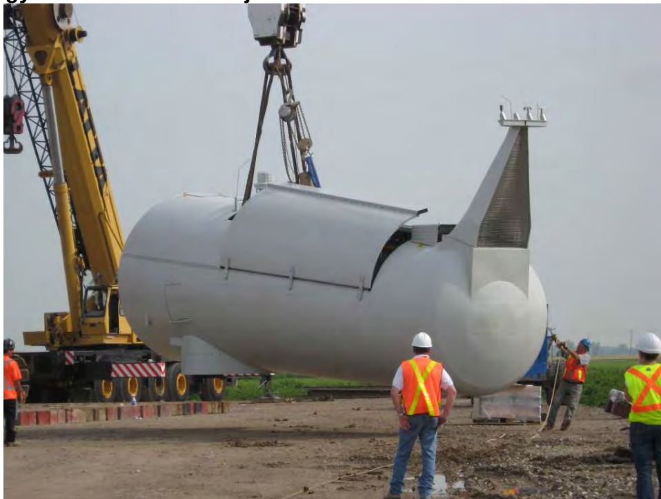
An 82 tonne nacelle for the Siemens 2.3 MW MK II wind turbine is being lifted off the ground for installation at the Kruger Energy Port Alma Wind Farm at Port Alma
