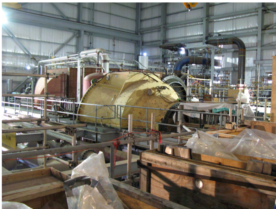
Installation of one of the two steam turbine generators at St. Clair Energy Centre is in progress
