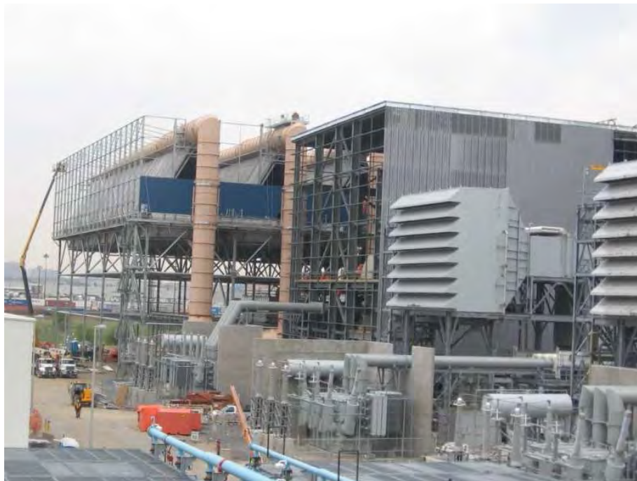
Work at the air-cooled condenser which is located next to the steam turbine hall continues
