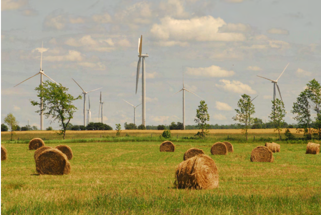
Some of the installed Vestas V82 turbines at the Enbridge Wind Farm awaiting commissioning and testing
