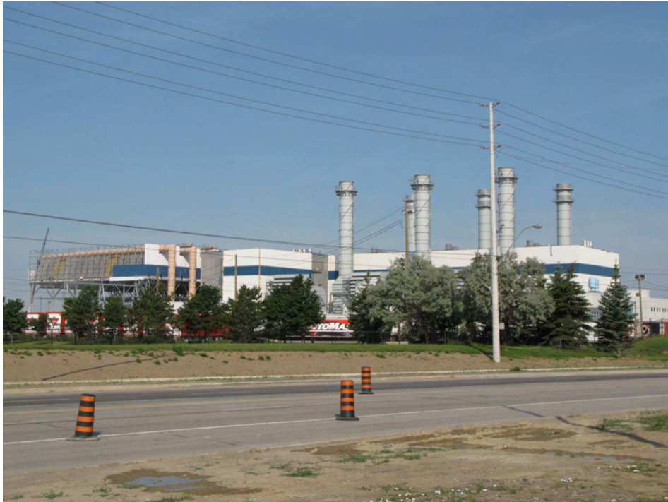
A view of the Goreway Station from Goreway Drive
