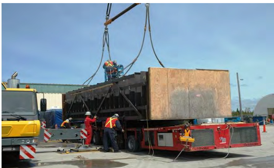
A crane lifts a new condenser tube bundle at the north warehouse near Bruce A
