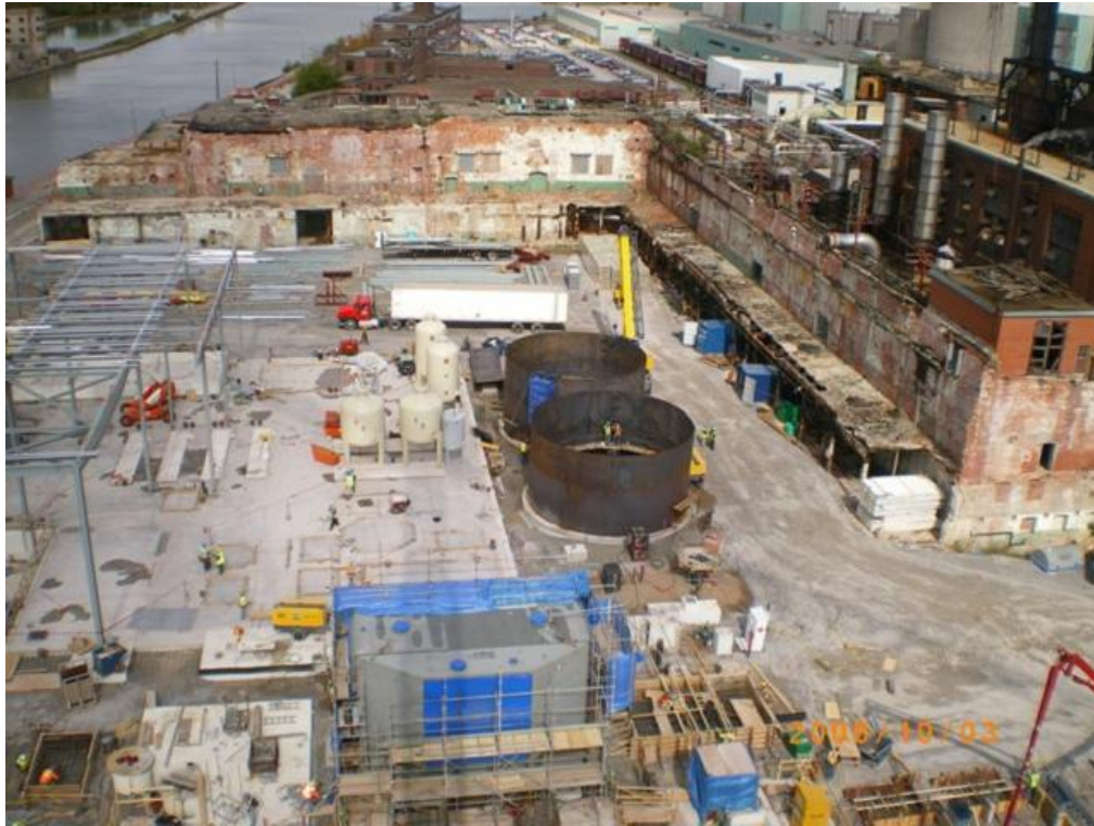
Work continues on the water treatment plant at the Thorold Cogeneration Project
