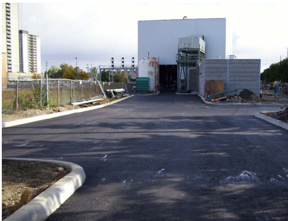
Exterior view of Countryside London Cogeneration facility
