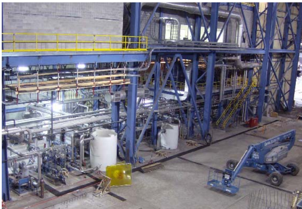
Work continues at the Algoma Energy Cogeneration water treatment plant
