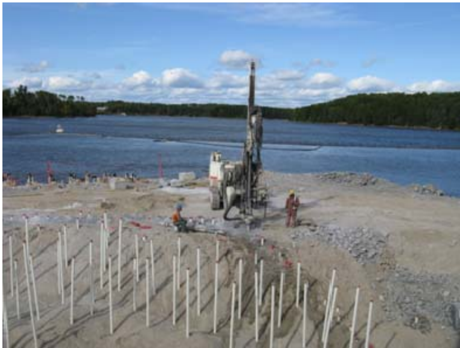
Intake drilling continues at the Lac Seul Generating Station
