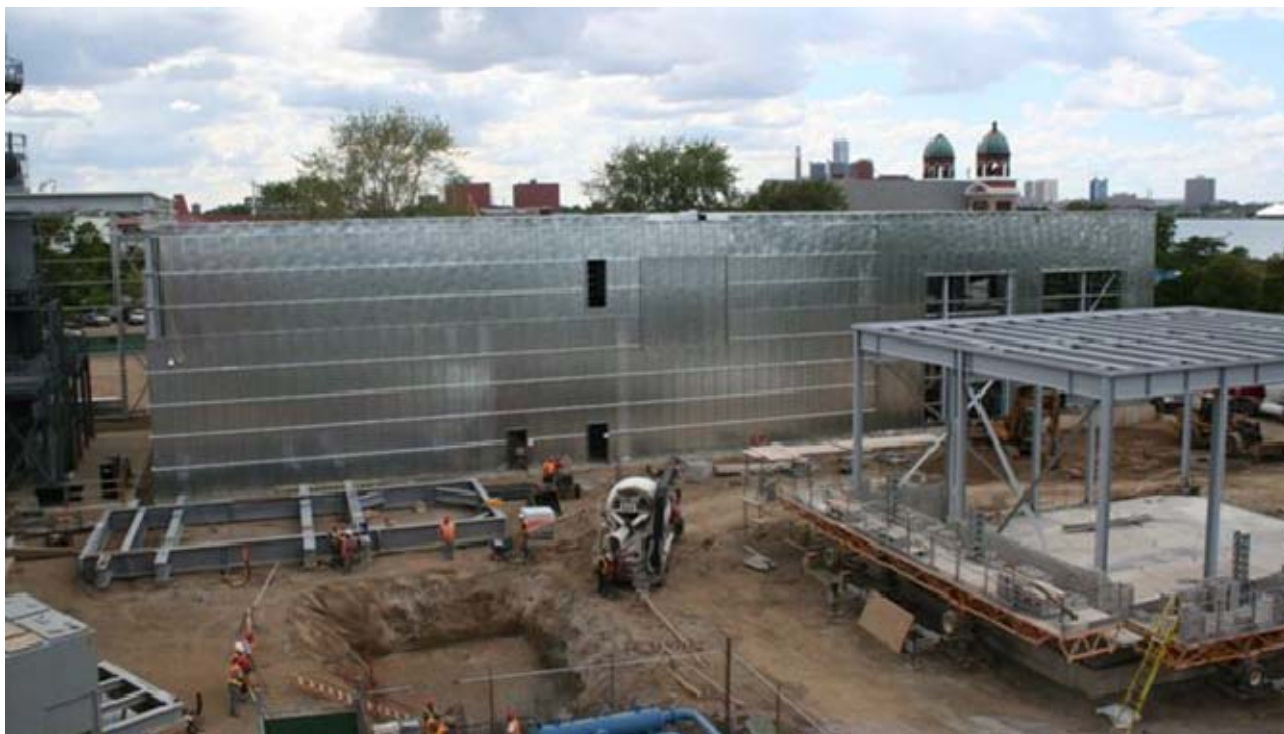
Balance of plant building, cladding erection and installation of the gas compressor building block wall at the East Windsor Cogeneration Centre
