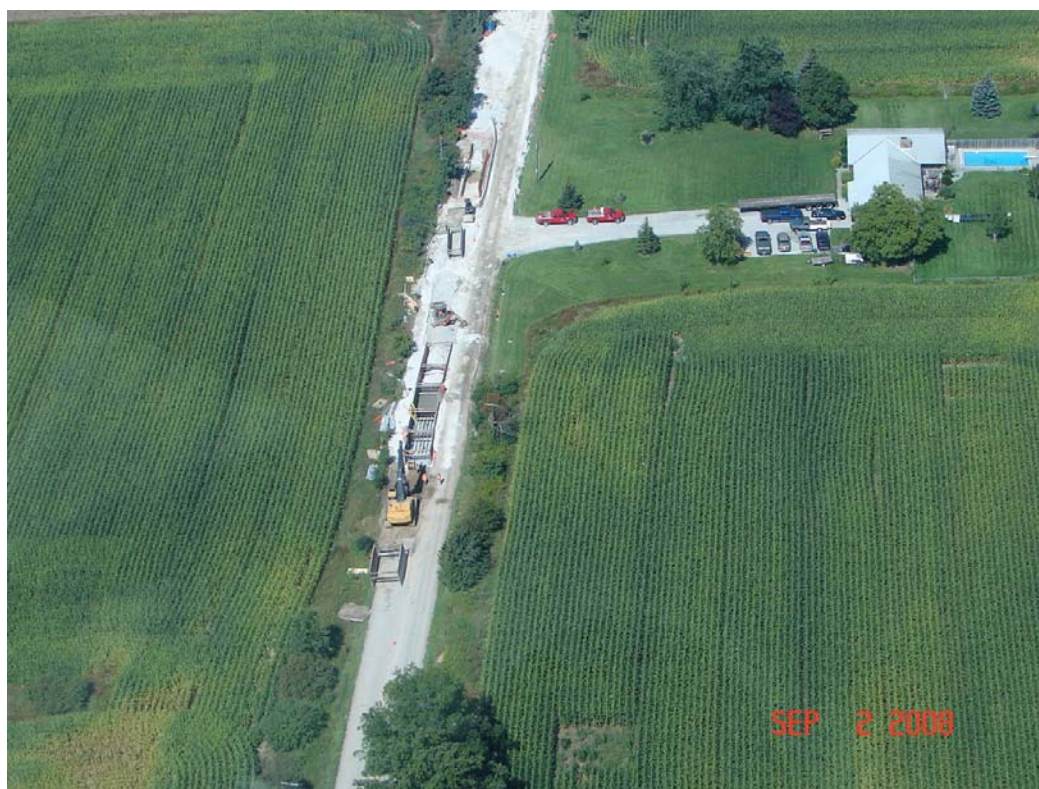
Installation of high-voltage transmission line concrete ductbank in progress at the Halton Hills Generating Station
