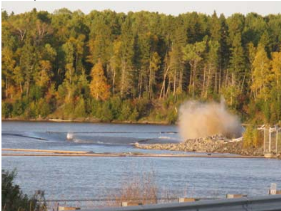
Intake blasting at the Lac Seul Generating Station
