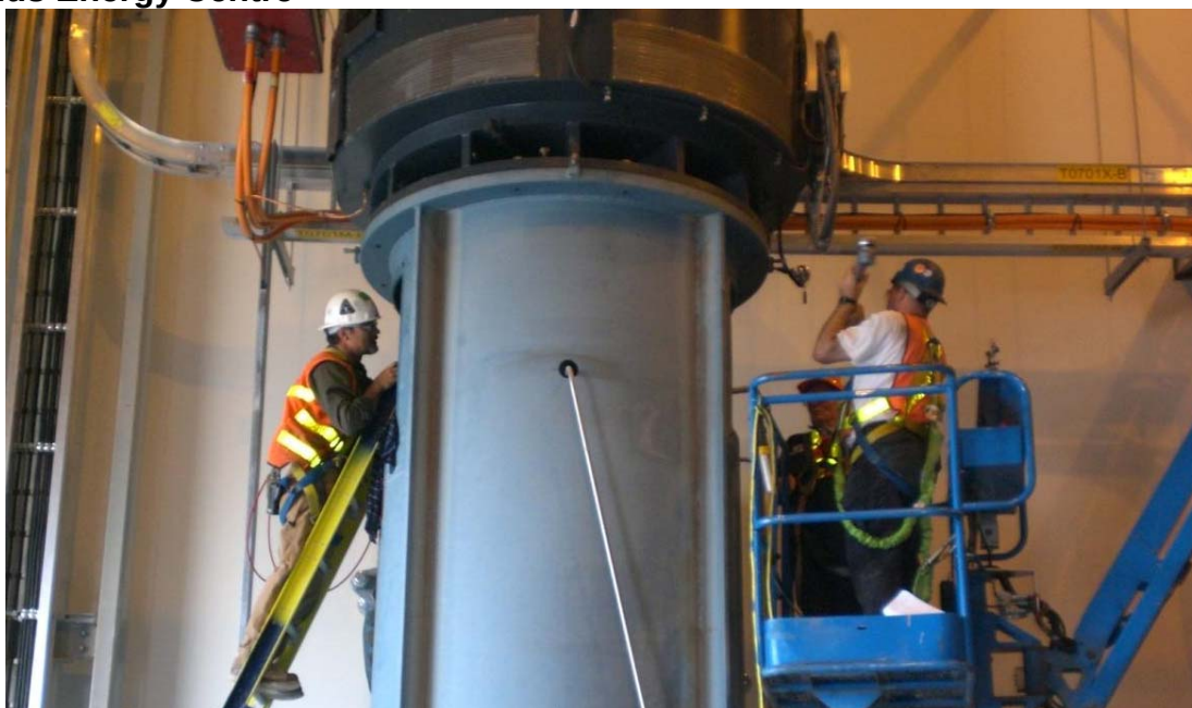
Checking circulating water pumps prior to the initial run at Portlands Energy Centre
