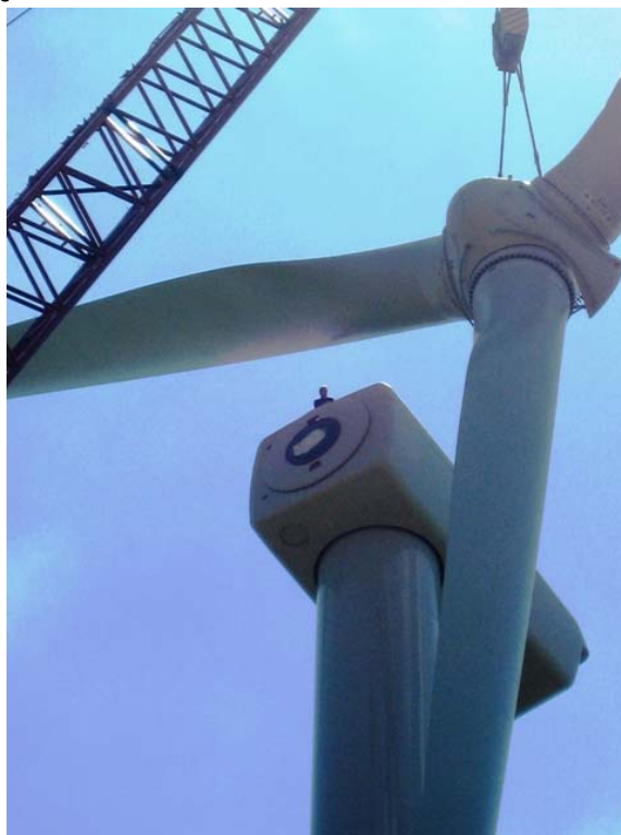
Blade and hub installation in progress at Melancthon II Wind Plant
