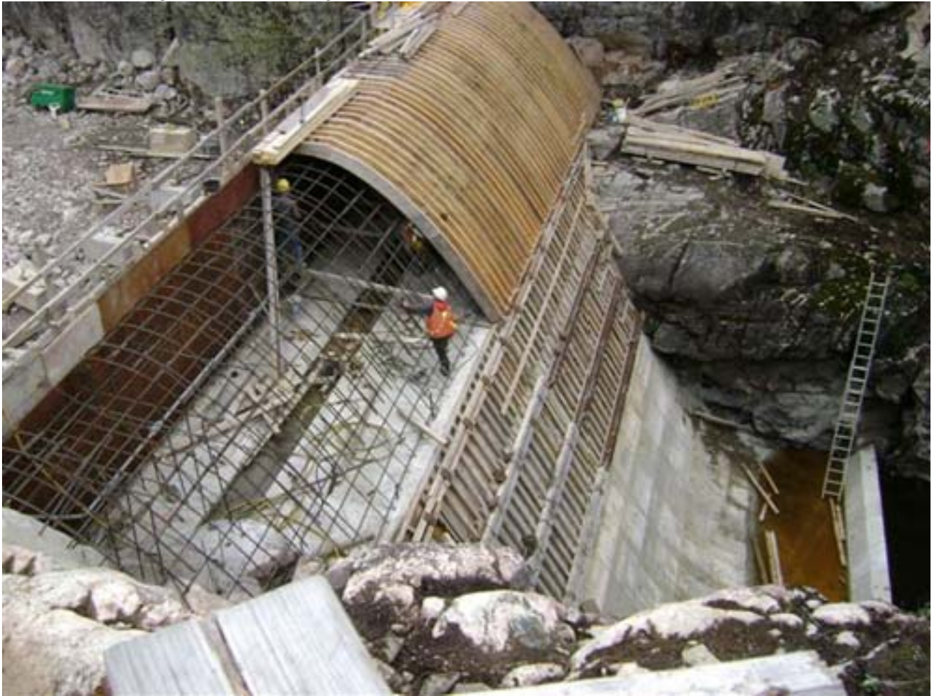
Overflow dam under construction at the Umbata Falls project
