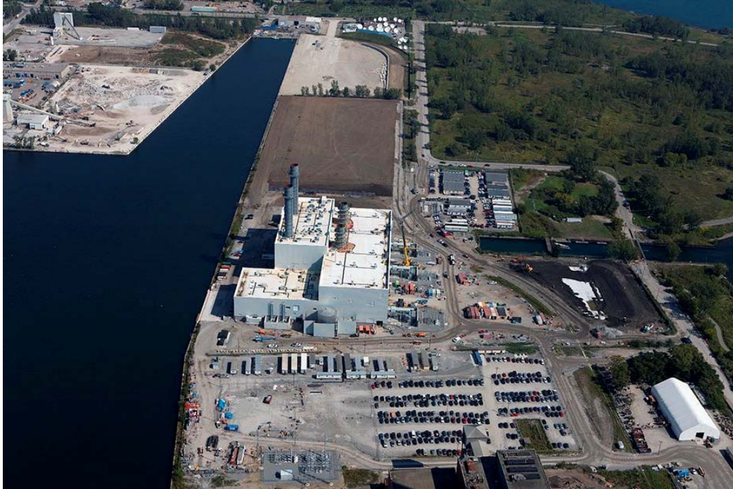
Aerial view of the Portlands Energy Centre from the west
