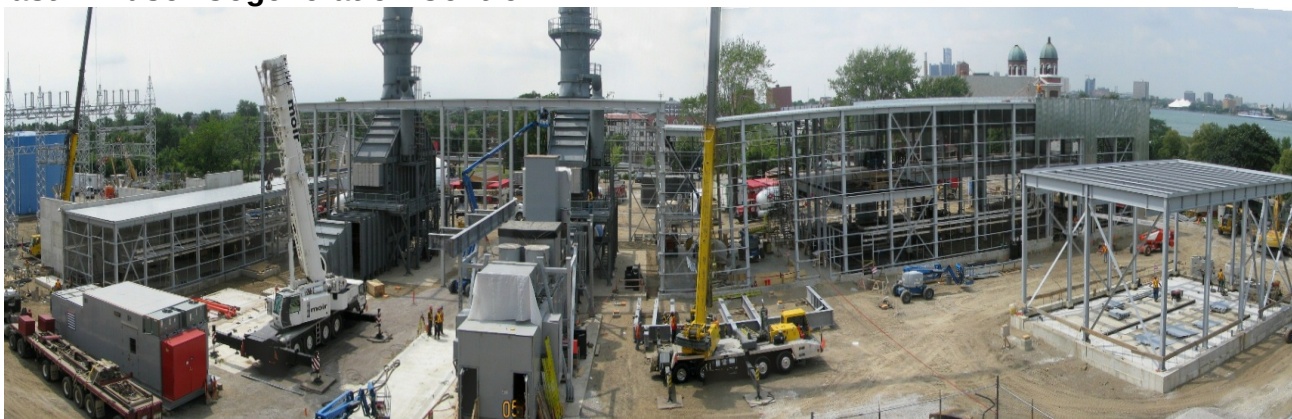
A view of the East Windsor construction site
