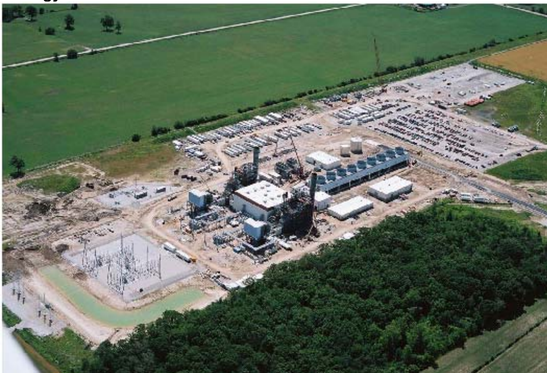
Aerial view of St. Clair Energy Centre
