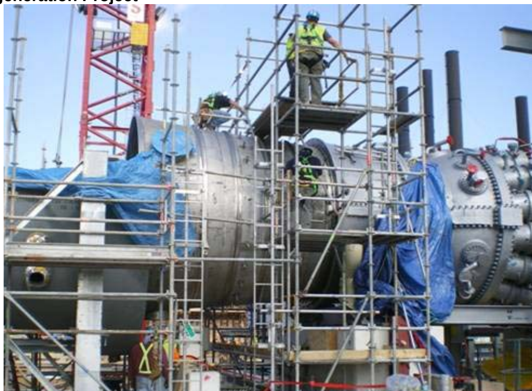
Gas turbine assembly at the Thorold Cogeneration Project
