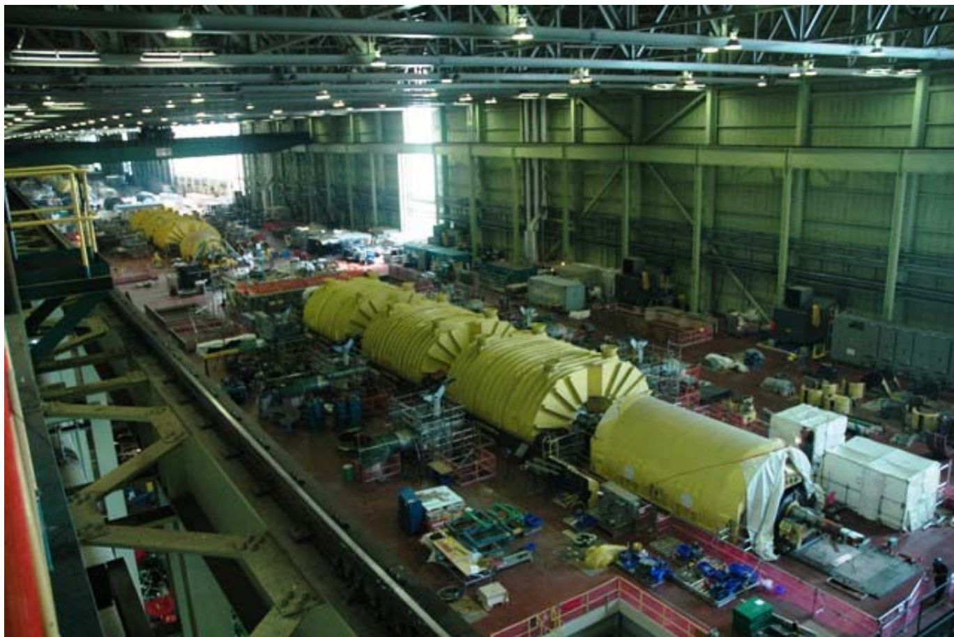
Reassembly of turbine generators for Units 1 and 2 at Bruce A is underway.
