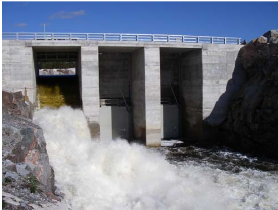
Umbata Falls spillway view from downstream
