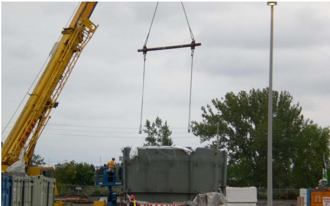
Dismantled stack for simple cycle operation ready to be moved off the Portlands Energy Centre site
