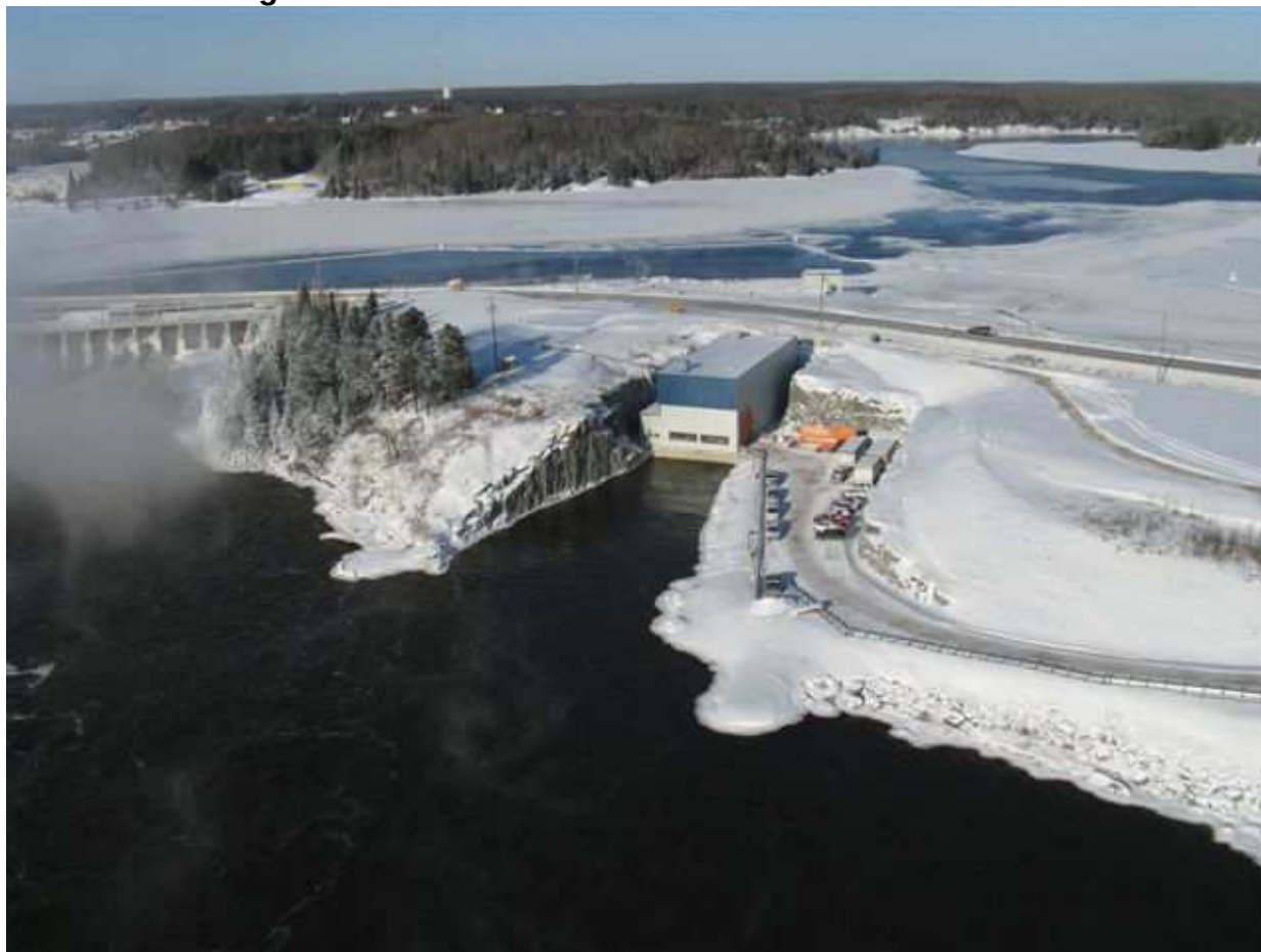
An aerial view of the Lac Seul Generating Station
