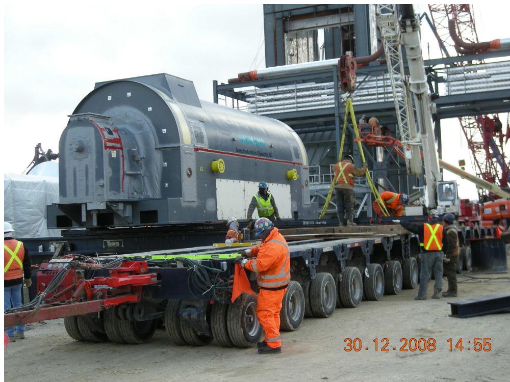
Generator placement in progress at the Halton Hills Generating Station
