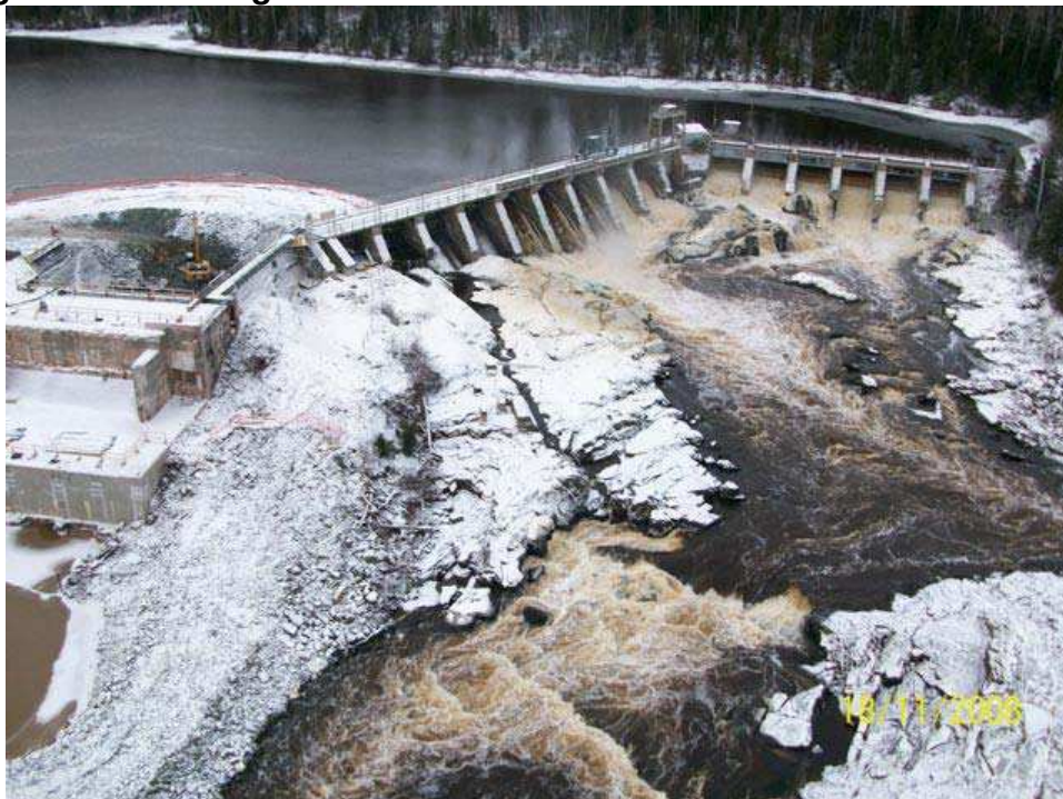
Excavation and spillway at the Lower Sturgeon Generating Station
