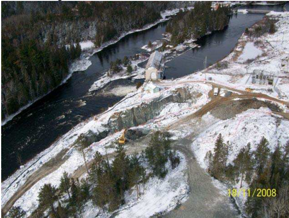
Powerhouse and tailrace excavation at the Hound Chute Generating Station
