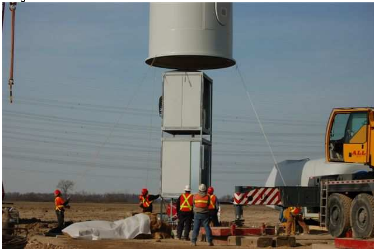
Field assembly of a turbine section at the Enbridge Wind Farm near Kincardine
