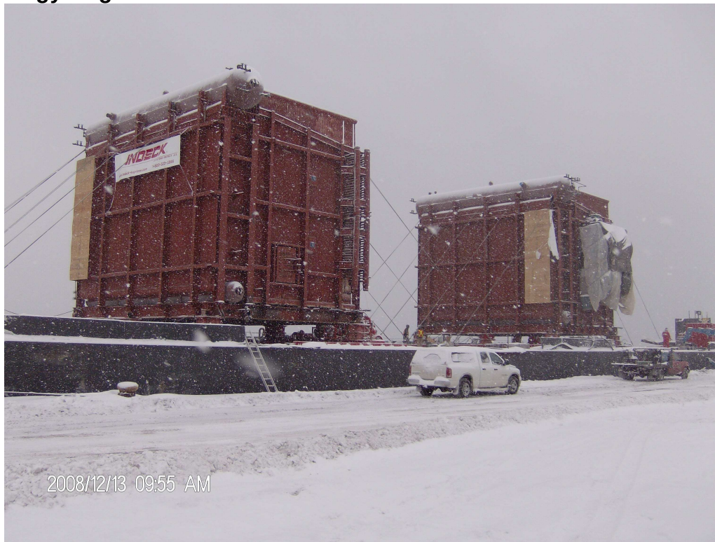
Boiler delivery by barge at the Algoma Energy Cogeneration facility
