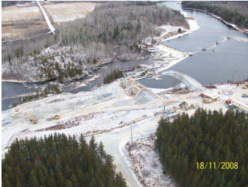
Construction site at the Sandy Falls Generating Station
