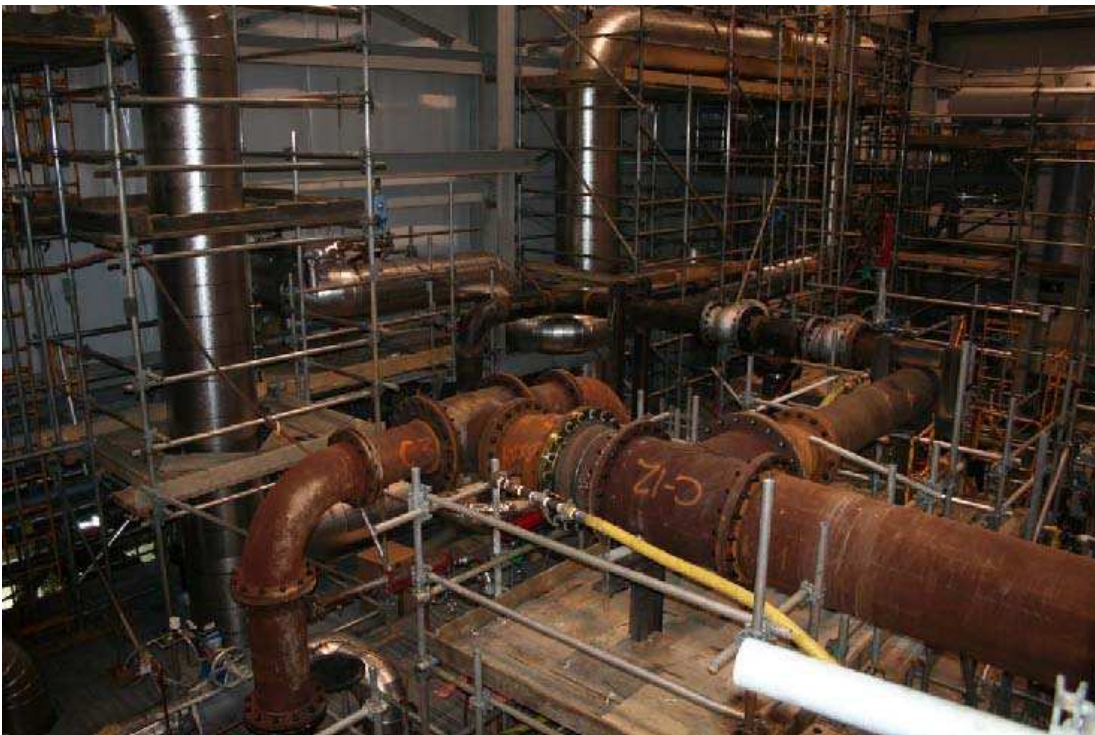
Steam blow piping insulation in progress at the St. Clair Energy Centre
