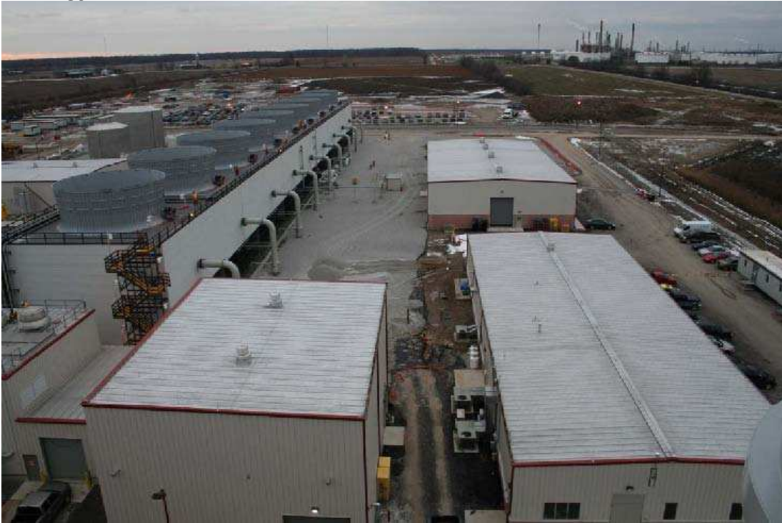
Cooling tower, waste water, administration and warehouse buildings at the St. Clair Energy Centre
