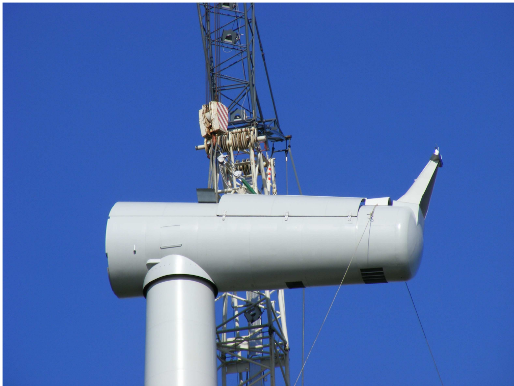
A wind turbine nacelle being erected at the Wolfe Island Wind Project
