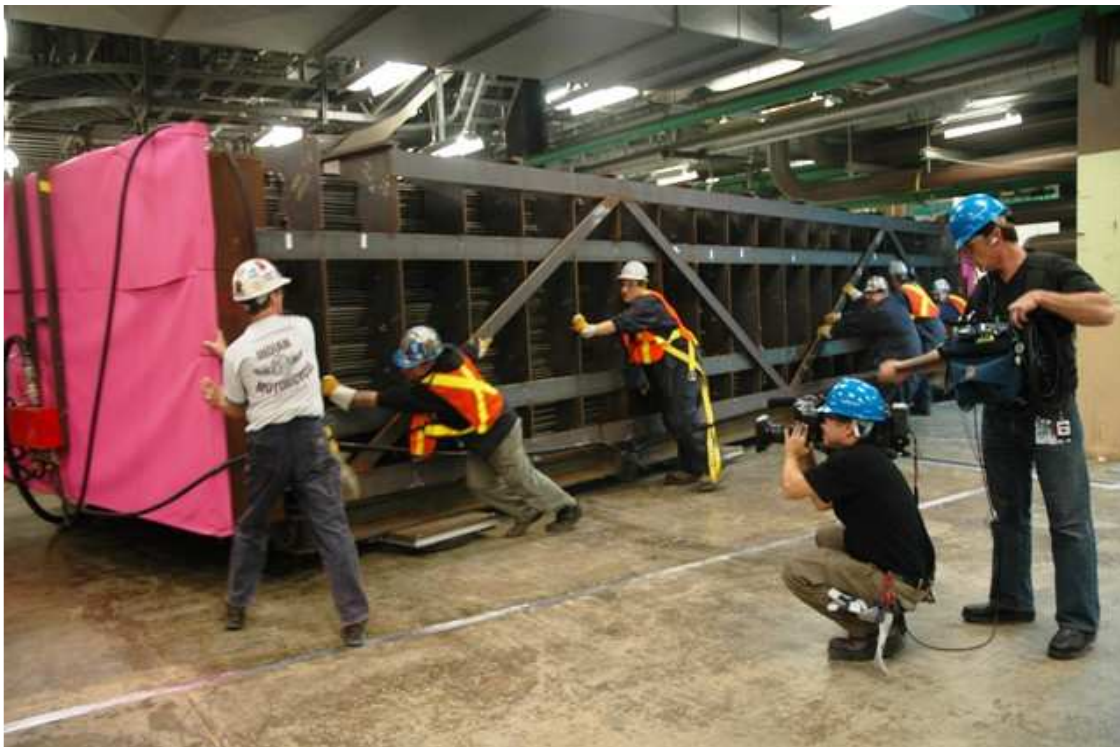
Moving last of 12 new tube bundles into staging position for installation at Bruce A Unit 2
