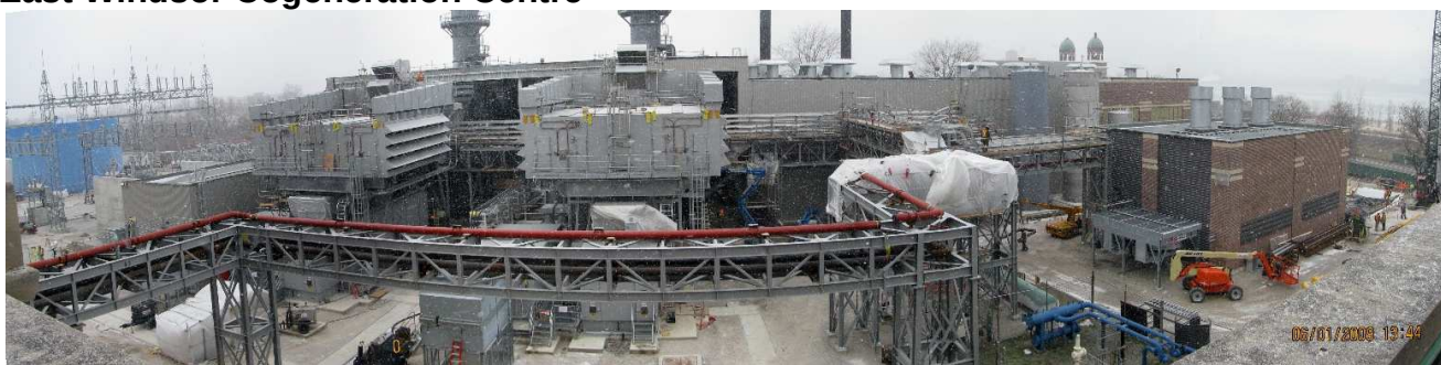
A panoramic view of the East Windsor Cogeneration Centre construction site
