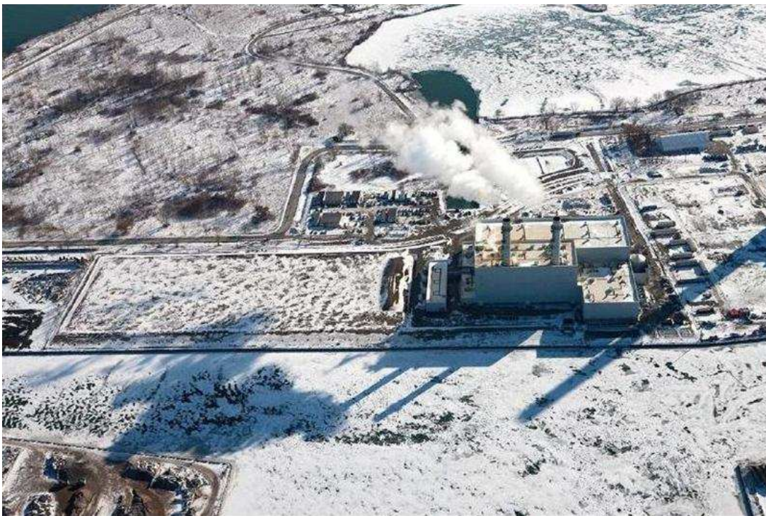
Aerial view of the Portlands Energy Centre from the north
