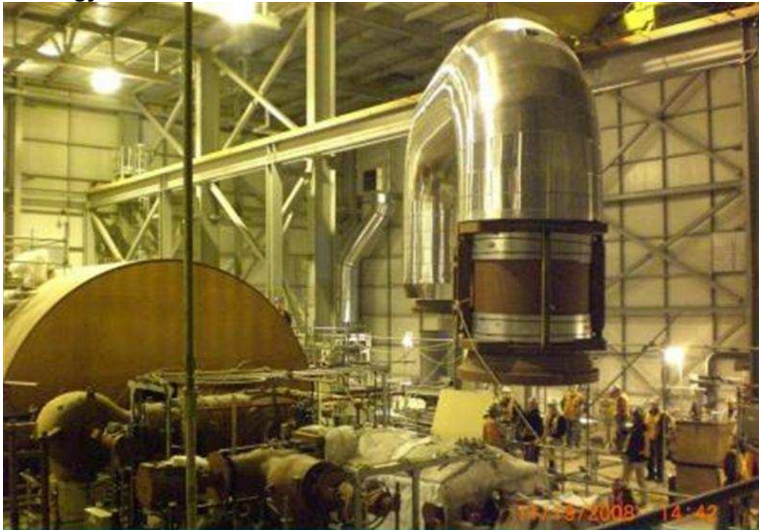
Lifting the crossover pipe to be installed at the steam turbine at the Portlands Energy Centre
