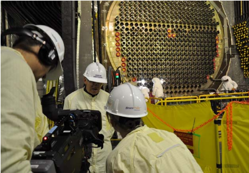
Bruce A Units 1 and 2 Restart Bruce Power President and CEO, Duncan Hawthorne, being interviewed for the Discovery Channel in front of the Unit 2 reactor
