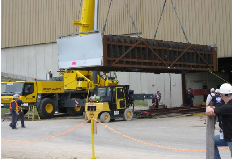
Bruce A Units 1 and 2 Restart Delivery of final condenser tube bundle being moved with a 275-ton, heavy-duty mega form boom, hydraulic crane
