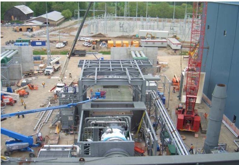
Halton Hills Generating Station Installation of combustion turbine #2 underway
