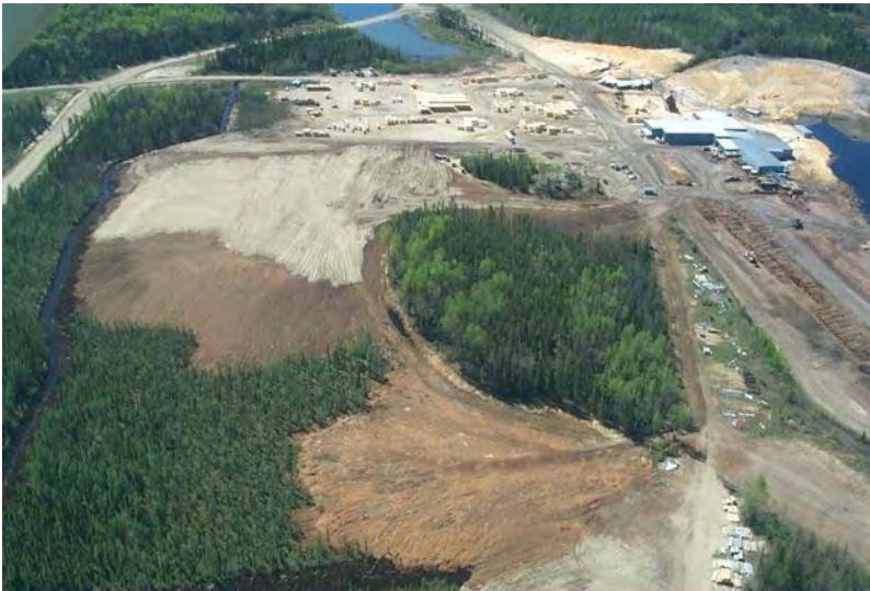
Becker Cogeneration Plant Aerial view of the site for the new plant to be located in the northern region of the District of Algoma
