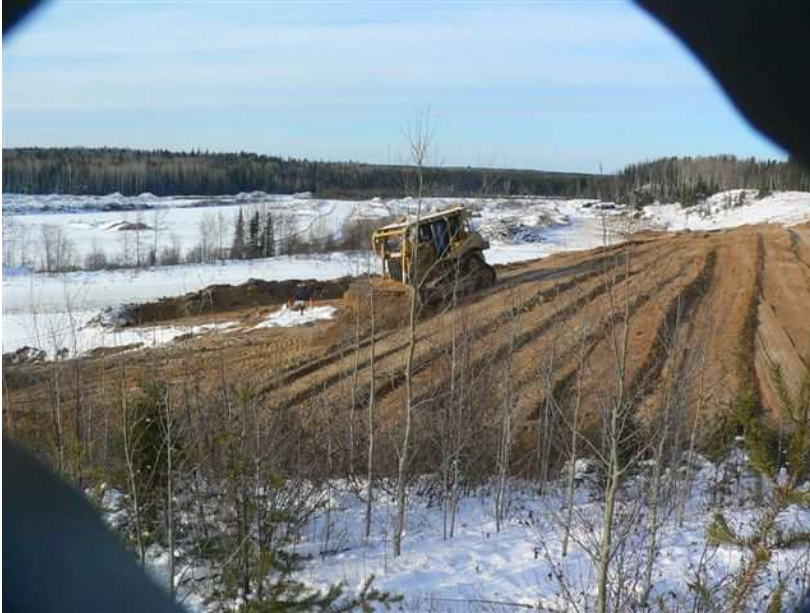
Becker Cogeneration Plant Site clearing and preparation for construction in progress and near completion
