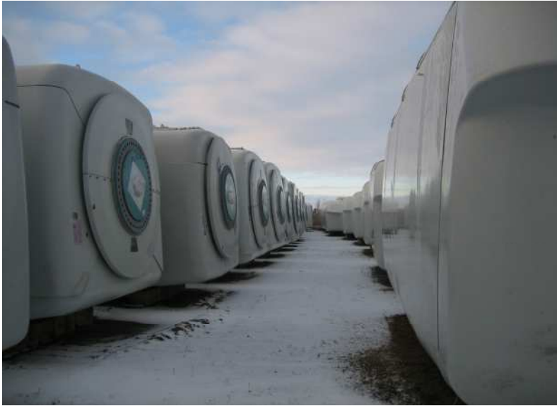
Raleigh Wind Energy Centre Nacelle components have been delivered to the site and are ready for installation
