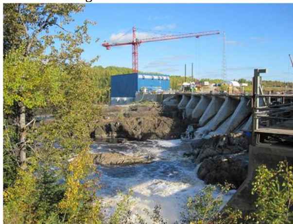
Figure 16 – Construction around the Lower Sturgeon GS powerhouse. Dam rehabilitation and all headgates were installed and commissioned. All rock was blasted and excavated from the upstream rock plug, while cofferdam removal is in progress. The project is 95 percent complete. Commissioning activities continue. Backfeed with Hydro One grid was completed.
