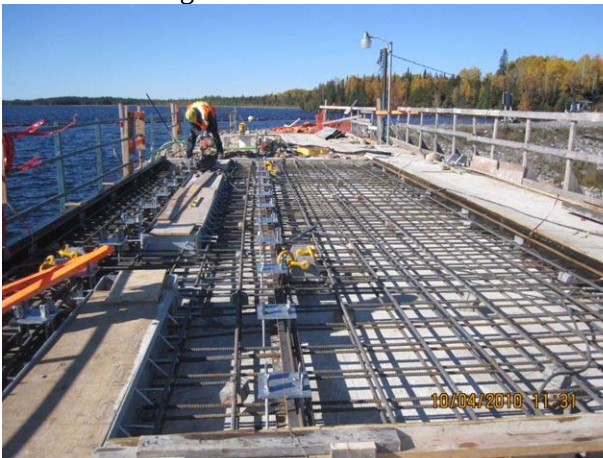
Figure 18 – Dam rehabilitation work continues. As of the end of the third quarter, the project is 97 percent complete. All water-to-wire electrical and mechanical construction activities were completed. Water-to-wire dry testing was completed. Wet commissioning activities continue. Downstream cofferdam was removed and tailrace was watered up. Watering up of both penstocks was completed.
