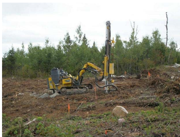
Figure 4 – Drilling for transmission line poles. Transmission line-related work commenced and installation of collector circuit poles was progressing.
