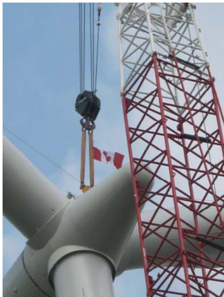
Figure 1 – During the third quarter 2010, remaining work on site involved: restoration of private property and public roadways; construction of the permanent operation and maintenance (O&M) building to house service and maintenance crews; and final documentation, cleanup, and contractor demobilization.
