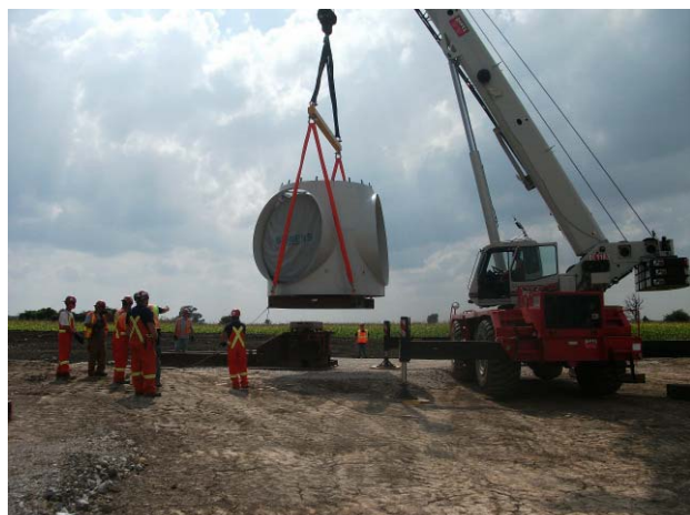
Figure 9 – As of the end of the third quarter, access roads were 100 percent complete. Foundation work for turbine towers continued and turbine erection commenced.
