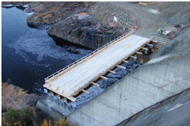
Figure 11 – A temporary bridge built across the Harmon spillway. Road access commenced at Harmon GS.
