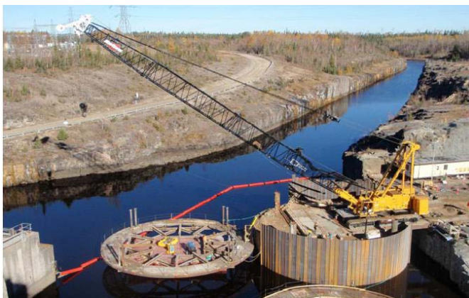
Figure 13 – Cell one (of two) for the Little Long GS cofferdam was installed.
