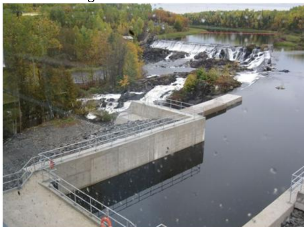
Figure 17 – Intake and an upstream view from the powerhouse. The project is 92.5 percent complete including dam rehabilitation work. First synchronization achieved on August 30. Site restoration was completed. Commissioning activities in progress.
