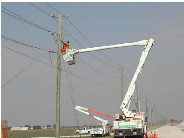
Figure 5 – Lineman connecting a collector line. IESO meter registration process was complete and an authorization to interconnect was received from IESO on September 2.
