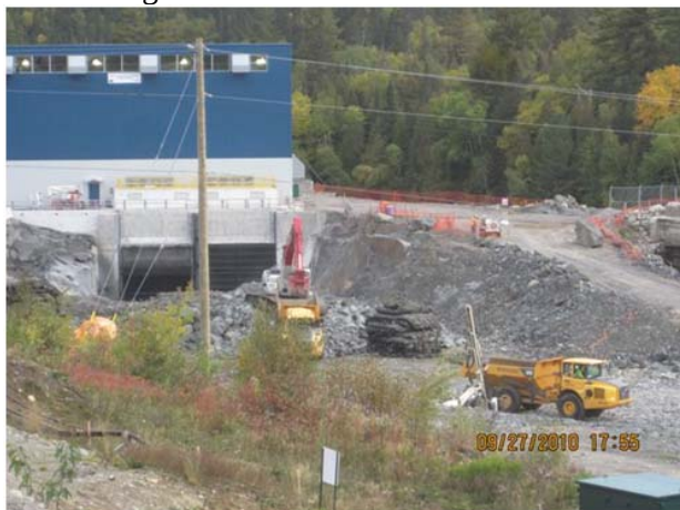
Figure 15 – Work around the Hound Chute powerhouse. The project is 93 percent complete with all mechanical and electrical installations inside the powerhouse completed. Commissioning activities are in progress. Backfeed with Hydro One grid was completed.
