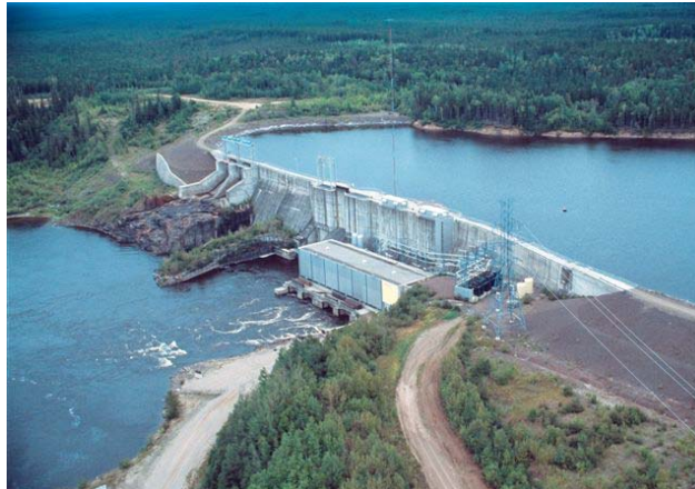
Figure 12 – A view of Kipling GS. The station is in the planning stage.
