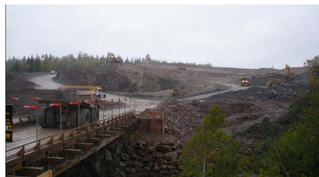
Figure 14 – The bridge and access to Smoky Falls island was completed. Excavation for the new Smoky Falls powerhouse commenced.
