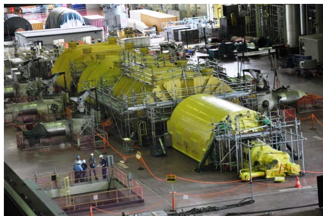
Figure 23 – Workers giving the turbine generator in unit 2 a new paint job while commissioning progresses.
