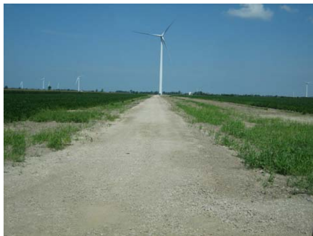
Figure 8 – During the third quarter, all tower erections were completed.
