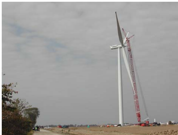
Figure 6 – A rotor being installed. Three turbines are generating power as of September 30.
