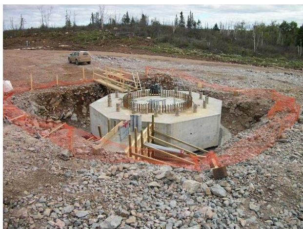
Figure 3 – Turbine foundation work in progress. As of the end of the third quarter 2010, IESO market entry was progressing. Access road and turbine foundation work continues.
