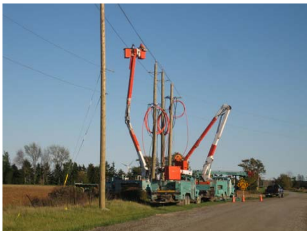
Figure 7 – Workers installing collector system. As of the end of the third quarter, the underground collection system was 10 percent complete and the electrical overhead collection system was 100 percent complete.
