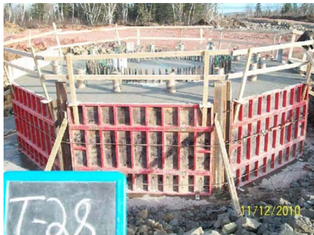
Figure 9 – At the end of the quarter, 85 percent of all turbine foundation work was completed.
