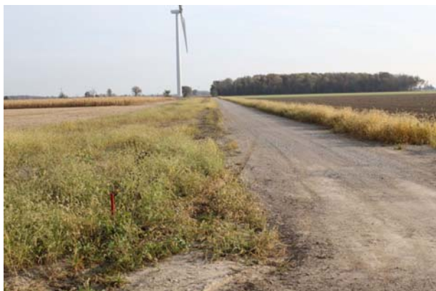
Figure 13 – Collector system and access roads are complete.
