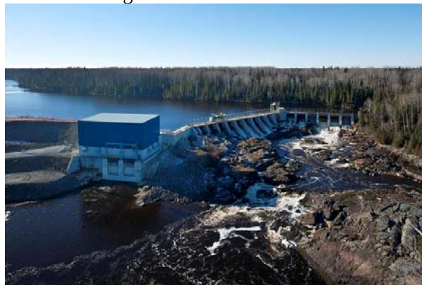
Figure 6 – A view of the new powerhouse and the refurbished dam structure.
