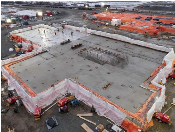
Figure 17 – Permits for equipment foundations, entrance roadway, construction trailers/equipment laydown and temporary bridge at site entrance have been issued. Major foundations for power block equipment including turbines and generators have been poured.
