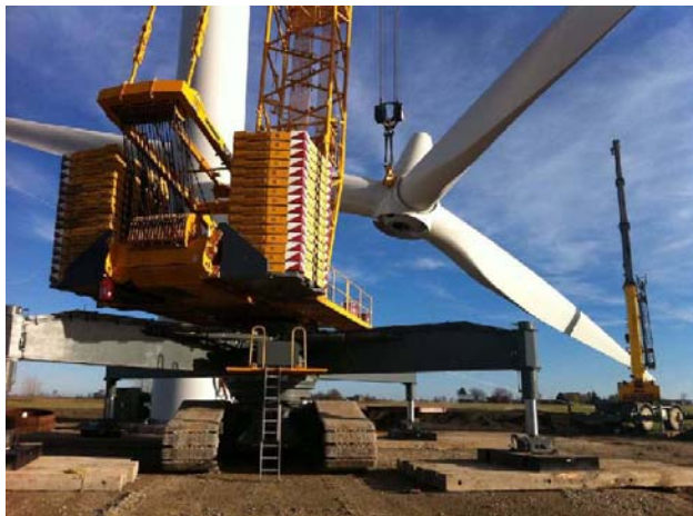
Figure 15 – Lifting of the last turbine rotor in progress. All of the turbines were commissioned.
