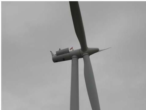
Figure 11 – Last tower erected in November. Received New Facility Notification Form confirming that Market Entry process was completed.
