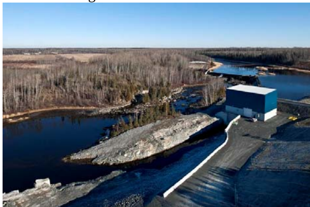
Figure 7 – A view of the new powerhouse and the tailrace.
