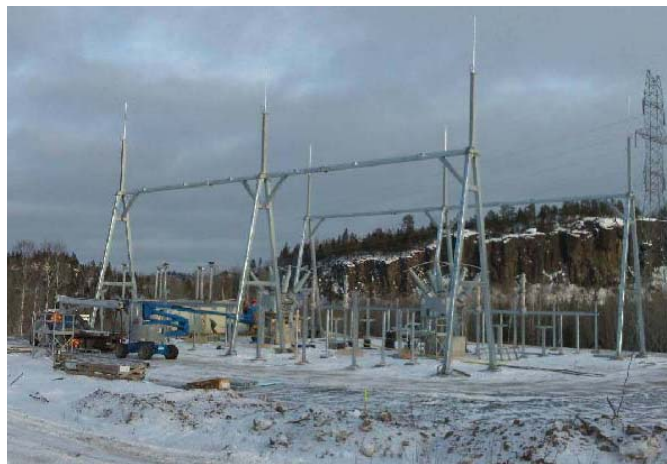
Figure 10 – Transmission lines related work has commenced. Substation transformers are in place and ready to be energized. Switching station is ready to be tested.
