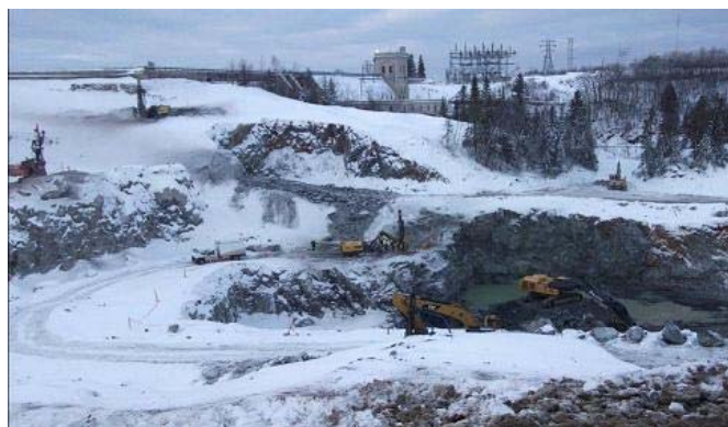
Figure 4 – Excavation continues on exposed bedrock within the powerhouse/tailrace and intake channel footprints. The upstream cofferdam rock fill work was completed and installation of the cofferdam cut-off wall has commenced.
