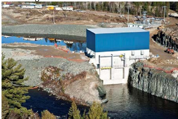
Figure 5 – A view from the tailrace of the new powerhouse.
