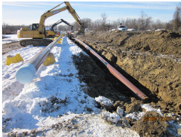
Figure 18 – Enbridge pipe installation of 300 meters of gas pipeline on site to the valve station has been completed. Significant construction progress was made on the entrance roadway, stormwater pond, underground utilities and construction trailer/equipment laydown area. Major equipment fabrication for turbines, generators and transformers was completed, and deliveries are underway well ahead of schedule.
