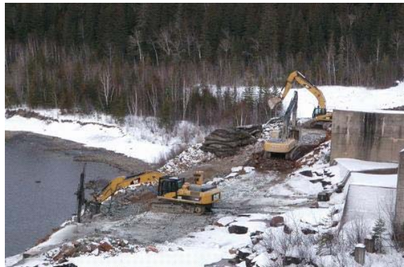
Figure 2 – Spillway access was completed. Drill and blast operations and hauling to the marine pad is ongoing.
