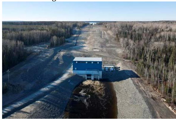
Figure 8 – Looking upstream from the tailrace of the new Wawaitin GS.
