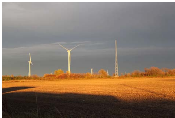
Figure 14 – 51 of 52 turbines have been commissioned.
