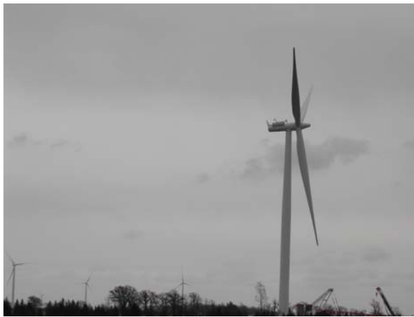
Figure 12 – All turbines were commissioned by November 19 and all commissioning tests completed with Hydro One and IESO.
