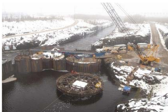
Figure 3 – The cellular cofferdam is near completion with work continuing on the east side shore tie-in.
